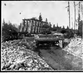
Head gate on Ward Ditch.
