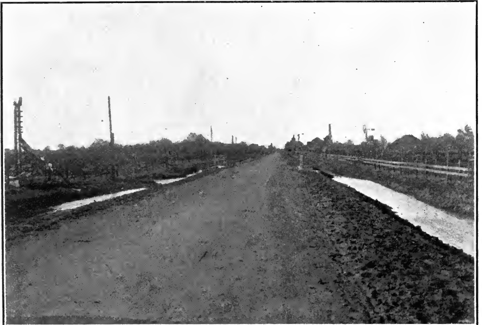
MARIPOSA ROAD AFTER IMPROVEMENT. THIS ROADWAY REMAINED PRACTICALLY UNINJURED AFTER THE FLOODS OF THE PAST WINTER.
