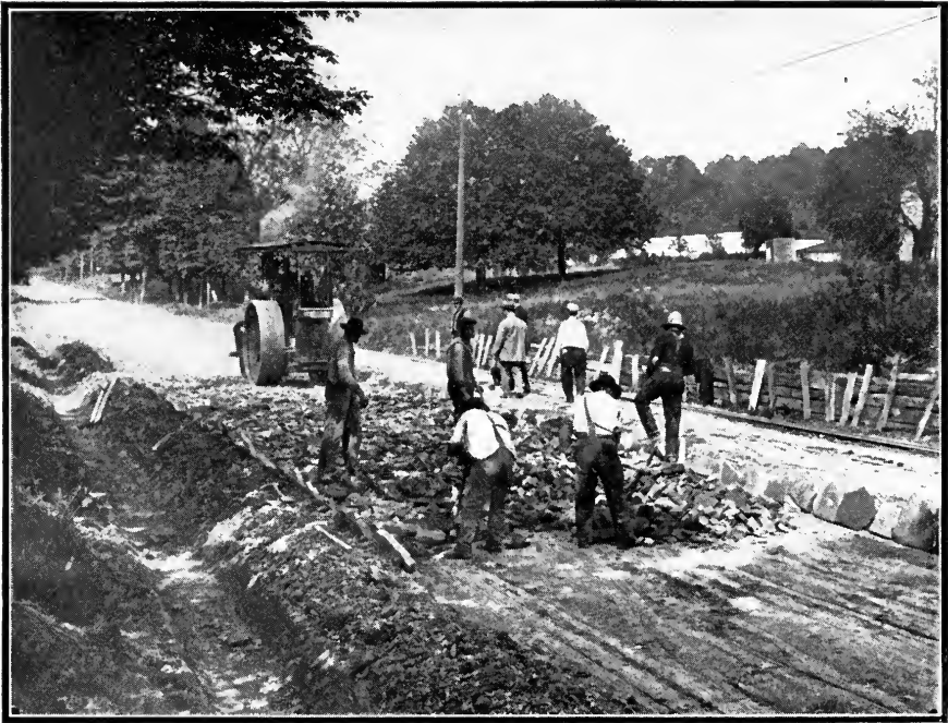
CLEVELAND TO PAYNESVILLE ROAD, BUILT BY THE AUTOMOBILE CLUB. SHOWING THE THOROUGH MANNER IN WHICH THE ROAD WAS LAID.
