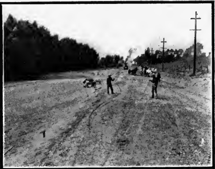
SURFACING THE BOULEVARD.
