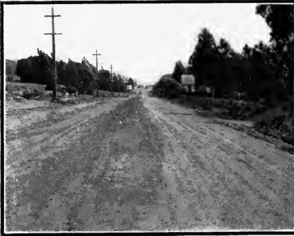
THE FINISHED ROADWAY.
