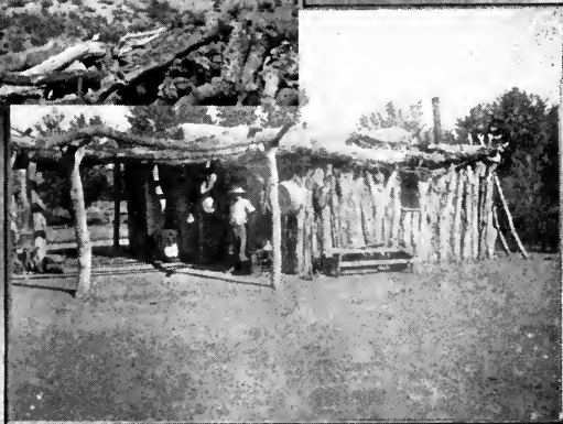
From top to bottom—1. A home constructed of adobe and brush. 2. Adobe bricks being made on a home-made press in the desert. 3. Typical mud roof home. 4. The jacal, the uprights of cottonwood cuts, chinked with mud.
