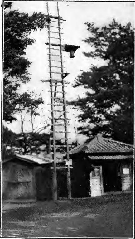
A Japanese "fire tower" and bell, used to sight distant fires and sound an alarm.
