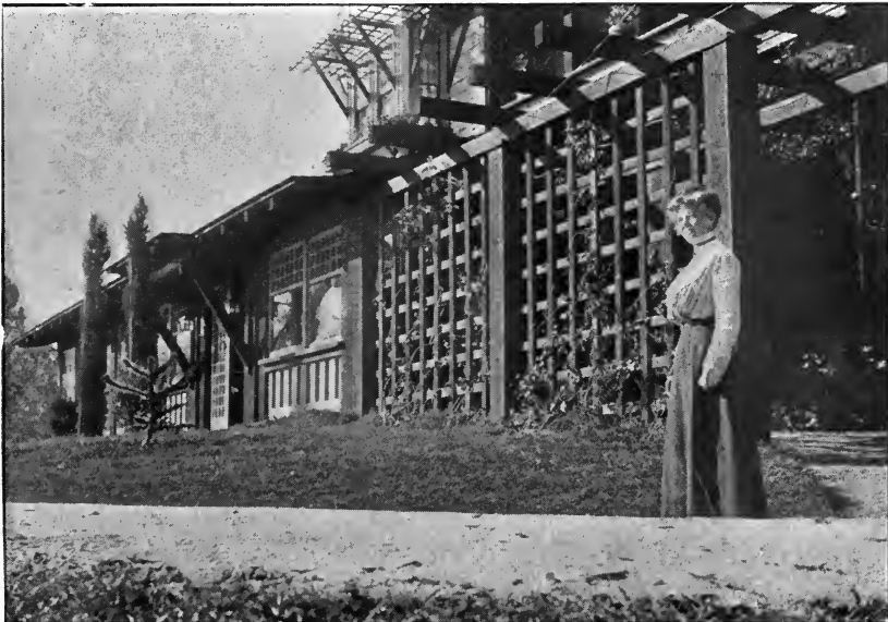
"The entrance hall which has been added."
