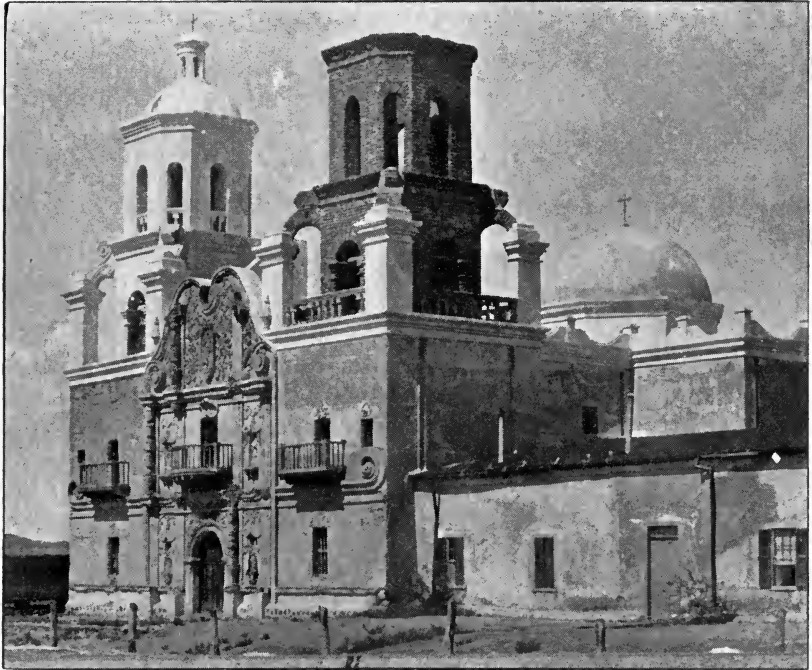
San Xavier del Bac. (Notice the adobe construction of the unrestored tower.)
