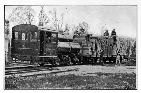
Compressed air engine and a truck car of loaded ammunition on a mile run to the water front on the Hudson River, New York.
