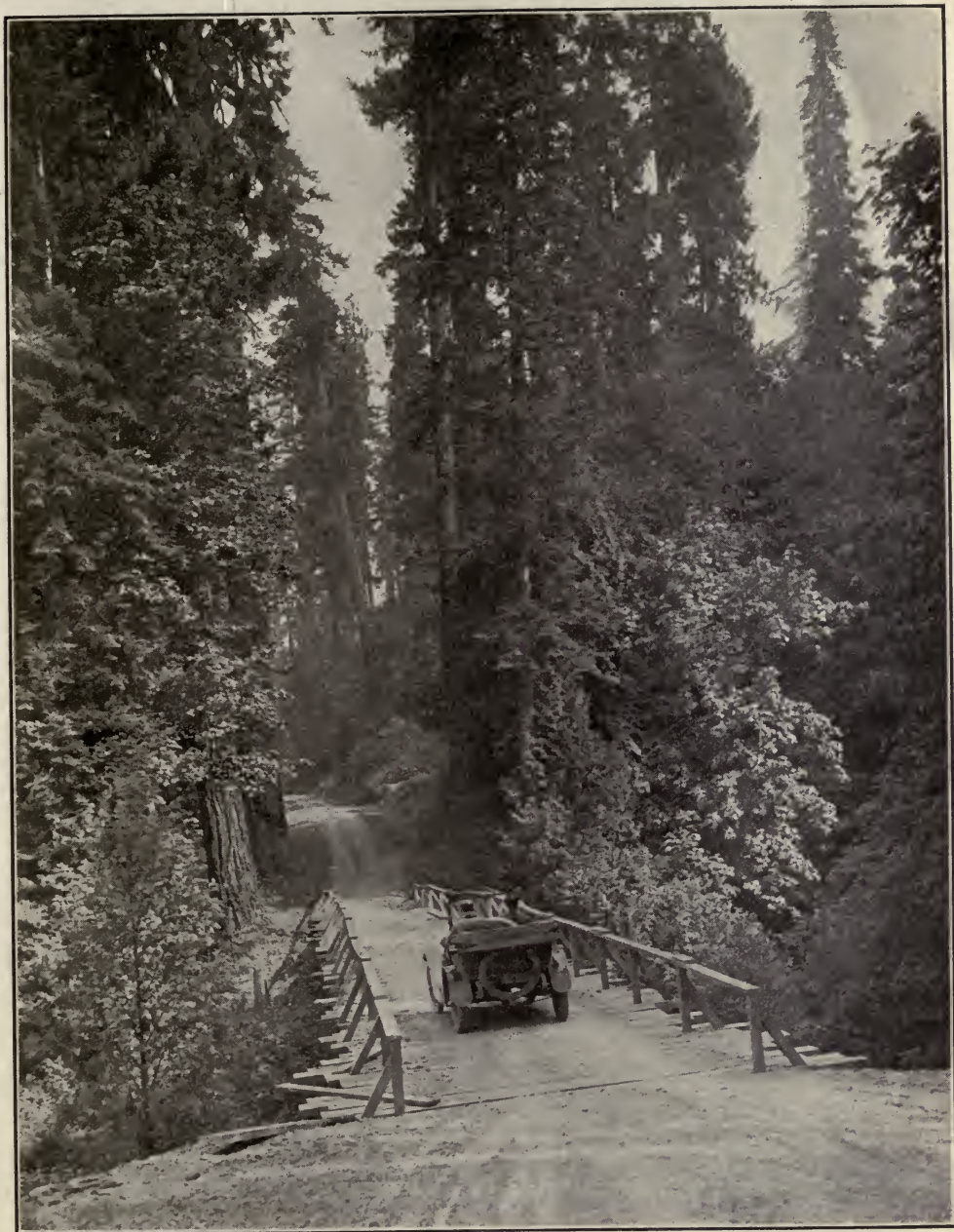
On the Pacific Highway, in a stretch of pine forest.
