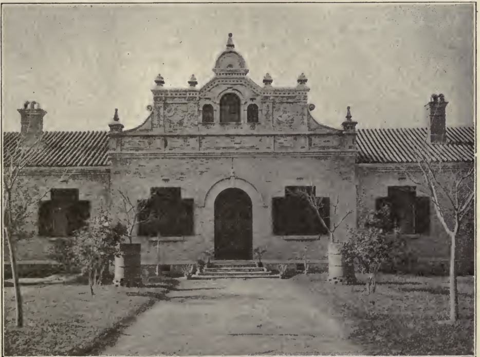
Middle School building.
