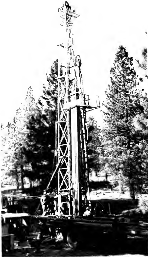
Rotary Well-drilling Rig in Operation
