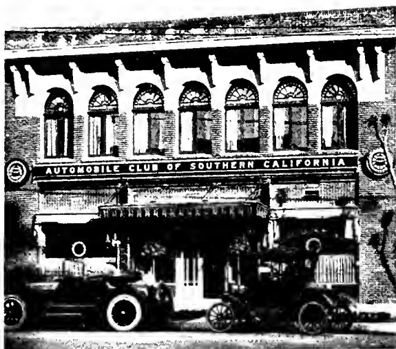
CLUB HEADQUARTERS, 1344 SO. FIGUEROA STREET
