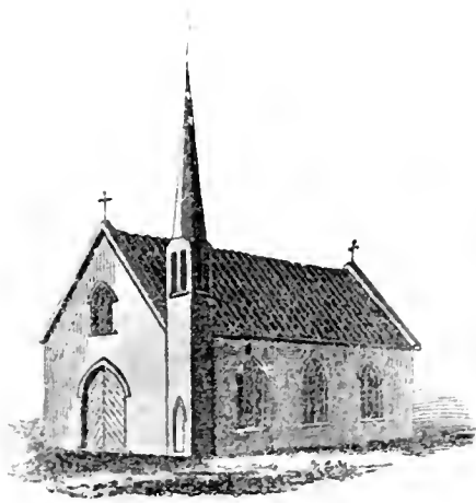
GRACE CHAPEL (1849) SOUTHWEST CORNER POWELL AND JOHN STS., SAN FRANCISCO
