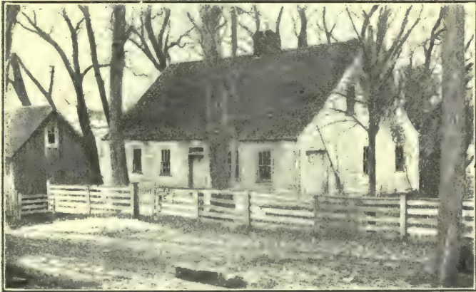
GLEN ALLAN—Oldest house in Bridgewater, N.S.
