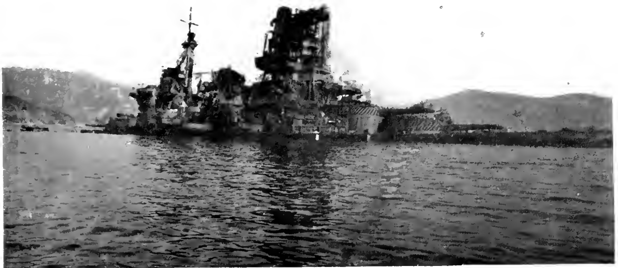
Photo 6 Beam View of Haruna (BB)
