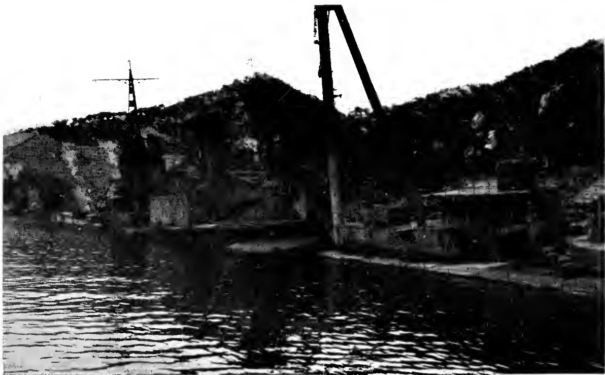
Photo 24 Appendix 107 Port Quarter View of Superstructure of Settsu (CL)
