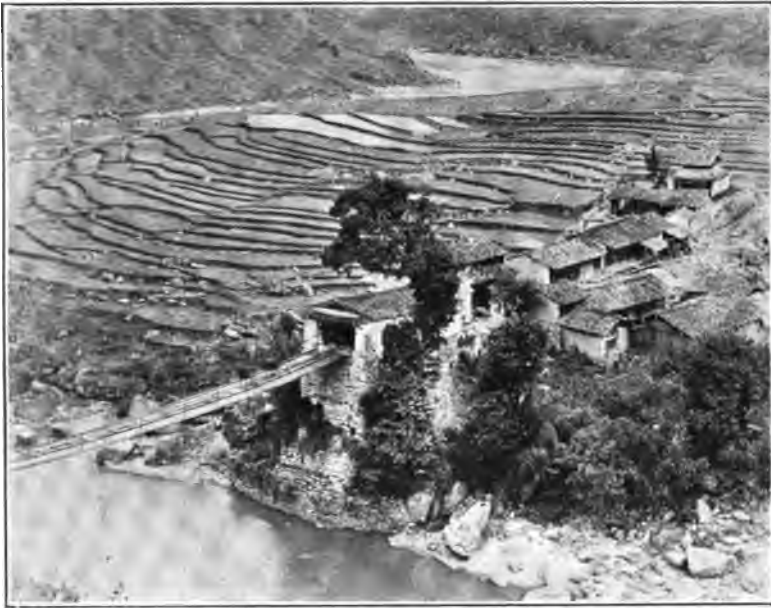
A SUSPENSION BRIDGE
