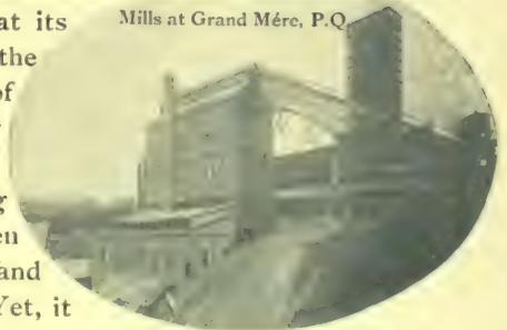
Acid Tower and Pulp Mill
