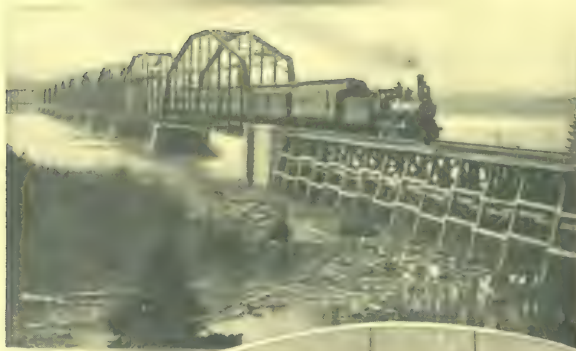
International Bridge at Soo
