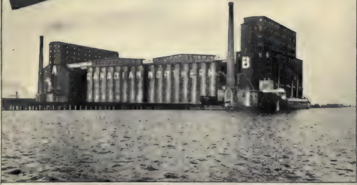
CANADIAN NORTHERN ELEVATOR AT PORT ARTHUR.
