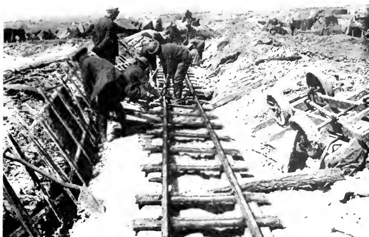
BUILDING A LIGHT RAILWAY OVER VIMY RIDGE
