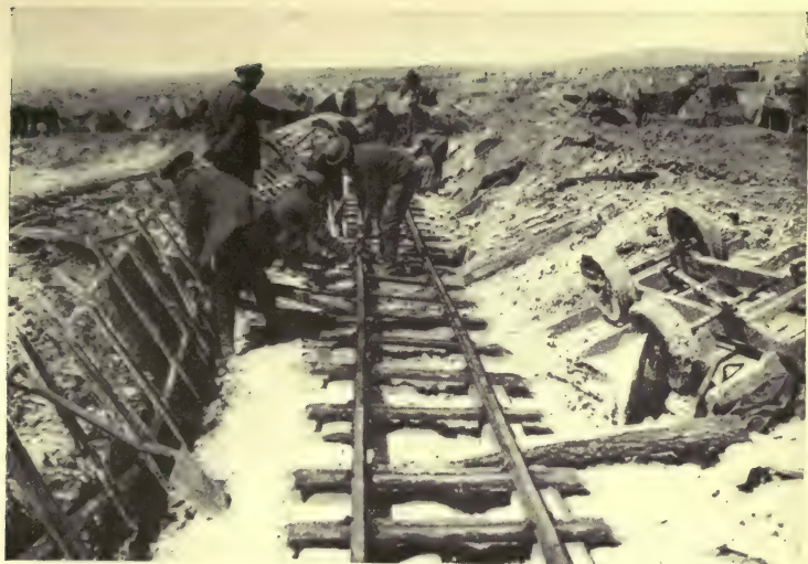
BUILDING A LIGHT RAILWAY OVER VIMY RIDGE
