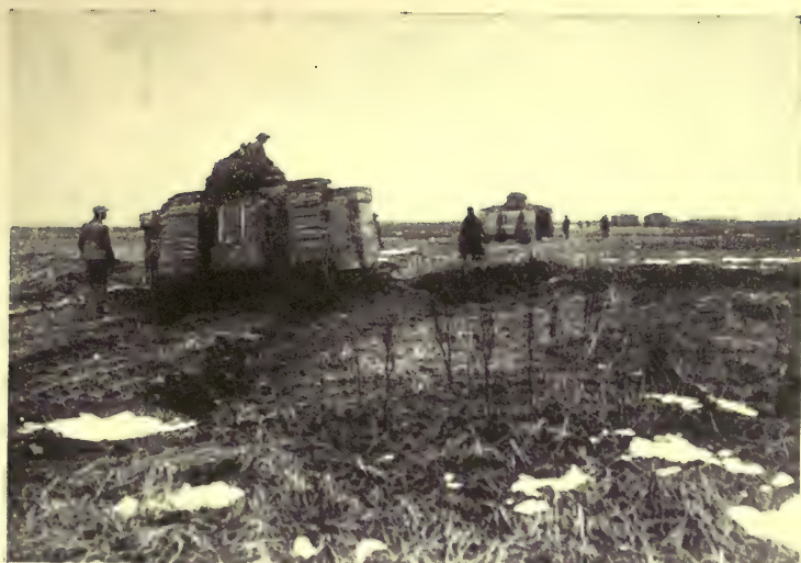
TANKS IN ACTION
