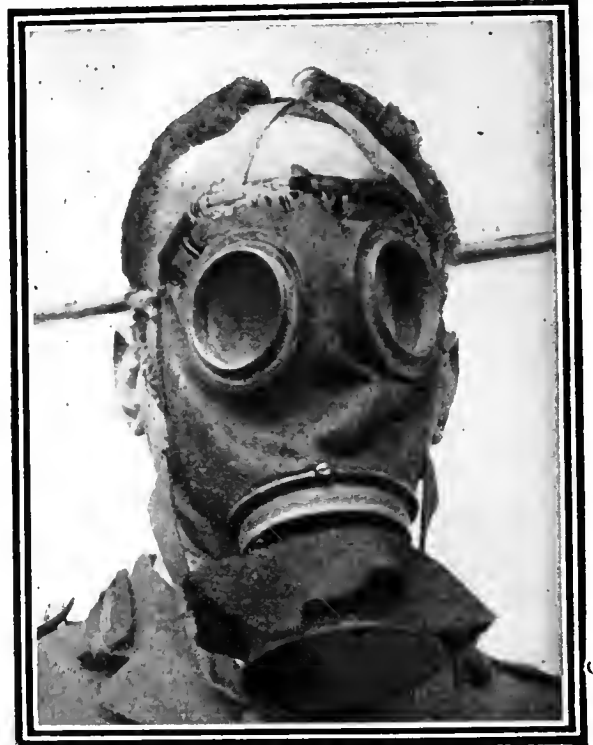
These gas masks, taken from the Germans by Canadians, show that, owing to shortage of rubber, the flexible parts are now made of leather
