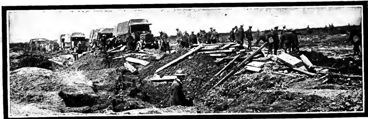
When the Canadians cannot wait for light railways they build cordwood roads. This is the improvised road on which they followed up victory across Vimy Ridge
