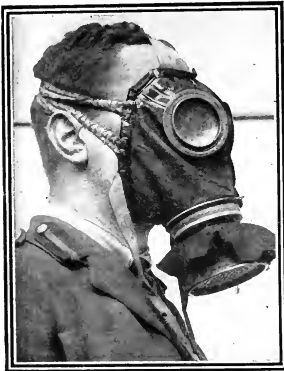
These gas masks, taken from the Germans by Canadians, show that, owing to shortage of rubber, the flexible parts are now made of leather
