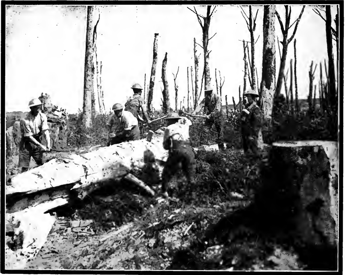
Splitting trunks of trees into logs for reinforcing trenches
