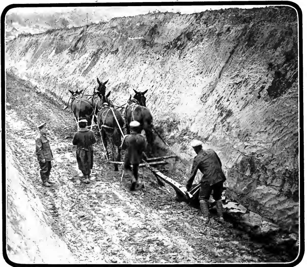
Light Railway construction troops ploughing up the earth which the drag "scrapers," drawn by mules, carry away for "dumping"
