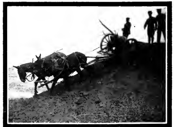
"Scraper" dumping its haul
