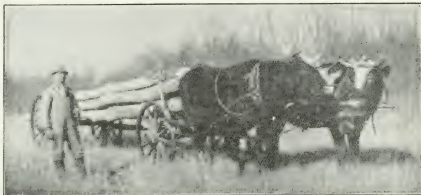
HOW THOSE MEN WORKED, CUTTING DOWN TIMBER, GRUBBING OUT STUMPS, AND BUILDING LOG SHACKS
