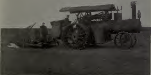
1. Threshing outfit off to the wheatfields. 2. Breaking up new wheat lands. 3. The steam plough.
