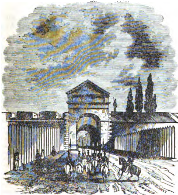
ST. LOUIS GATE, DEMOLISHED, AUGUST, 1871.
