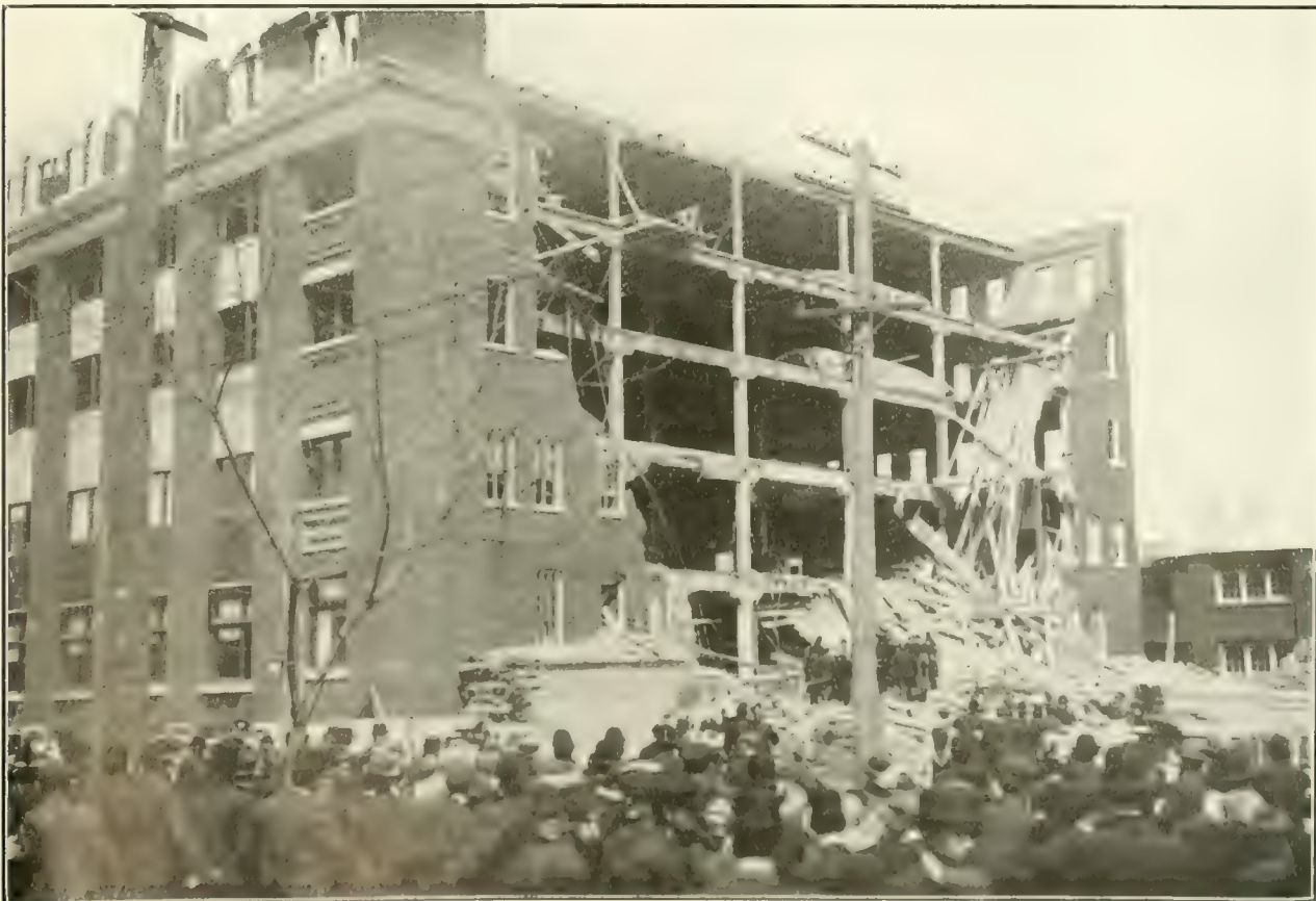
South wall of Neilson factory, Gladstone Avenue, Toronto, which collapsed at 10:30 a.m. on Saturday, May 4th, 1912
