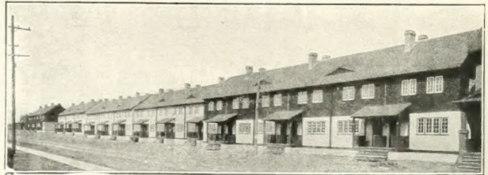
Workmen's Houses, erected by the Brown Brass & Copper Co., New Toronto; using only Stucco Board inside and outside on studding; plastered on interior and stuccoed, shingled and clagboarded on Stucco Board on exterior, giving cozy, homelike effect.
