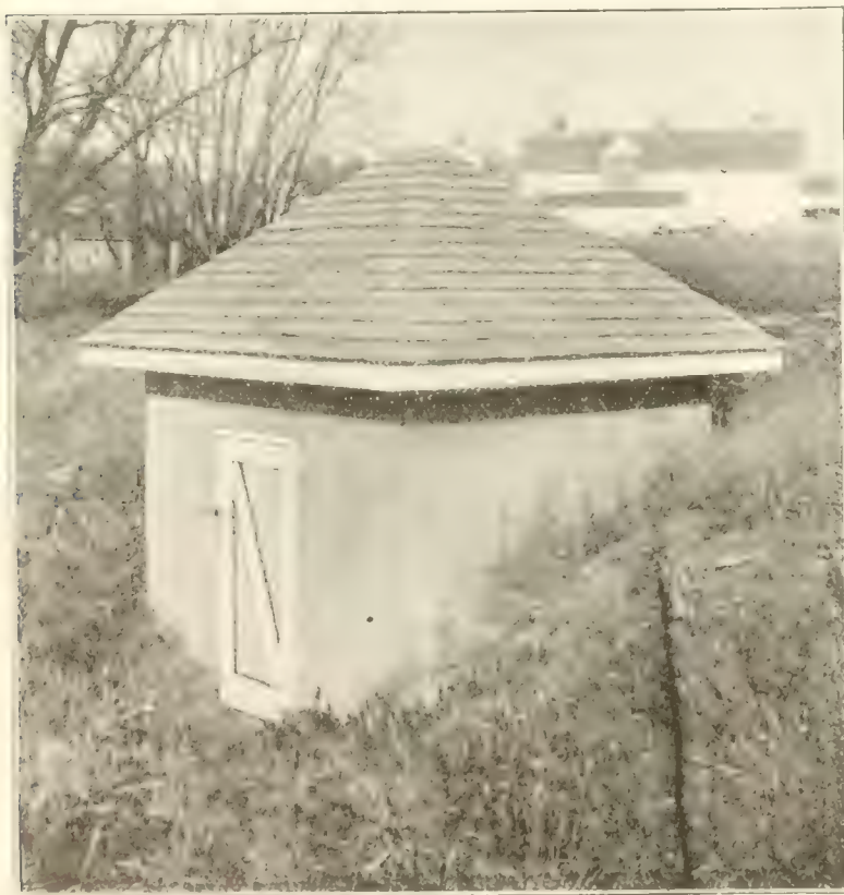
A concrete hydraulic ram house.
