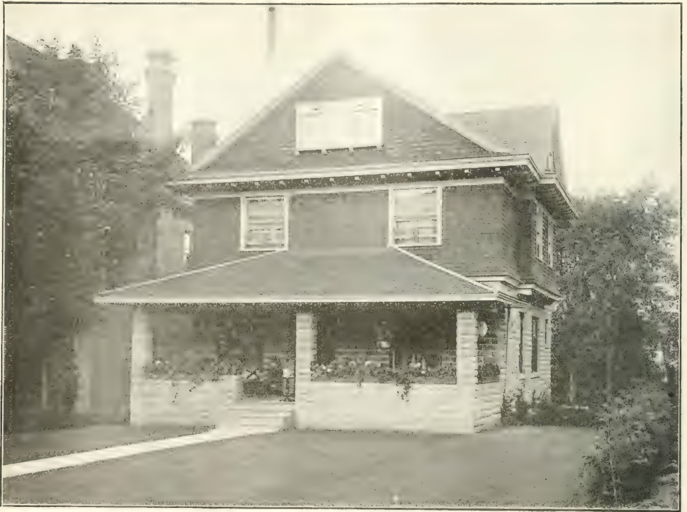
A TTRACTIVE house of R. McDowall, C.E., Owen Sound, Ont. The concrete blocks are hand chipped, resulting in an effect closely resembling stone. Plans were prepared by Architect Forster, Owen Sound, and the house was built by the owner.
