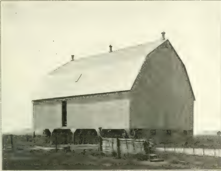
Steel truss barn erected for Nicholas Roth, Shakespeare, Ont. The entire frame of this barn, ready for covering, was erected in one day by ten men.
