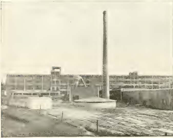
New factory of T. S. Simms & Co., St. John, N.B., designed by Lockwood, Green & Co., Montreal, and built by Aberthaw Construction Co., of reinforced concrete.
