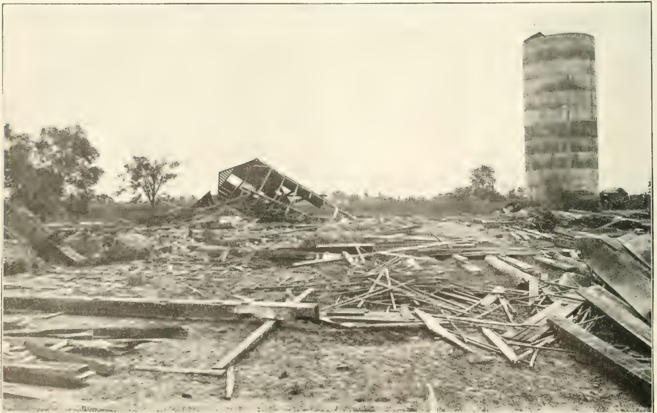
The silo erected by the Polk system of Polk-Genung-Polk Co., Fort Branch, Ind. It is 16 ft. x 45 ft. This picture was taken after a cyclone which destroyed 81 barns, leaving the silo standing.
