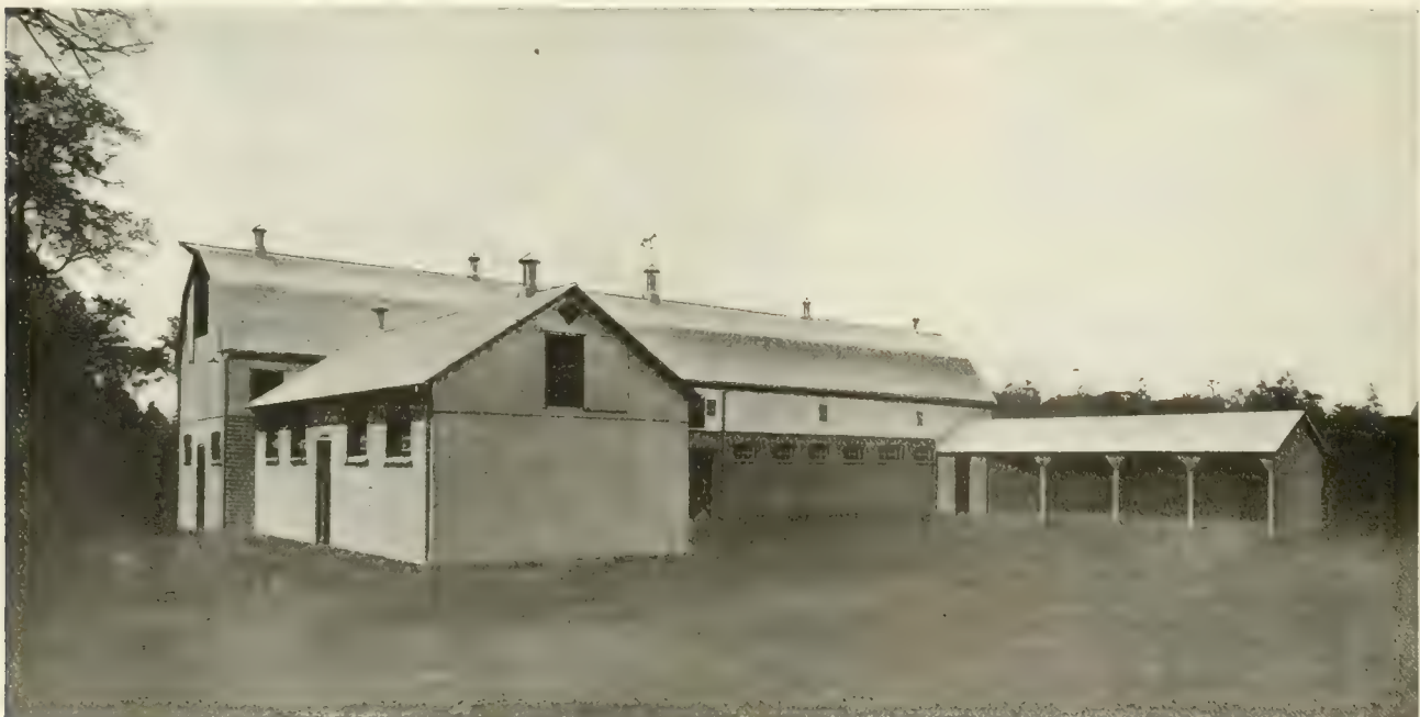
Serviceable new stables of Miss K. L. Wilks, at Orickston Park, Galb., Ont., designed by A. A. Gilmore. The main stable is over 130 feet long. The roof is covered with galvanized "Preston" safe lock shingles, and fitted with "Acorn" barn ventilators. The sides are "Acorn" corrugated galvanized iron, and the eaves are covered with cornice of same make. The lower half of the stable is of brick construction. The sheds and smaller stable are also covered with galvanized metal shingles and side covering.
