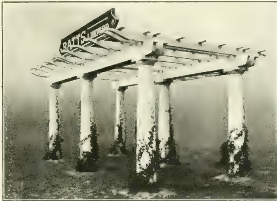
Well-built pergola of neat design. This and the other photos illustrating this article are published by courtesy of Batts, Limited, West Toronto.
