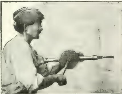
Operating the drill on a vertical wall.
