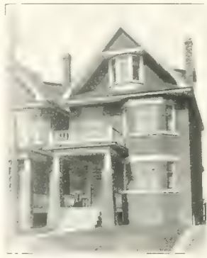
Two houses on Carlaw Ave., Toronto, 8 rooms and sun-rooms at back, shingle roofs, treated as follows: House on left, shingles, eaves of gable and roof stained with Solignum, all paint work with Paripan (3 coat work), interior hardwood filled and varnished, other woodwork painted with same enamel. The owner states that the cost of material was $32.50, labor run into $55. Referring to the house on the right, the shingles were not stained, cost of material was given by the writer of the article, $45, and labor about $60. The difference in cost was due to use of Paripan on the outside.
