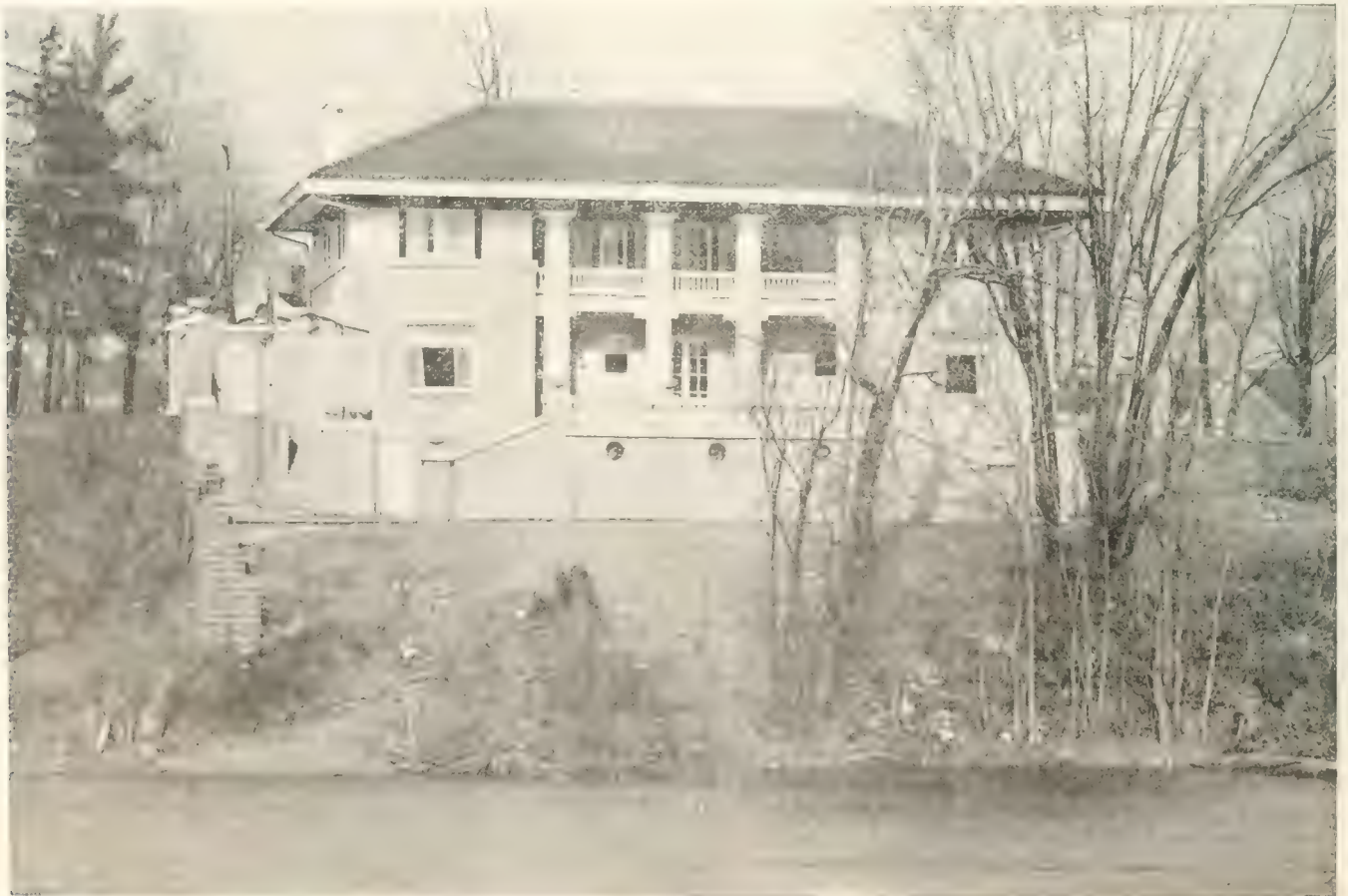
Stucco—Bungalow of Dr. Harter at Elkhart, Indiana.
