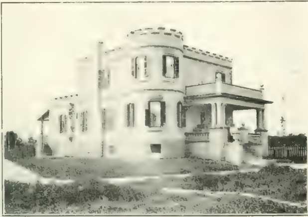
A $5,000 Concrete Block and Stucco House, size 28 x 40 ft., 10 rooms, hot air heat, erected for A. H. Dunning, McKel at Townsite, Ottawa by Boyd Bros., Osgoode.
