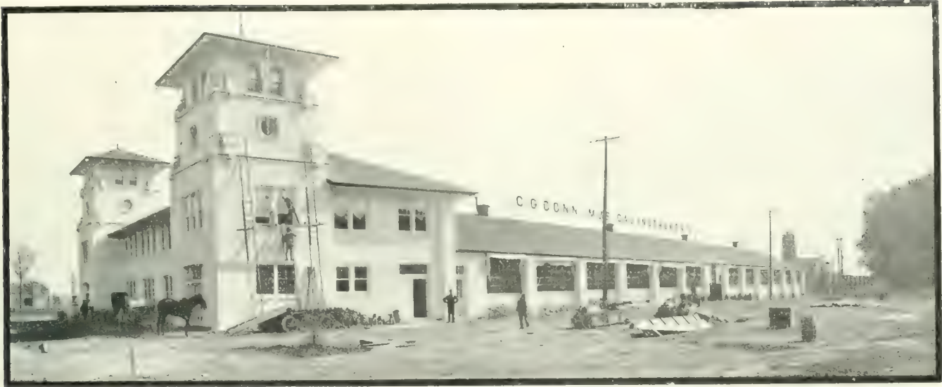
Musical Instrument Factory of Concrete Blocks with Stucco Finish
