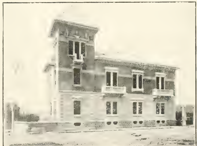
Building erected of concrete blocks in Milan, Italy.
