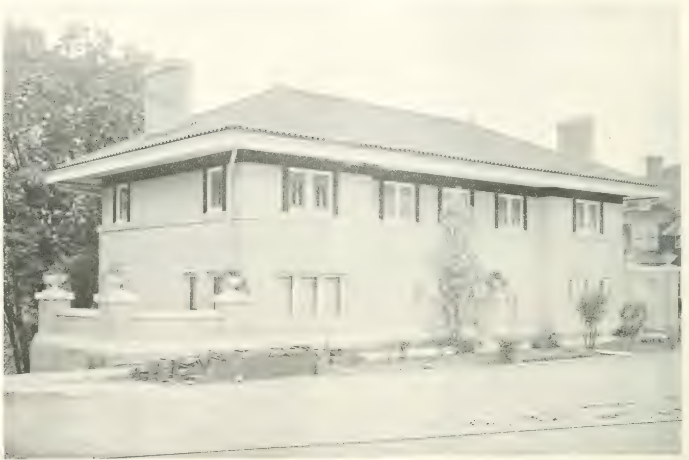
Stucco Bungalow of Dr. Harter at Elkhart, Indiana
