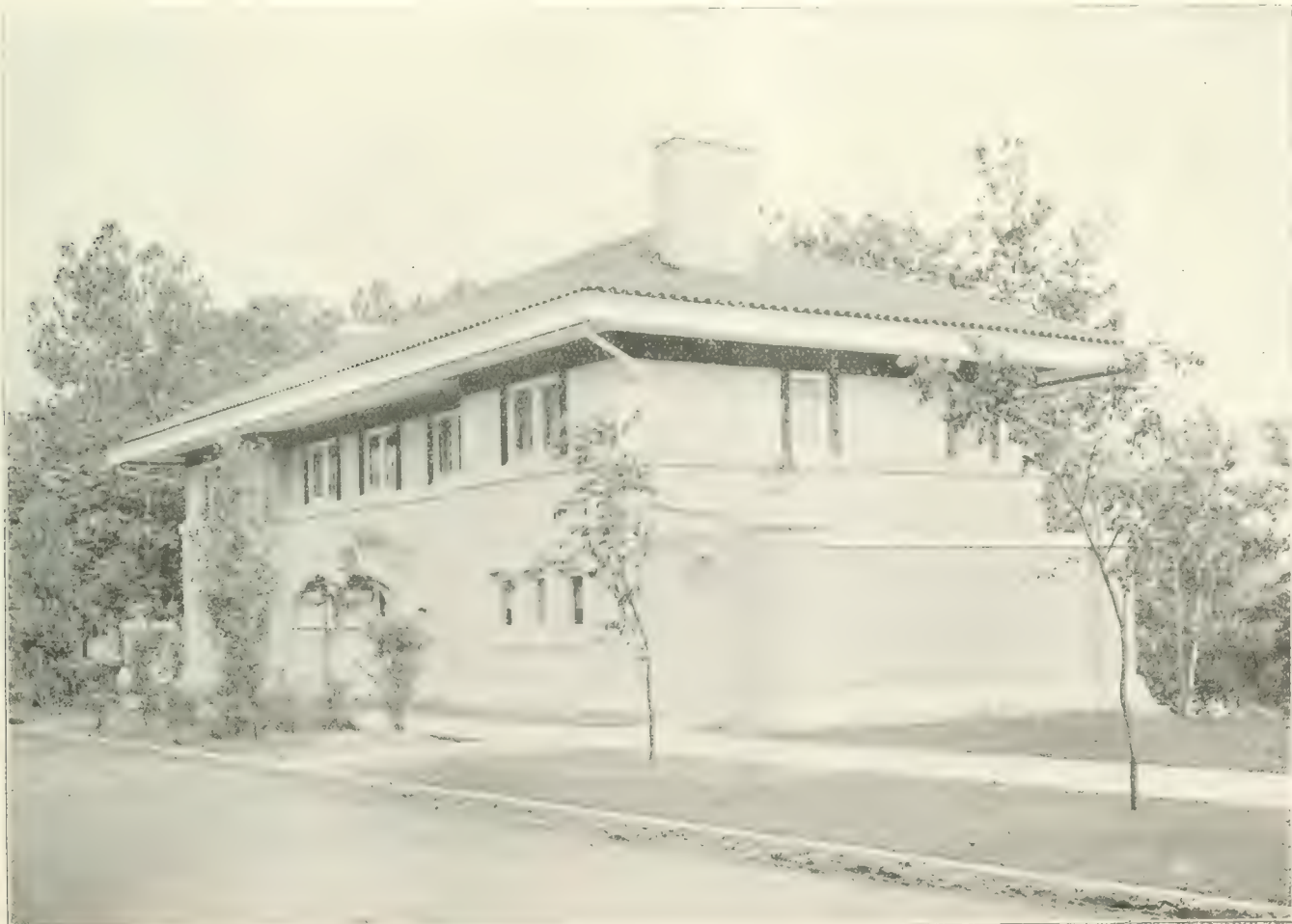
Stucco Bungalow of Dr. Harter at Elkhart, Indiana.
