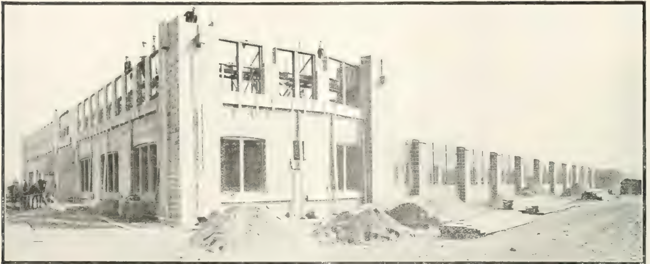
Musical Instrument Factory of Concrete Blocks in Course of Construction.
