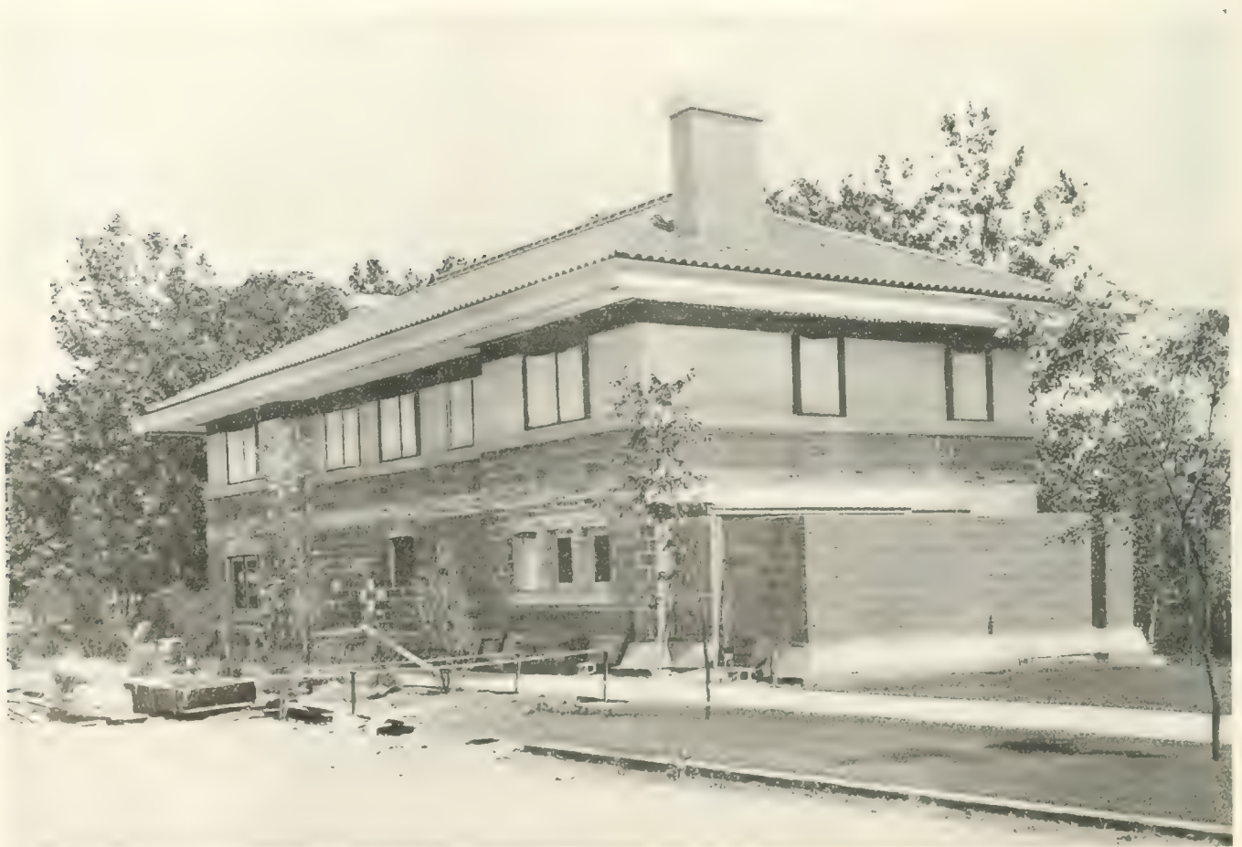
Stucco Bungalow at Elkhart, Indiana, showing Concrete Blocks before Stucco was applied.
