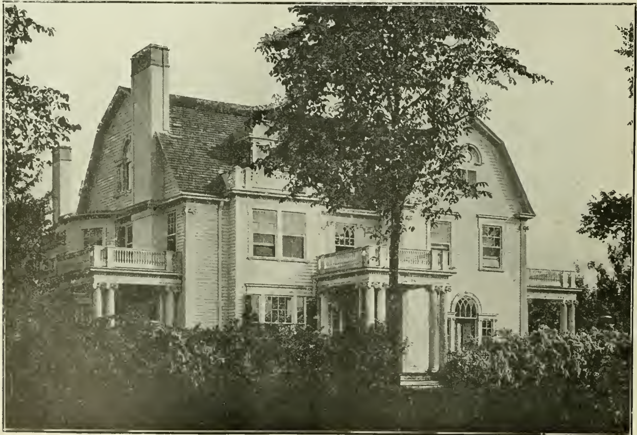
An artistic home covered with asphalt slate shingles, manufactured by Walkerville Roofing Co., Walkerville.
