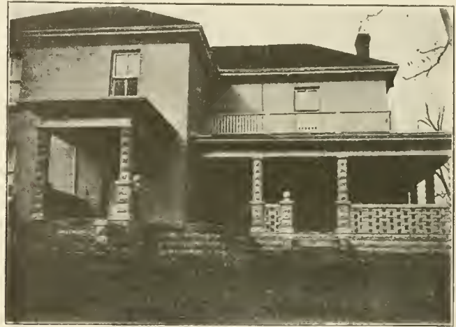
Brick house with cement block verandah erected by W. A. McLenaghan, Builder, Perth, Ont.
