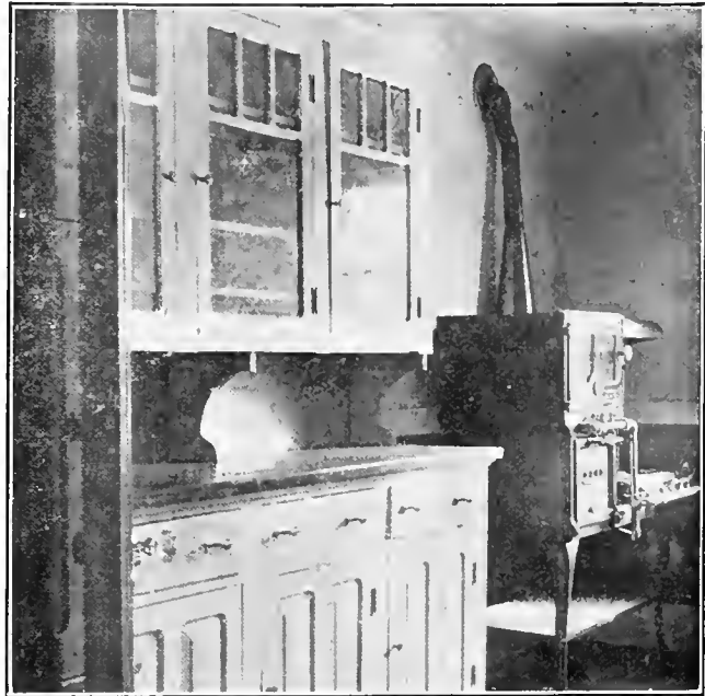
Fig. 3.—View in the kitchen, showing wall cupboard and gas range, with which each suite is furnished. A refrigerator also is supplied.
