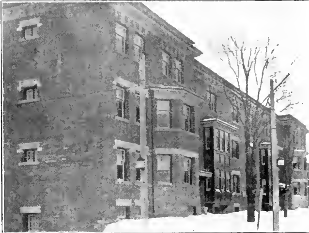
Front view of the Upper Canada Apartments, at the corner of Lonsdale Road and Lawton Avenue, Toronto
