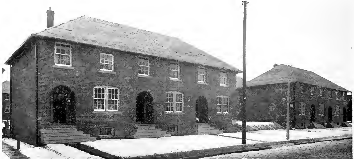
Toronto Housing Co., Spruce St.
