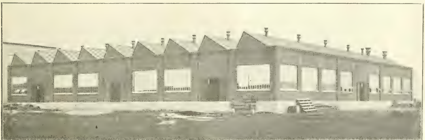
Fig. 1. -New factory building erected by the Remington Arms-Union Metallic Cartridge Co., Windsor.
