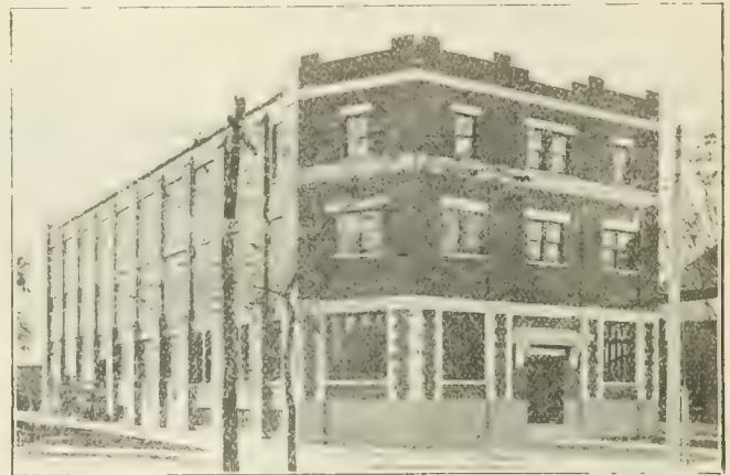
New warehouse designed for Holbrooks, Limited, by T. Pringle & Son, Toronto.
