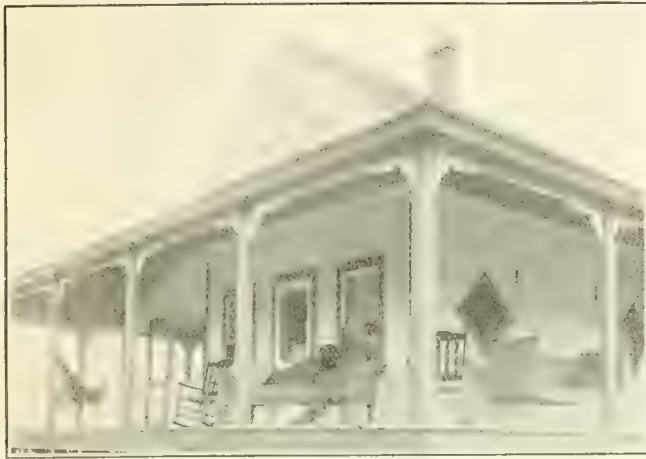
Fig. 1—Cottage with screened-in dining room and wide verandah
