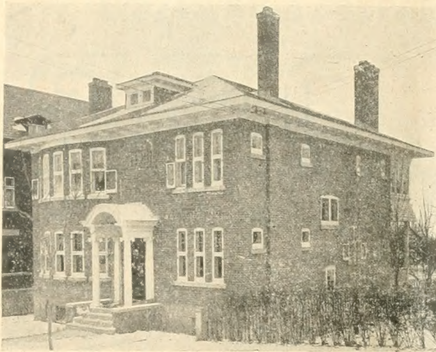
Brick house at Westmount.
