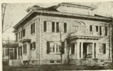
Residence of J. R. Reid, Winnipeg, Man. Keystone Hair Insulator used.
