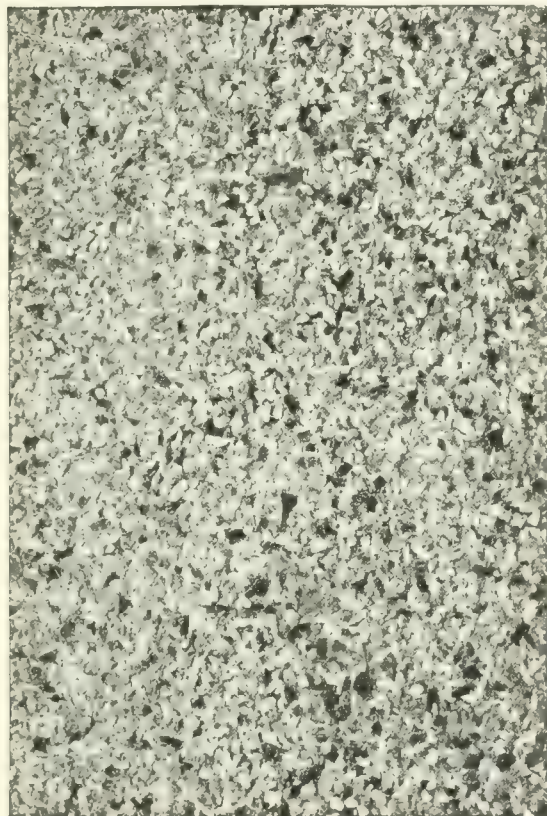
Enlarged View of Granite Smooth Facing
