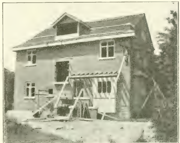
Mr. Crane's house, in course of construction.
