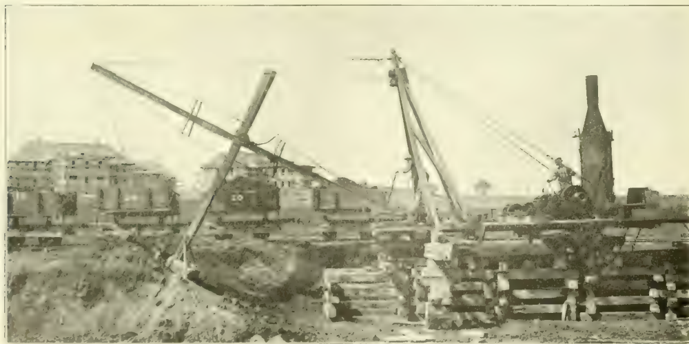
Excavator and steam shovel made at the Prison Farm, Guelph.
