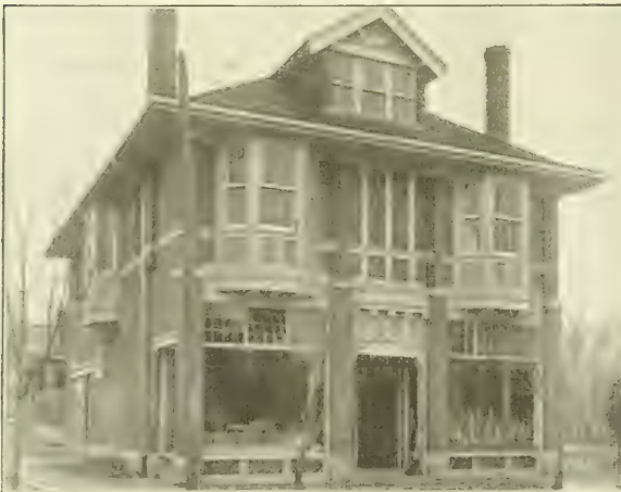
E XTERIOR view of store of W. N. S. Hunter at the corner of Prospect and Maple Avenues, Hamilton, Ont. The store is in a residential section and fits in well with the surroundings. The grocery section is on the right and the butcher shop on the left with separate entrances to each. There is a connecting door inside, however.
