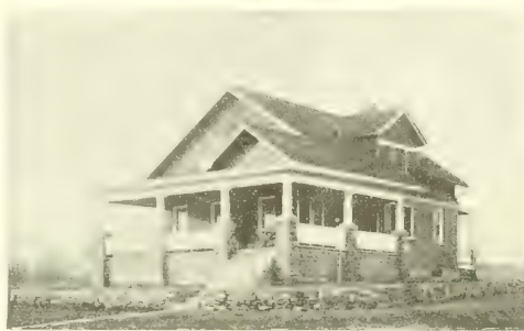
Brick veneer, hilltop cottage at Vineland, Ont. Designed and built by L. R. Fretz.
