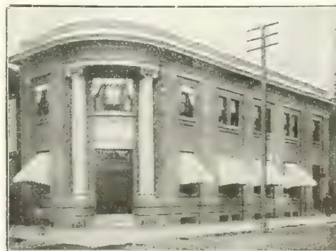
Owner, Molson's Bank, Montreal, Can.; architect, A. J. Dunlap, Lindsay Bldg., Montreal, Can.; contractors, Byers & Anglin, 18 St. Alexis St., Montreal, Can.; block layer, Edward Cox. Erected at Revelstoke, B.C.; frontage 25 ft.; depth 45 ft.; 1,624 faced blocks of horizontally tooled design used; blocks are not waterproof, concrete foundation, hot water heat; cost of block work, $1,080; cost of building complete, $20,850.
