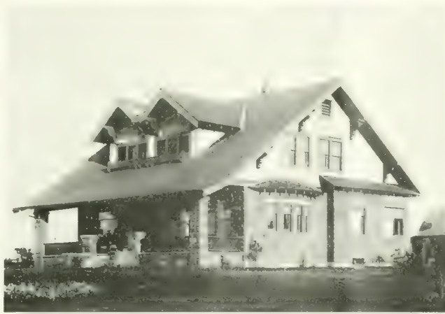
Owner, Judge Smith, Trust Bldg., Ottawa, Canada.; architect, the Bungalow Craft Co., Los Angeles, Calif.; contractors and block layers, Boyd Bros., Osgoode, Ont. Erected at Beaufort House. Frontage 38 ft.; depth 38 ft.; 1,800 8x8x16 in. faced blocks of rock and panel designs used. Building has concrete foundation, 9 rooms, hot water heat. Cost of block work, $750.00; cost of building complete, $1,400.
