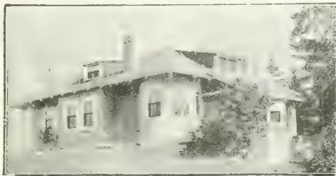
Owner, G. W. Daniels, St. Stephens, New Brunswick; architect, Mrs. G. W. Daniels; contractor and block layer, Emerson B. Hanson, St. Stephens, N.B. Frontage 39 ft.; depth 41 ft.; 2,000 8x8x16 in. faced blocks of rock design used. Building has 9 rooms and hall, stone and brick foundation, hot air heat, and is free from dampness. Completed Aug. 1910. Cost of block work, $700; cost of building complete, $1,400.
