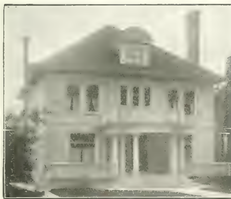
Owner, Thos. I. Dates, Owen Sound, Ont.; architect, E. C. VanLeyan, Detroit, Mich.; contractor, Edward Martyn, London, Ontario; block layer, T. Banks. Erected at Owen Sound, Ontario. Frontage, 37 ft. 6 in.; depth, 37 ft. 6 in.; 6,250 8x8x16 in. and 8x10x16 in. faced blocks of vertically tooled and plain designs used. Building has Ideal block foundation, has hot air heat, 10 rooms and is perfectly dry; temperature of 70 deg. maintained throughout the cold winter on 8 1/2 tons of coal. Cost of block work, $1,350.00; cost of building complete, $5,650.00.
