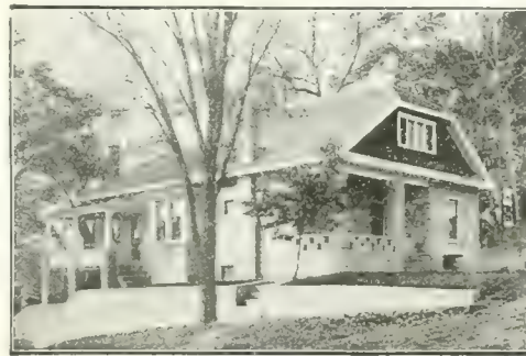
Owner, Rev. Austin Potter, Dundas, Ont.; architect, Martyn H. Hewitt, Dundas, Ont.; contractor, J. W. Dickson, Dundas, Ont.; frontage, 30 ft.; depth, 40 ft.; 1,800 8x8x16 in. faced blocks of rock and Bush Hammered design used. House has concrete foundation, 8 rooms, hot air heat and is free from dampness. Cost of blocks, $315; cost of building complete, $2,600.
