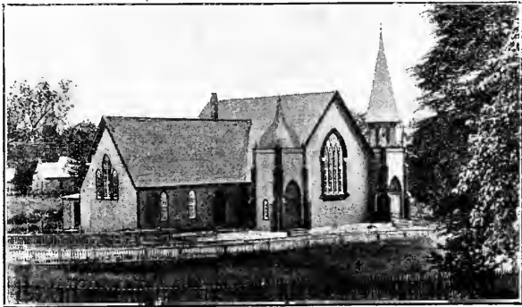
CONGREGATIONAL CHURCH. LIVERPOOL, N.S.
