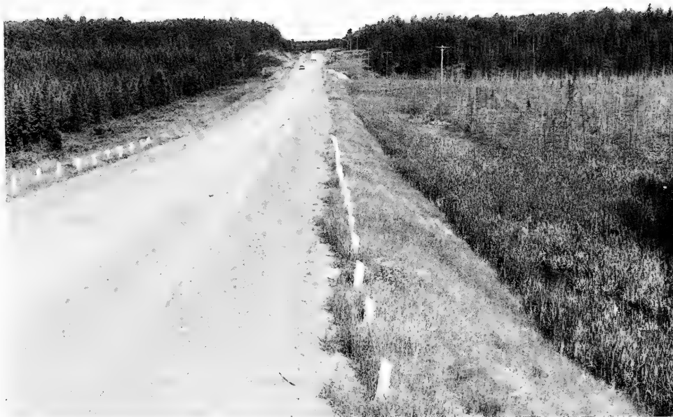
FIGURE 1. Ground photograph of the road dam. The open peatland is to the right, the treed peatland to the left. Cat-tails ( Typha latifolia ) are in the ditch on the right. The view is from southeast to northwest.
