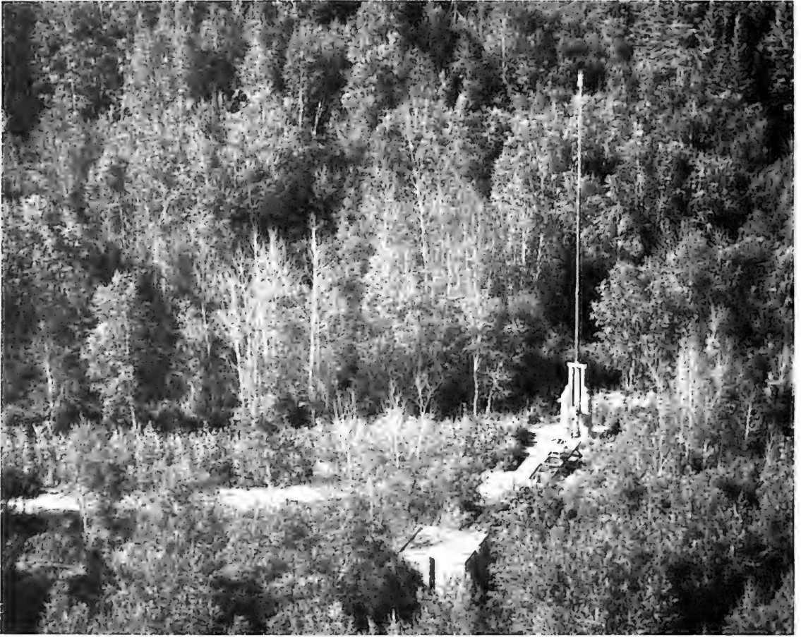
FIGURE 2. FIG irradiation tower photographed in 1973, showing the 20 m tower, tower supports, beam stop, plantation, service road, and mixed boreal forest.
