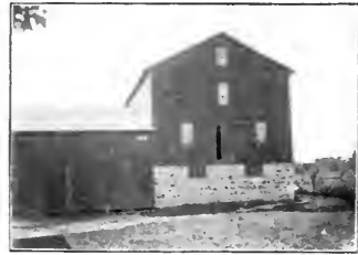
FIG. 1478.—MR. FISHER'S FRUIT HOUSE. first in the Burlington district to plant largely of grapes, and to demonstrate
