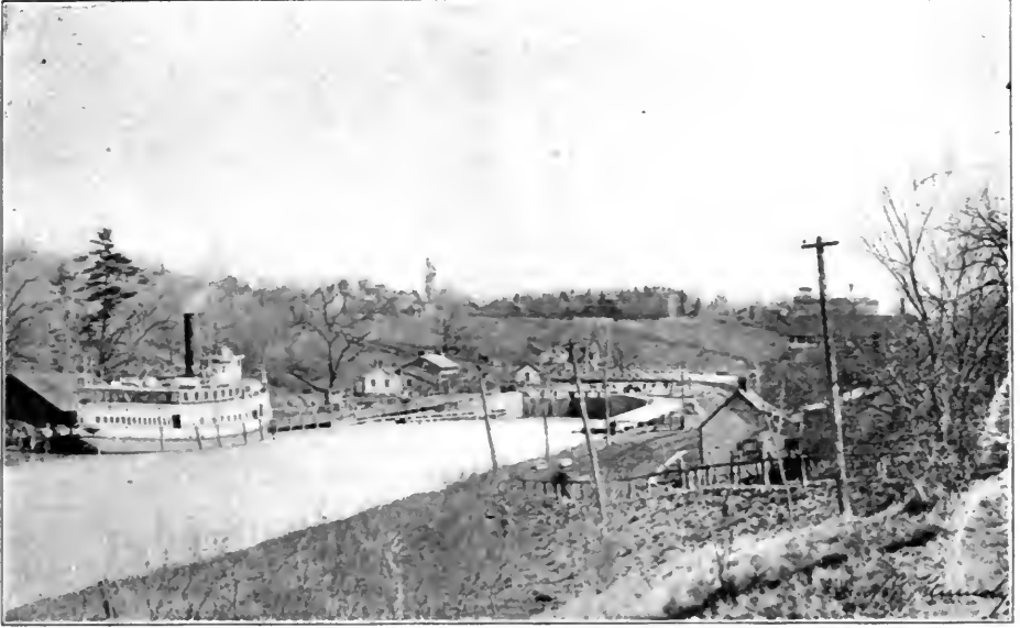
FIG. 1498.—LOCK 2, OLD WELLAND CANAL.
