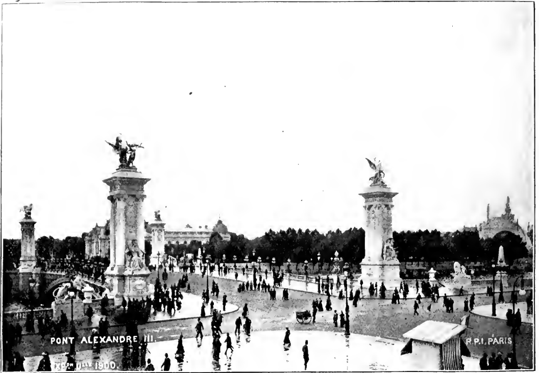
FIG. 2011. ALEXANDER III BRIDGE, PARIS.
