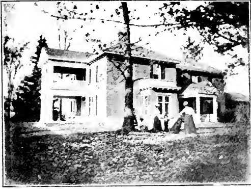
FIG. 2192. RESIDENCE OF H. MUSSEN.
