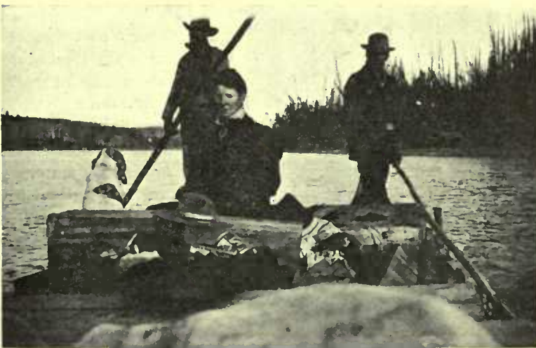
The raft and its crew floating down the Peace River.
