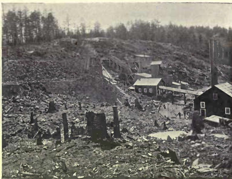
The power and crushing plant, open pit and ore stock pile, Moose Mountain Mines.
