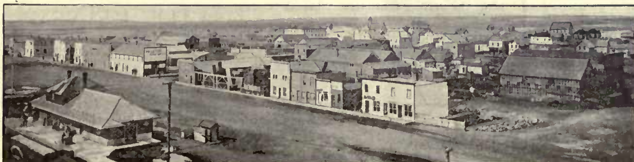
A view of the town of Hanley, Sask., from one of the elevators.
