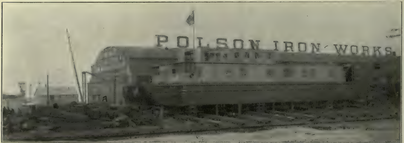
Fig. 1.—The Dredge Shuniah Before Launching, Polson Iron Works, Toronto.
