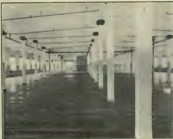
Construction of Fairbanks-Morse New Warehouse.
