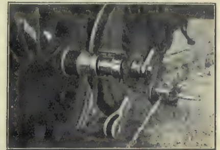
Portable Crank Pin Turner.
