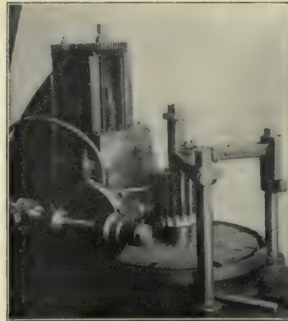
Farwell Gear Hobber Cutting Pinion.
