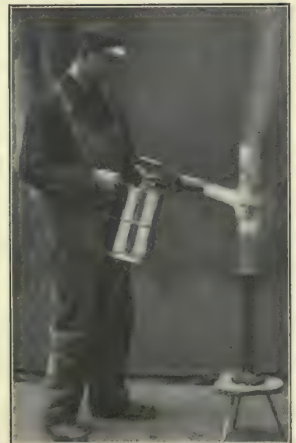
Brazing a Cup Joint With Kerosene Lamp.
