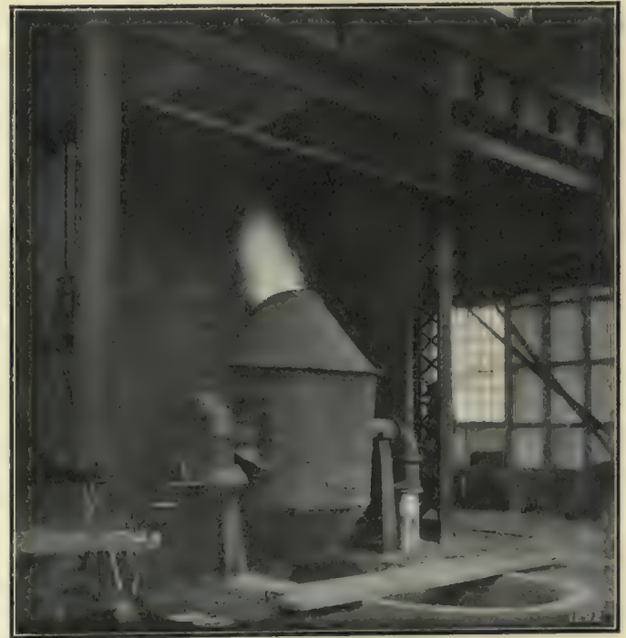
Fig. 5.—Converter During Progress of the Blow.
