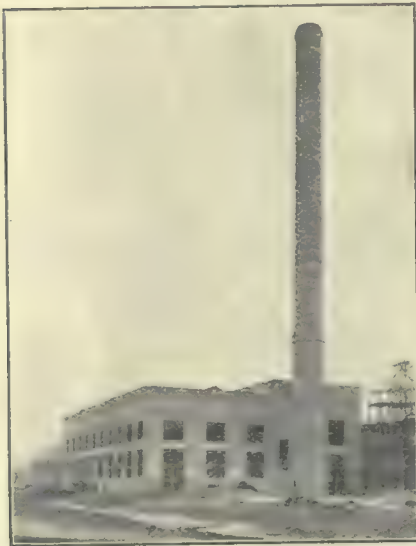
G.T.P. Power House Where 4,000 H.P. is Generated and Chimney 200 ft. High.
