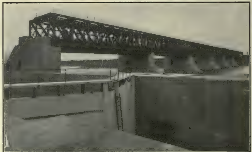
Fig. 2.—View of Dam With Curtain Frames Raised, Also Upper End of Lock Chamber.
