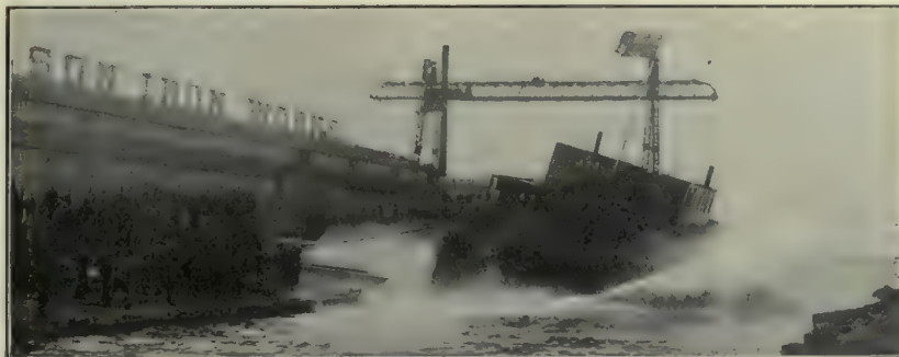
Fig. 3.—Launching New Dredge at Polson Iron Works, Toronto.
