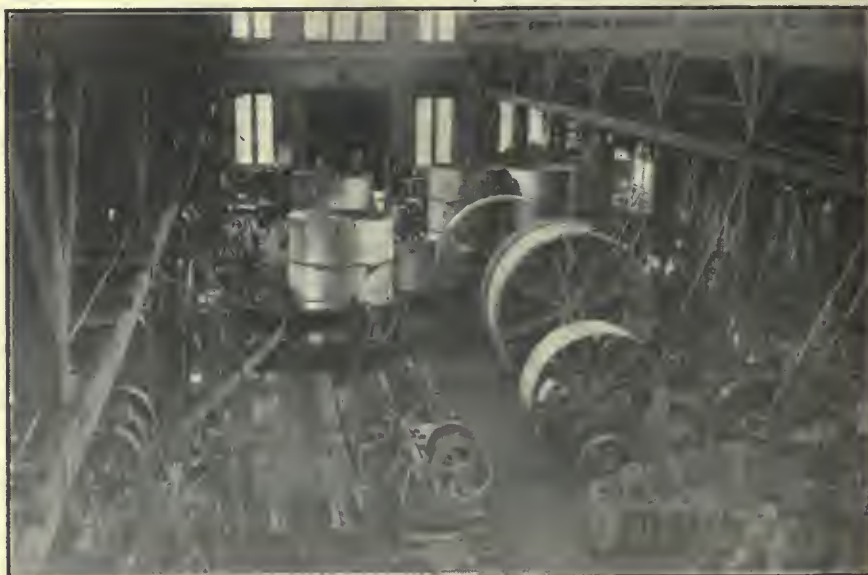
FIG. 13. INTERIOR OF MACHINE SHOP LOOKING SOUTH.
