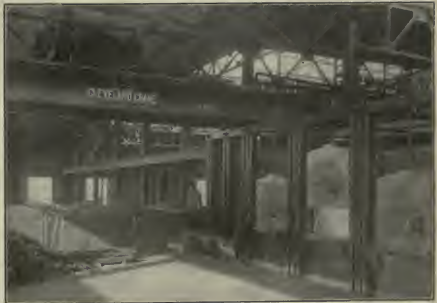
CHARGING PLATFORM, NO. 1 OPEN HEARTH FURNACE. IN THE BACKGROUND IS SEEN ONE OF THE DRYING OVENS UNDER CONSTRUCTION.
