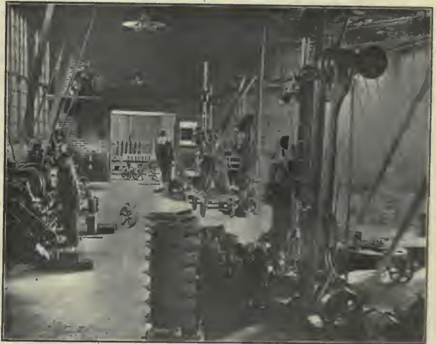
FIG. 10. A SECTION OF THE HANGER SHOP.
