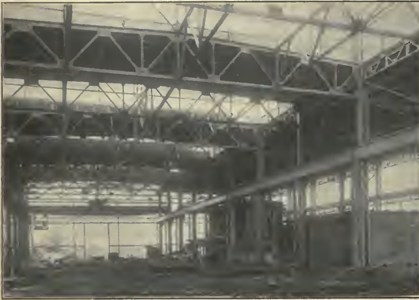
MAIN BAY OF FOUNDRY WITH DRYING OVENS AND NO. 1 OPEN HEARTH FURNACE UNDER CONSTRUCTION.
