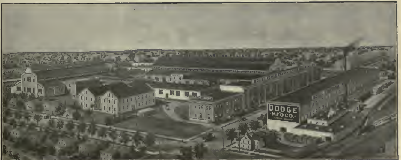
FIG. 1. BIRD'S EYE VIEW OF DODGE MFG. CO. PLANT.
