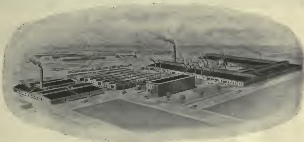
VIEW OF WORKS. THE GEO. WHITE & SONS, CO., LTD., LONDON, ONT.
