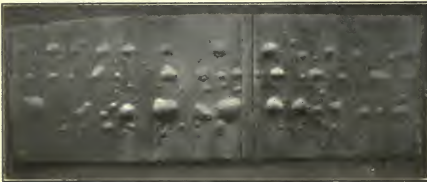
PHOTOGRAPH OF BLISTERED STEEL SHEET.
