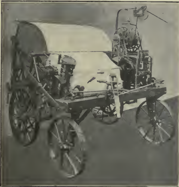
FIG. 1. FRONT VIEW OF SAND MIXING MACHINE.
