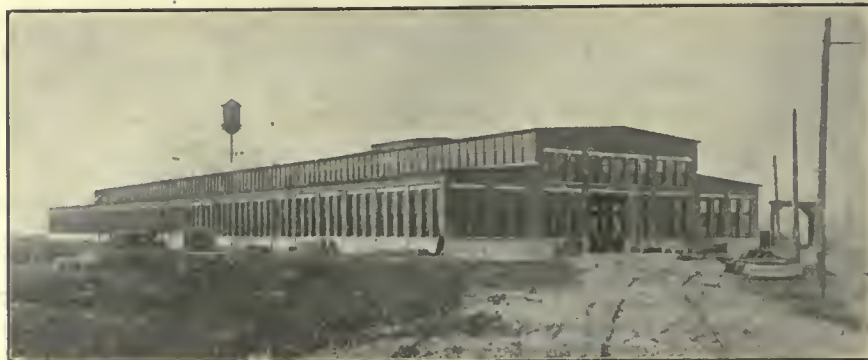
BOILER SHOP OF THE GOLDIE & McCULLOCH CO., LTD., GALT, ONT.
