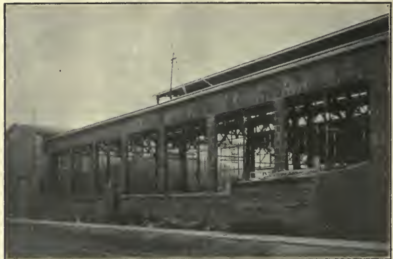
NEW FOUNDRY OF SHELDONS, LTD.—UNDER CONSTRUCTION.
