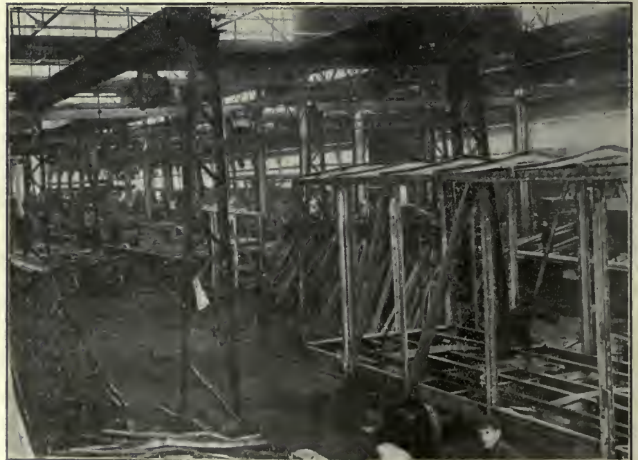
STEEL ERECTION DEPARTMENT.
