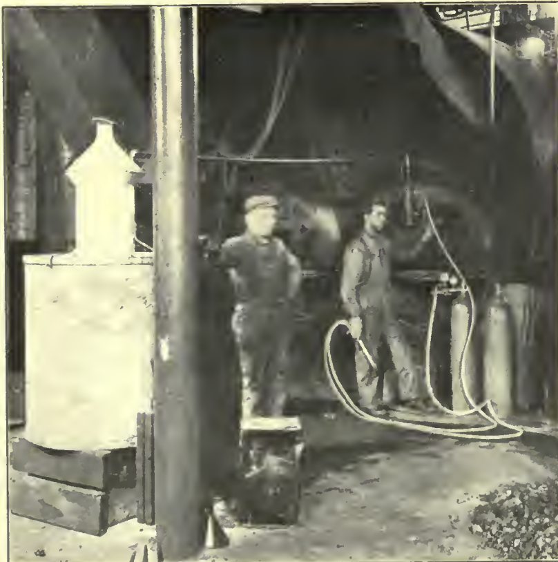
FIG. 3. PREPARING TO REPAIR A BOILER FRACTURE.
