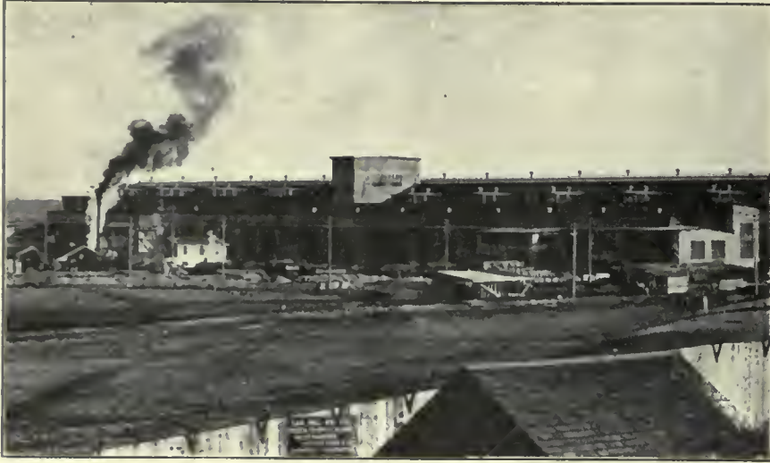
MAIN BUILDING FROM WEST, SHOWING BLACKSMITH AND BOILER SHOP BAYS.
