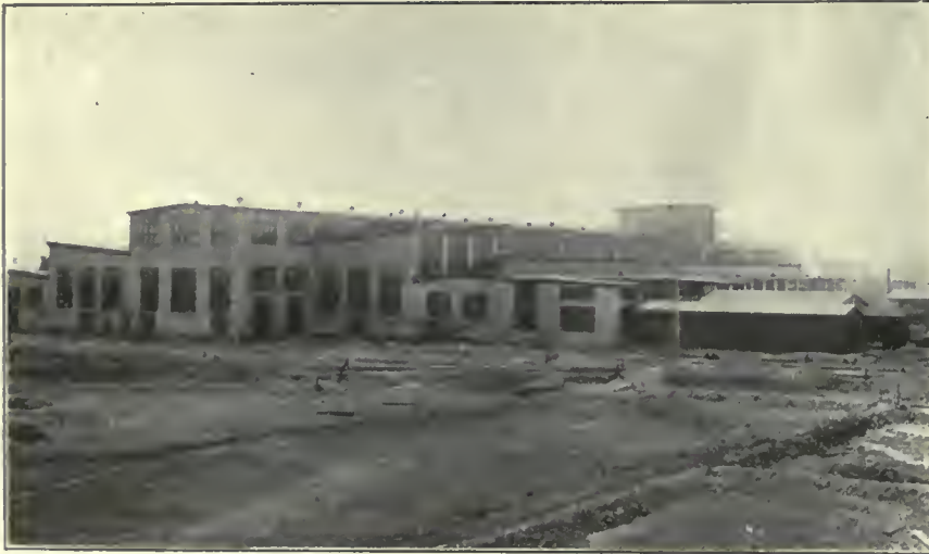
NORTH-WEST VIEW SHOWING ROOF ARRANGEMENTS WITH REFERENCE TO LIGHTING OF ERECTING AND MACHINE SHOPS.
