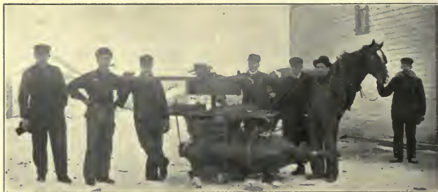
BORING 30 IN. SLUICE VALVE, CHUCKED TO EARTH AT TEMPERATURE 48 DEGREES BELOW ZERO.
