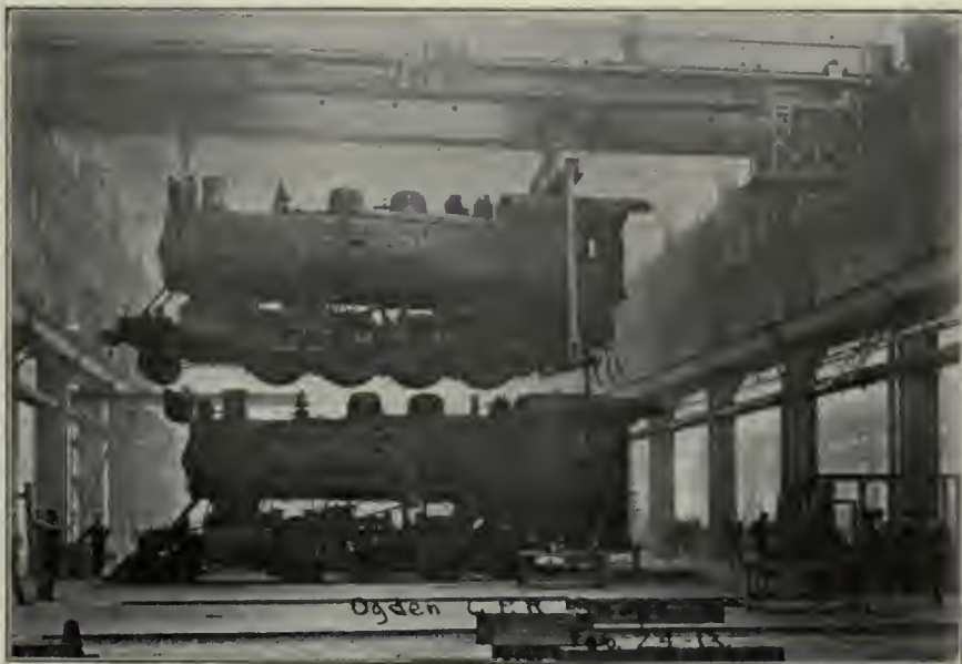
INTERIOR OF LOCOMOTIVE SHOPS, SHOWING 120 TON LOCOMOTIVE CRANE.
