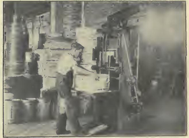
FIG. 6. WOOD PULLEYS BEING NAILED ON NAILING MACHINE.
