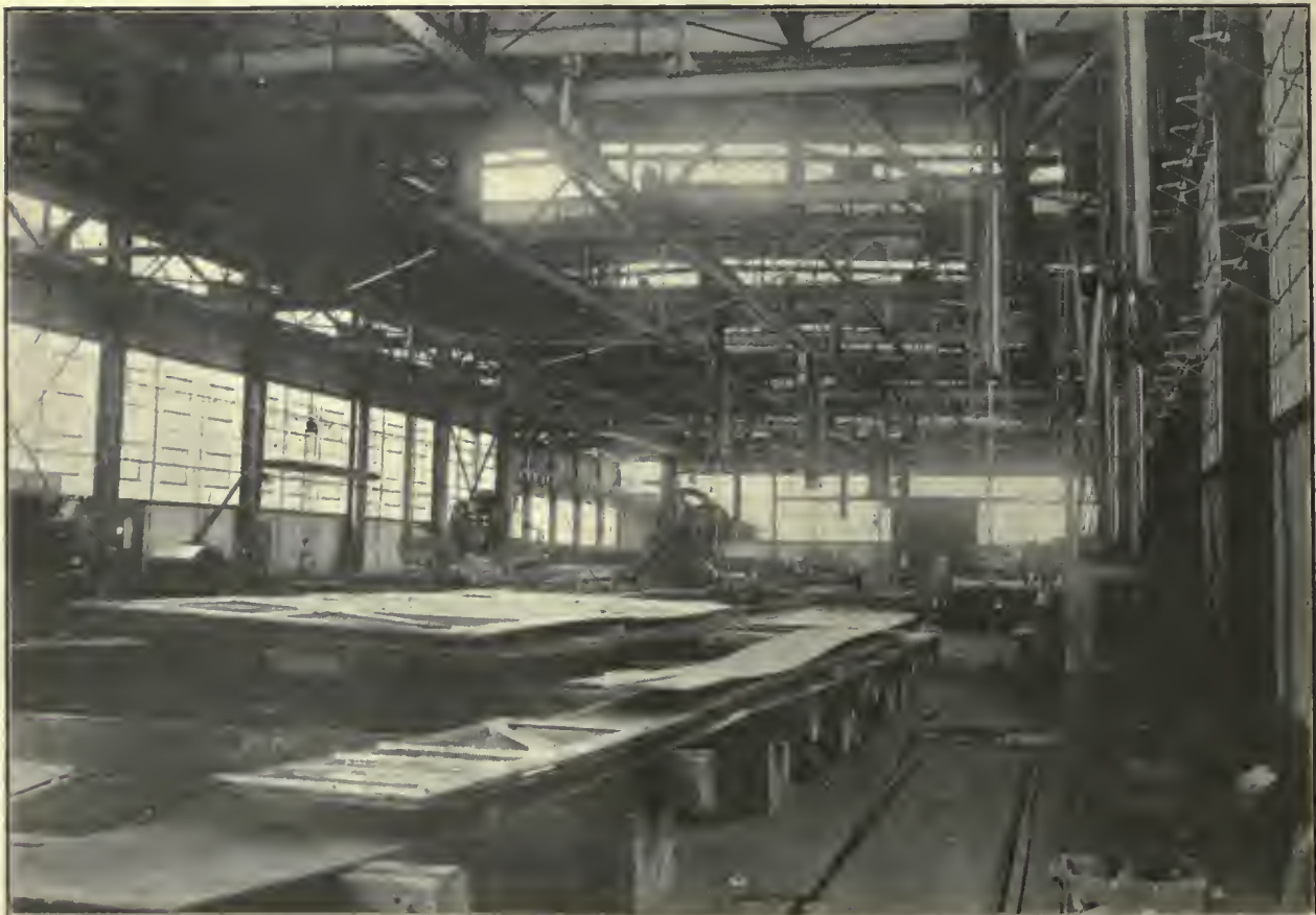
FIG. 3. INTERIOR OF STRUCTURAL SHOP LOOKING WEST. IN THE FAR CORNER IS SEEN THE 80 FT. OPENING INTO THE GIRDER SHOP. ILLUSTRATION SHOWS LONGITUDINAL TRAVELLERS FOR RIVETERS AND AIR HOISTS RUNNING CROSSWAYS ON LOWER CHORDS OF ROOF TRUSSES.
