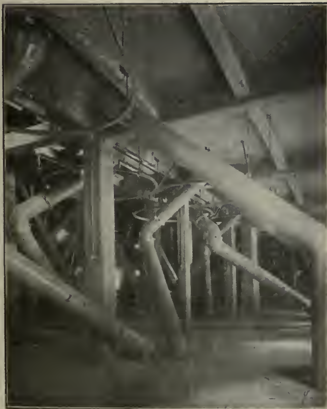
FIG. 4. DISTRIBUTING SPOUTS. STOREY OVER BINS.
