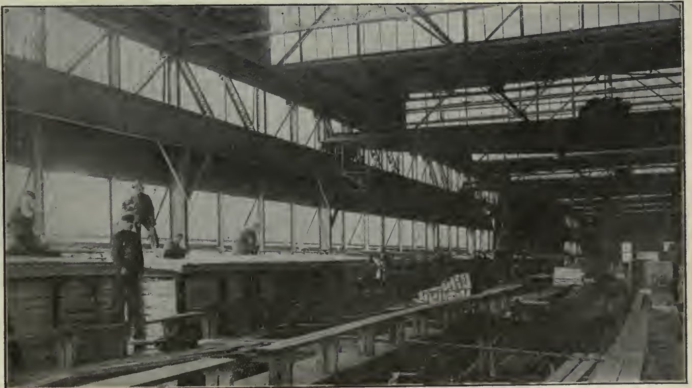
WOOD ERECTION DEPARTMENT.
