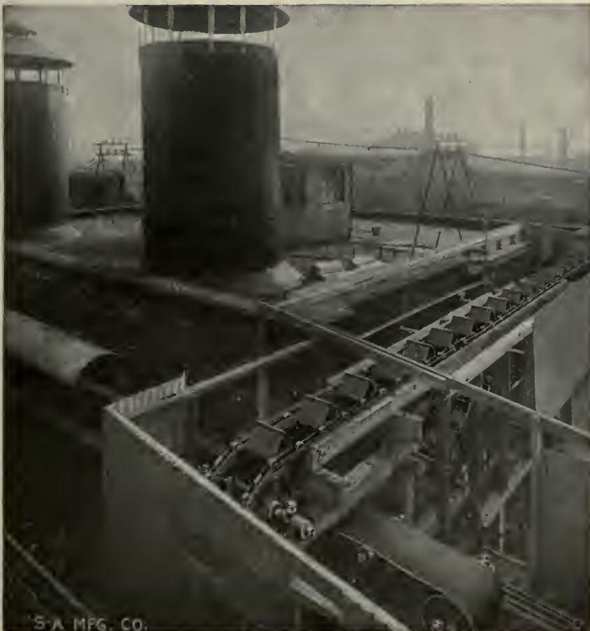
FIG. 1. CONVEYER-ELEVATOR AND BELT CONVEYER.
