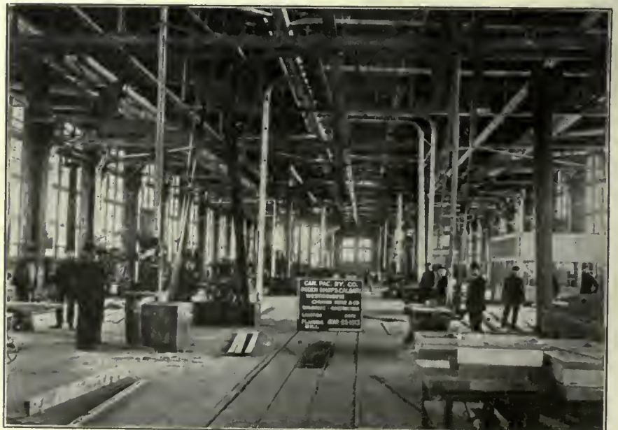
INTERIOR OF PLANING MILL.
