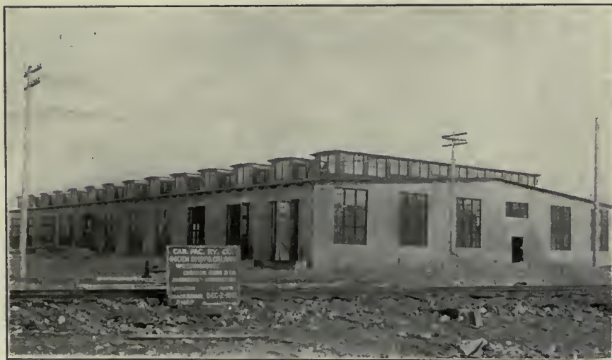
COACH REPAIR SHOP.
