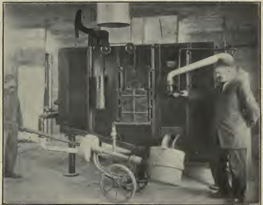
EMPIRE MFG. CO. NEW 3,500 LB. OIL-FIRED BRASS SMELTING FURNACE
