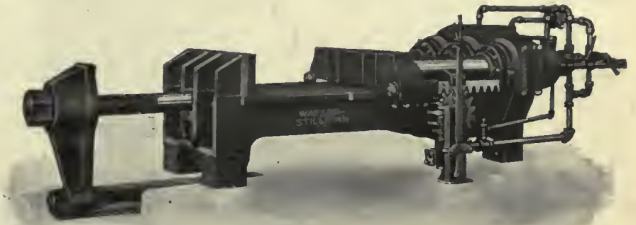
AN HYDRAULIC BULLDOZER.
