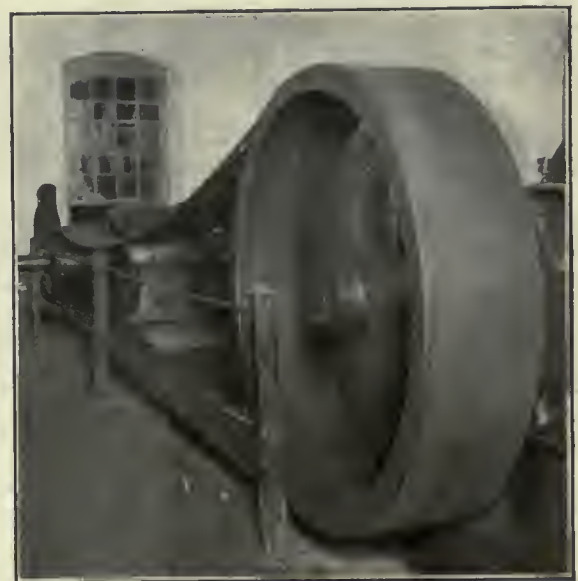
FIG. 1. TYPICAL EXAMPLE OF BELT DRIVE UNDER NON-SLIP TREATMENT.
