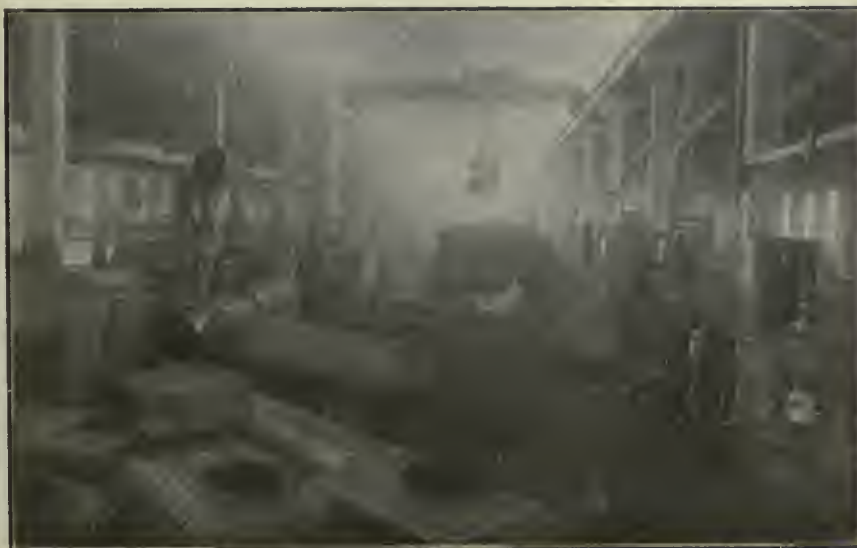
INTERIOR OF BOILER SHOP.
