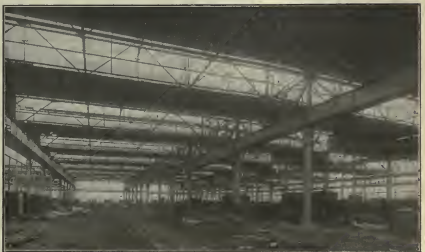
INTERIOR OF MAIN SHOP, NATIONAL STEEL CAR CO. NEW PLANT.
