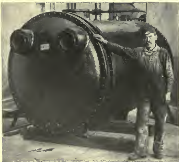
LARGE HOT WATER HEATER.
