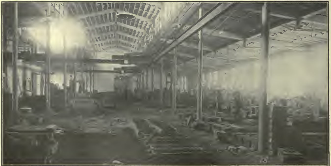
INTERIOR VIEW OF FOUNDRY LOOKING SOUTH. Note the overhead Mono-Rail Runway which here takes the place of a Travelling Crane.
