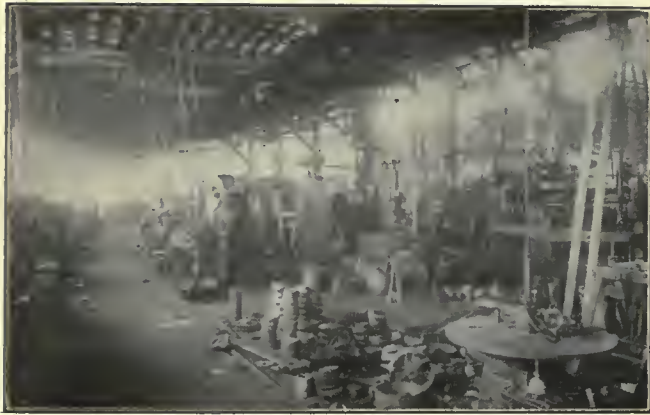
A VIEW IN THE MACHINE SHOP.
