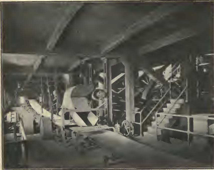
FIG. 5. BELT CONVEYORS IN SECOND STOREY OVER BINS.
