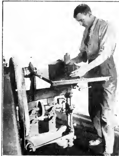
FIG. 2. DRUM ATTACHMENT, BESLY PATTERNMAKERS' GRINDER.
