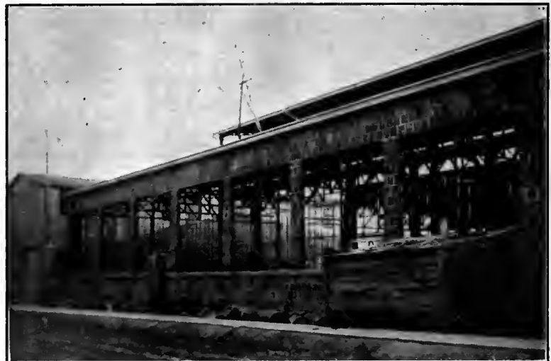
NEW FOUNDRY OF SHELDONS, LTD.—UNDER CONSTRUCTION.
