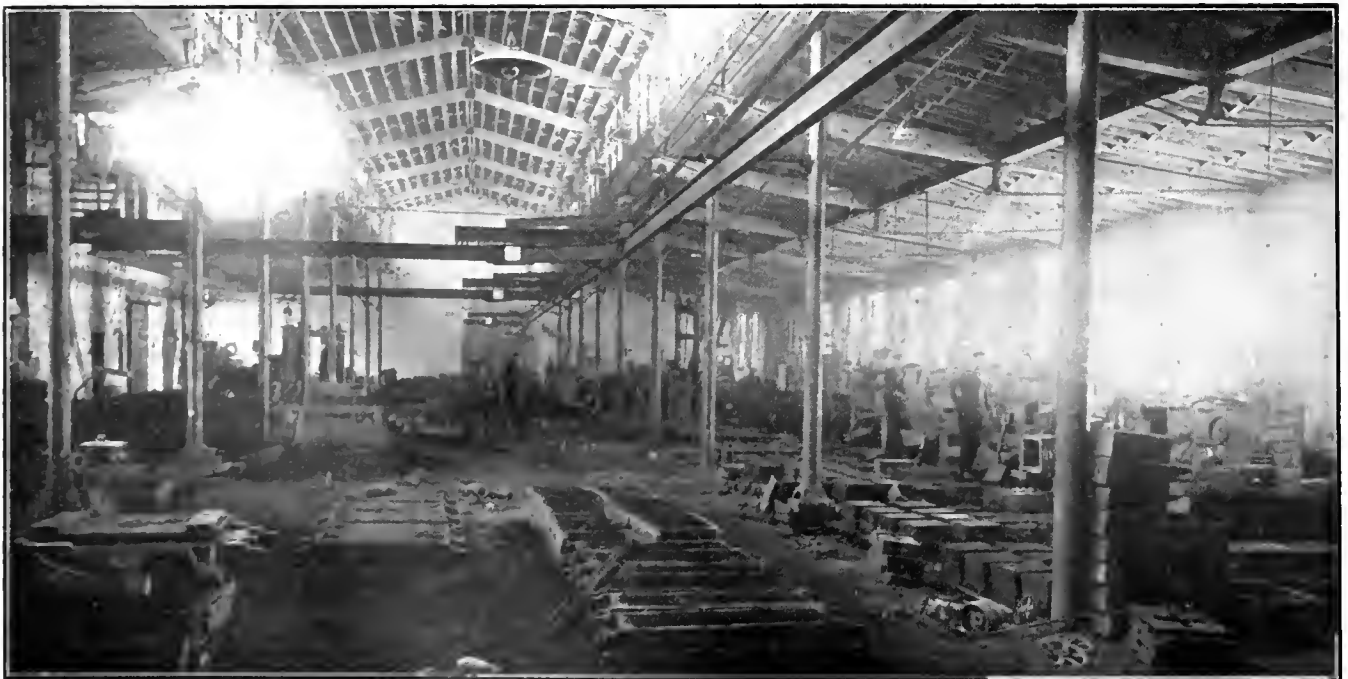
INTERIOR VIEW OF FOUNDRY LOOKING SOUTH. Note the overhead Mono-Rail Runway which here takes the place of a Traveling Crane.
