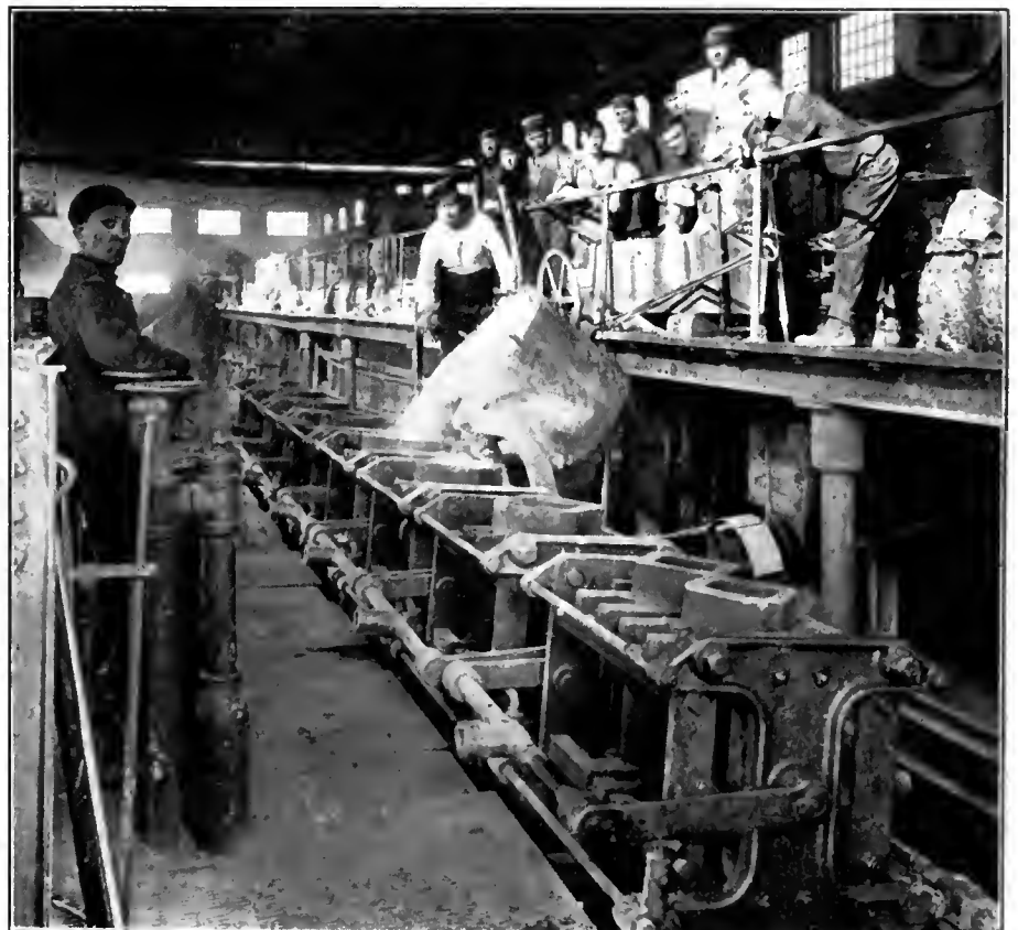
FIG. 4. CASTING THE INGOTS FROM AN HYDRAULICALLY OPERATED TOP POUR LADLE.
