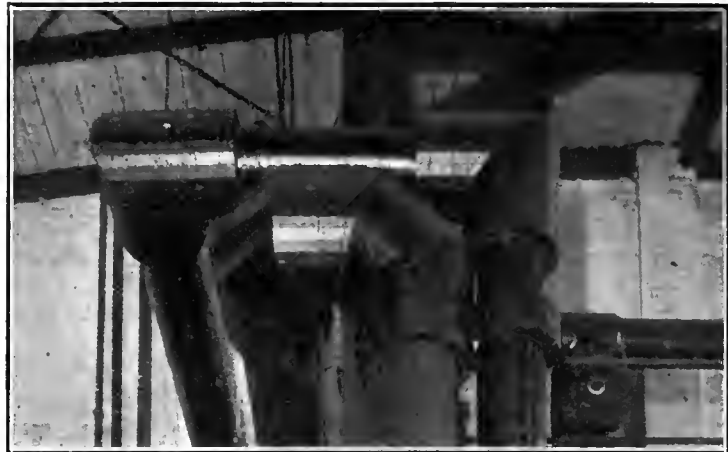
FIG. 3. A DIFFICULT PIECE OF PIPE COVERING. CORK COVERING ON 8 IN. X 12 IN. FLANGED BRINE PIPING.
