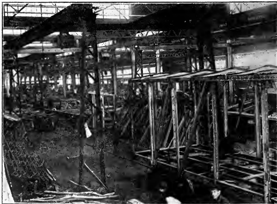
STEEL ERECTION DEPARTMENT.
