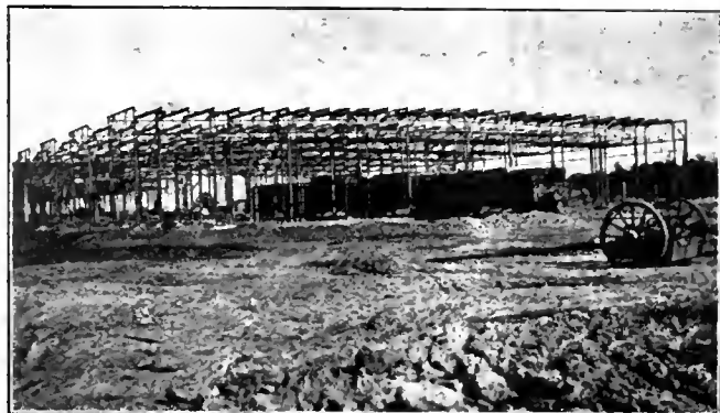
NATIONAL STEEL CAR CO. NEW PLANT. PAINT SHOP UNDER CONSTRUCTION.
