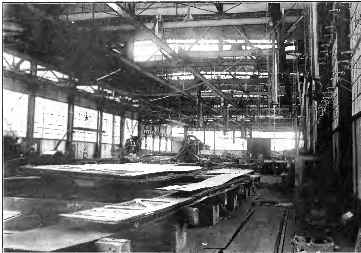
FIG. 3. INTERIOR OF STRUCTURAL SHOP LOOKING WEST. IN THE FAR CORNER IS SEEN THE 80 FT. OPENING INTO THE GIRDER SHOP. ILLUSTRATION SHOWS LONGITUDINAL TRAVELLERS FOR RIVETERS AND AIR HOISTS RUNNING CROSSWAYS ON LOWER CHORDS OF ROOF TRUSSES.
