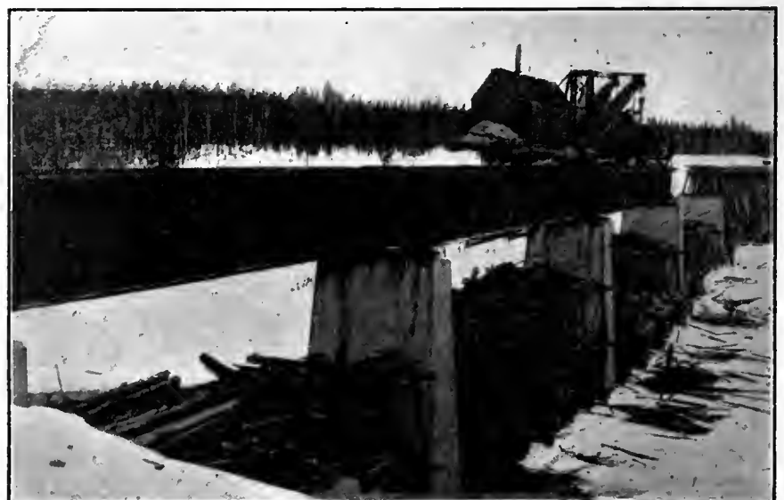
FIG. 9. ERECTION CAR PLACING 100 FT. DECK PLATE GIRDER IN POSITION.
