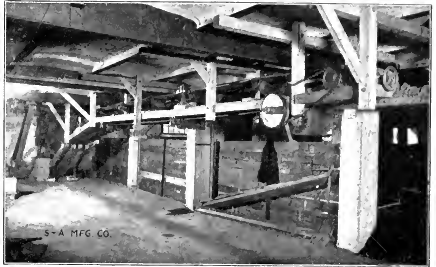
FIG. 2. CONVEYER IN BASEMENT.
