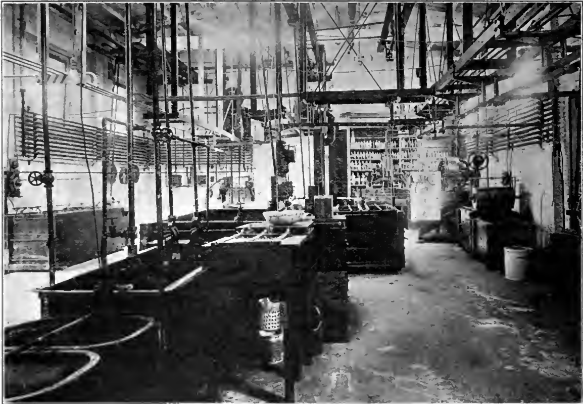
GENERAL VIEW OF THE ELECTRO-PLATING DEMONSTRATION PLANT, CANADIAN HANSON & VAN WINKLE CO., LTD.
