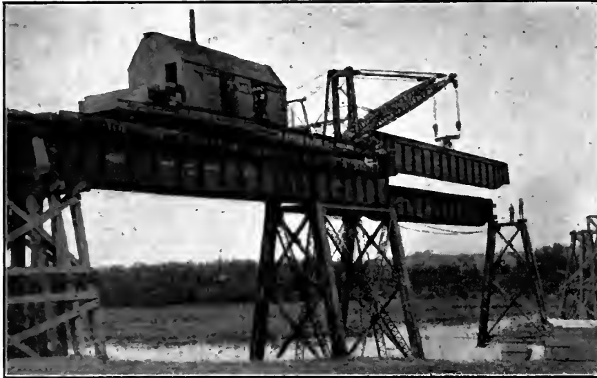
FIG. 8. DERRICK CAR ERECTING 80 FT. SINGLE TRACK GIRDER SPAN.
