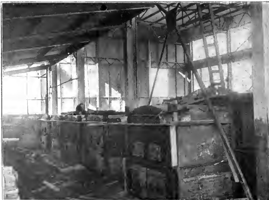
ANNEALING FURNACE FIRING PIT.
