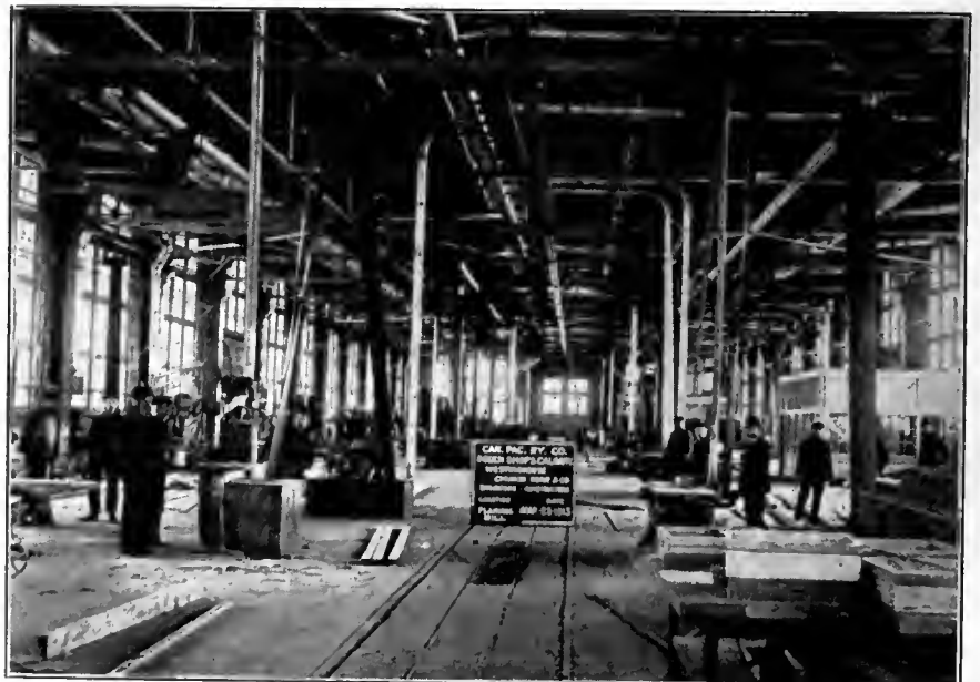
INTERIOR OF PLANING MILL.
