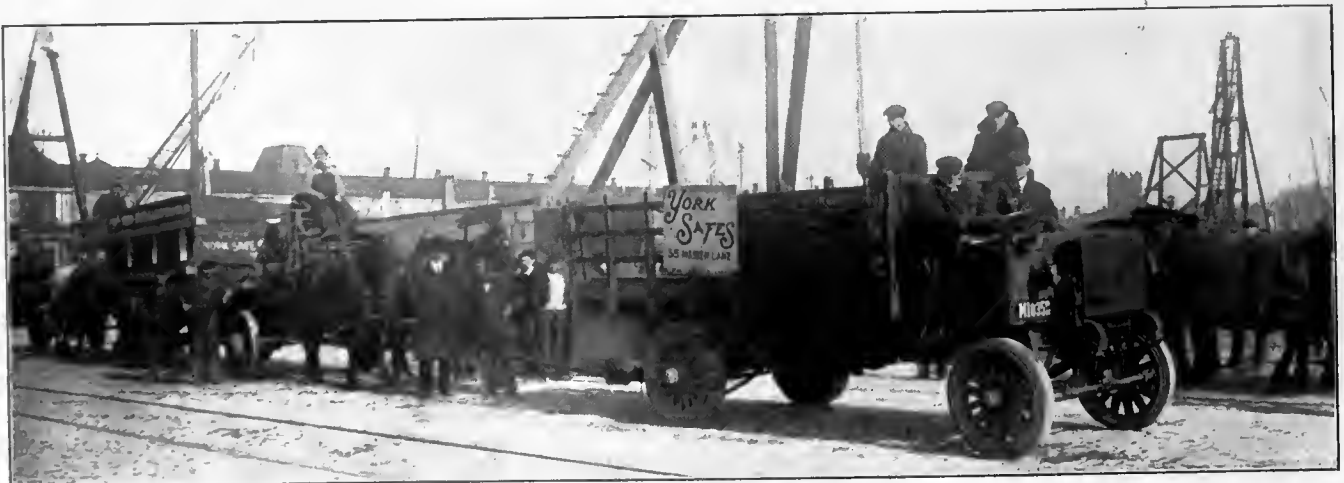
HYDRAULIC TRANSMISSION TRUCK HAULS 45-TON LOAD.
