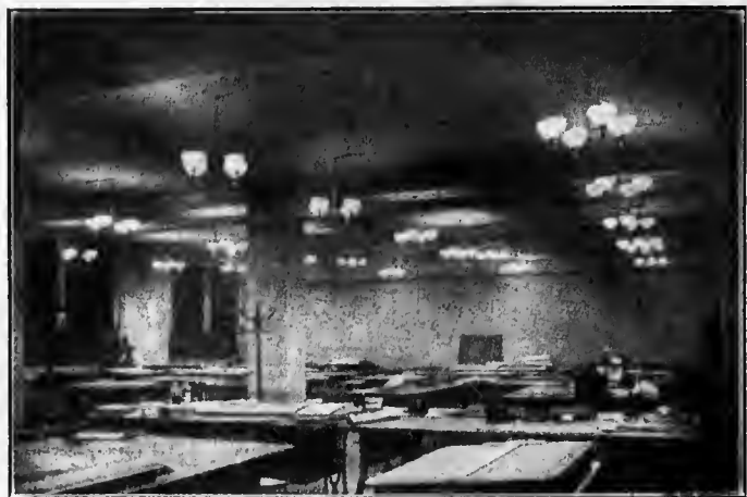
FIG. 6. VIEW OF A DRAFTING ROOM LIT WITH INVERTED TUNGSTEN LAMPS FITTED WITH DIFFUSING REFLECTORS.
