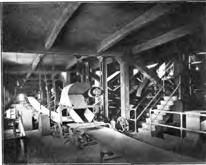
FIG. 5. BELT CONVEYORS IN SECOND STOREY OVER BINS.
