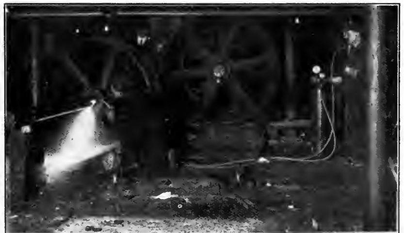
FIG. 2. CUTTING 6-INCH SHAFTS IN 6 MINUTES.
