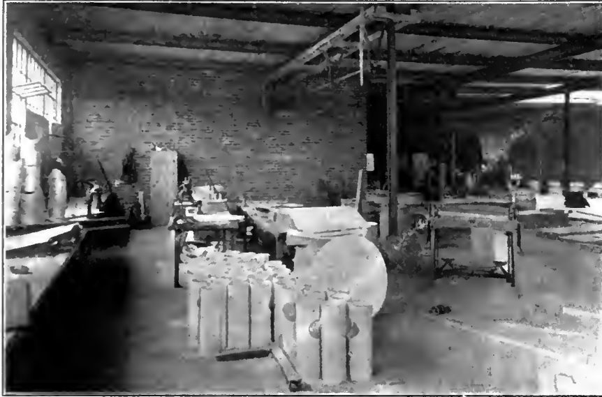
FIG. 3. PART OF MACHINE SHOP USED FOR TINSMITHING.
