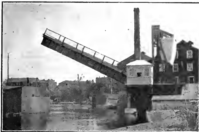
FIG. 6. ELECTRICALLY OPERATED BASCULE BRIDGE, WITH 60 FT. DECK PLATE GIRDER SPAN, OVER THE TRENT CANAL AT LINDSAY, ONT.
