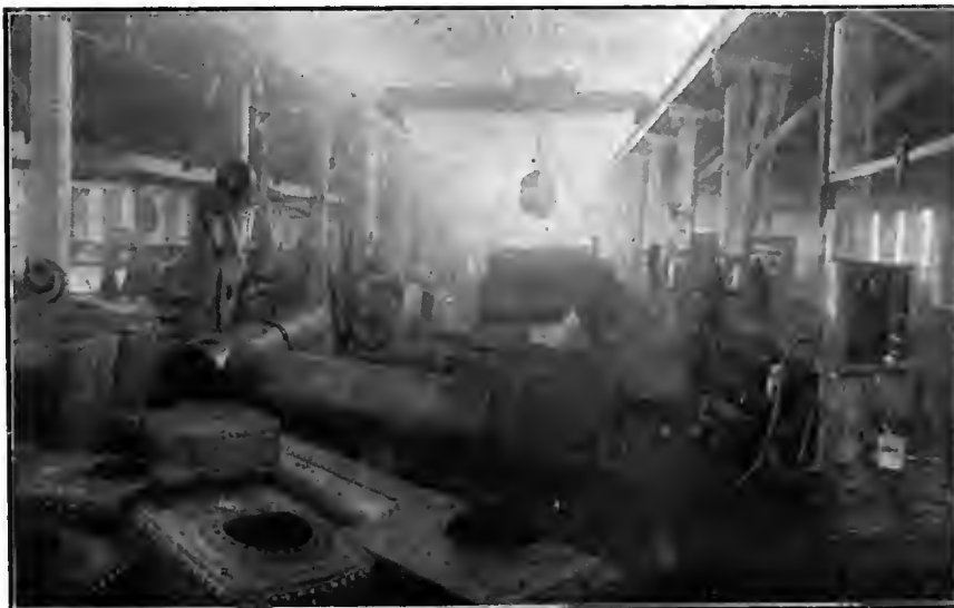
INTERIOR OF BOILER SHOP.
