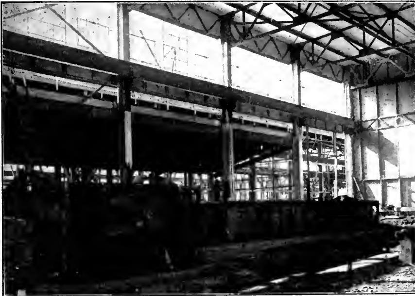
ANNEALING ROOM, SHOWING FURNACES IN COURSE OF ERECTION.
