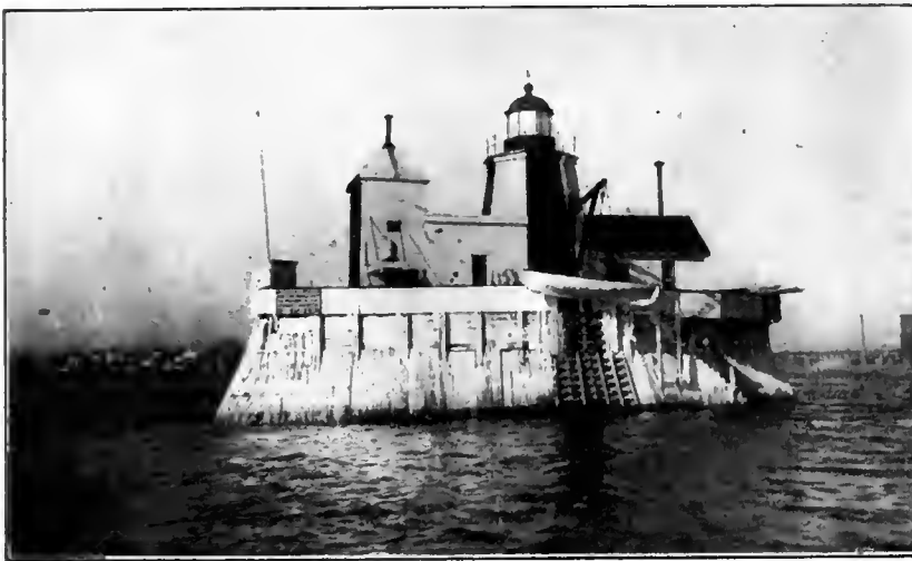
BEACON LIGHT AT HARBOR ENTRANCE, ST. JOHN, N.B.
