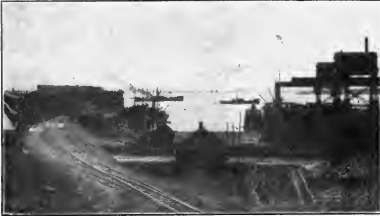
NOVA SCOTIA STEEL & COAL CO. COAL AND ORE PIERS AT NORTH SYDNEY, C.B.
