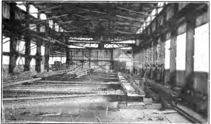
FIG. 4. GIRDER SHOP, LOOKING EAST. ON THE LEFT MAY BE SEEN THE 80 FT. OPENING FROM THE STRUCTURAL SHOP
