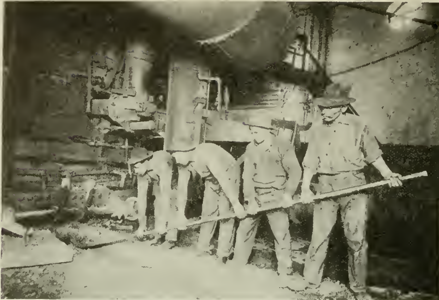
FIG. 13. UNSAFE METHOD OF DRILLING A TAPPING HOLE.
