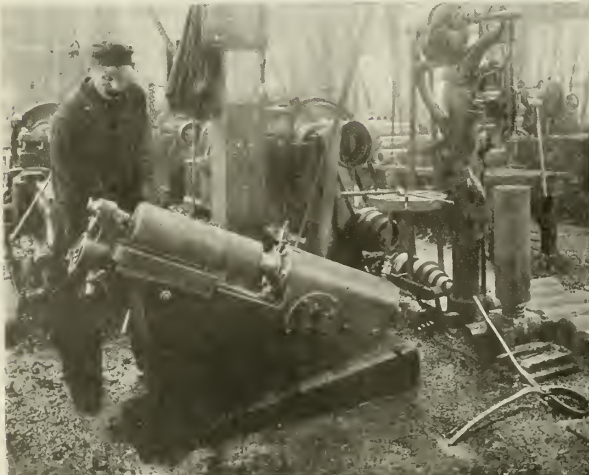
VICTORIA FOUNDRY CO. MACHINE FOR CENTERING BASE OF SHELLS.
