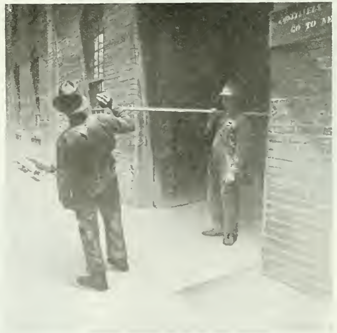
FIG. 26. SHOWING DANGER TO PASSERS-BY WHEN CARRYING BARS, PIPES AND SIMILAR MATERIAL THROUGH DOORWAYS.
