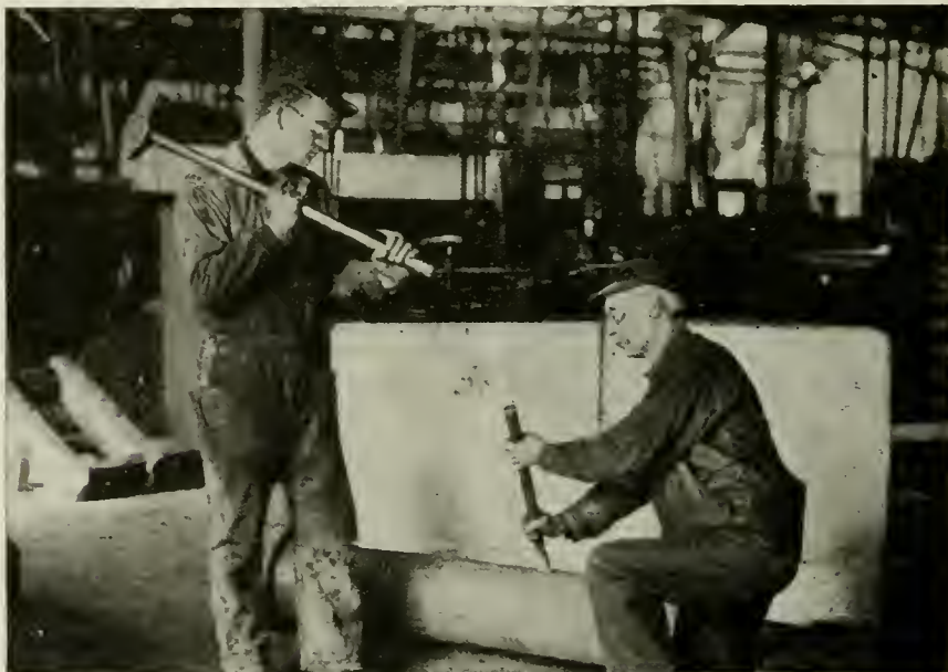
FIG. 37. WORKMEN CUTTING OUT RIVETS AND USING SHIELD. NOTE THAT GOGGLES ARE BEING WORN.
