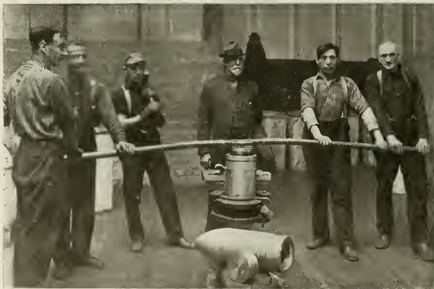
SCREWING ADAPTER IN SHELL BASE, SHOWING ALSO, IN FOREGROUND, FINISHED ADAPTER AND OPEN END OF SHELL READY TO RECEIVE IT.
