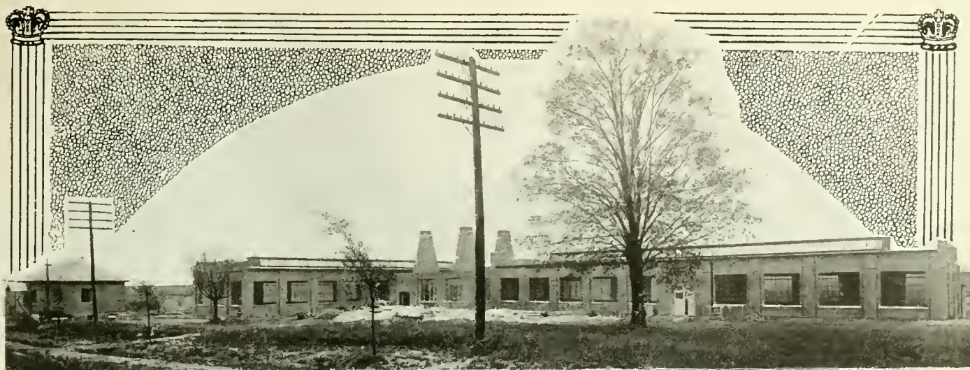
Photo shows our new plant just being completed.
