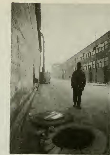
FIG. 28—WORKMAN LEAVING MANHOLE UNCOVERED
