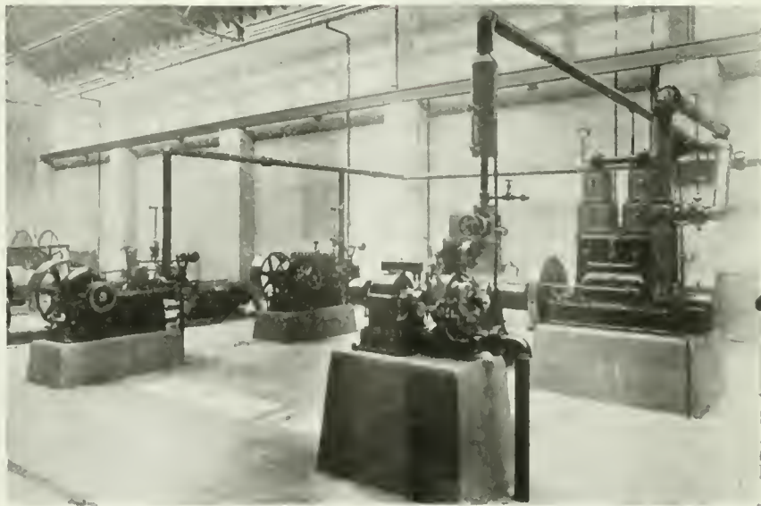
THERMODYNAMIC LABORATORY—DE LAVAL STEAM TURBINE WITH WILLIAMS VERTICAL AND LEONARD HORIZONTAL ENGINES IN BACKGROUND
