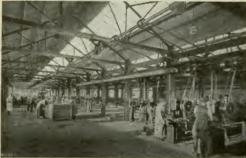
VIEW IN TOOL ROOM TEN WEEKS AFTER PLACING CONTRACT FOR ERECTION.
