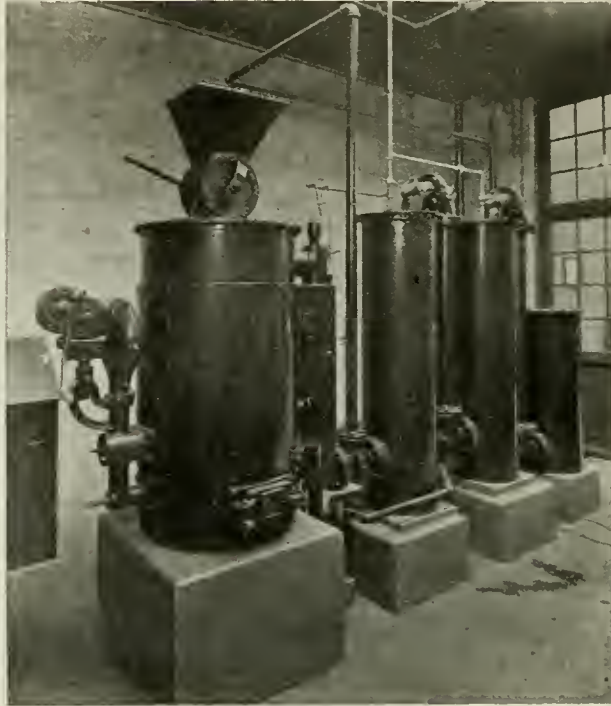
THERMODYNAMIC LABORATORY—SUCTION GAS PRODUCER PLANT.
