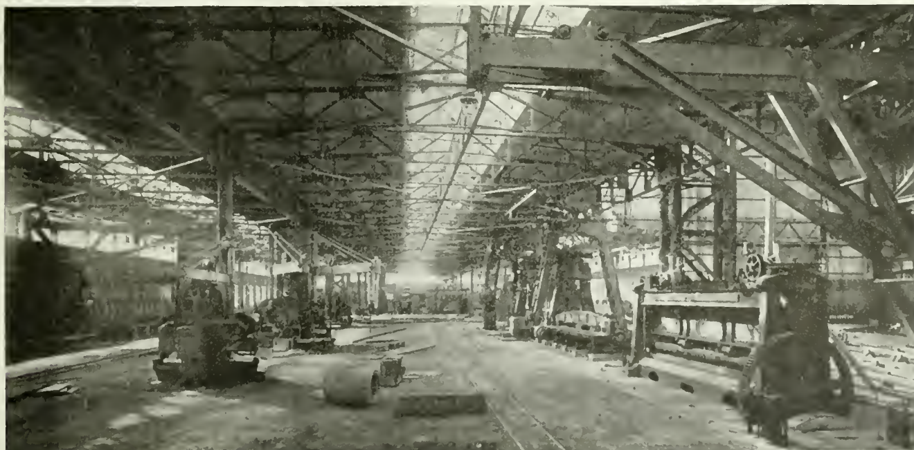
IRON WORKERS SHED, CANADIAN-VICKERS, LTD., MONTREAL.
