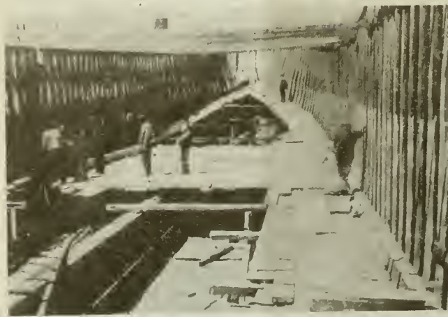
FIG. 4. STAGING FOR THE INTERIOR OF A VESSEL IN LAYING THE PLANKS, GREAT CARE MUST BE TAKEN TO SUPPORT THE ENDS SO THAT THE PLANKS WILL NOT TIP WHEN STEPPED UPON.
