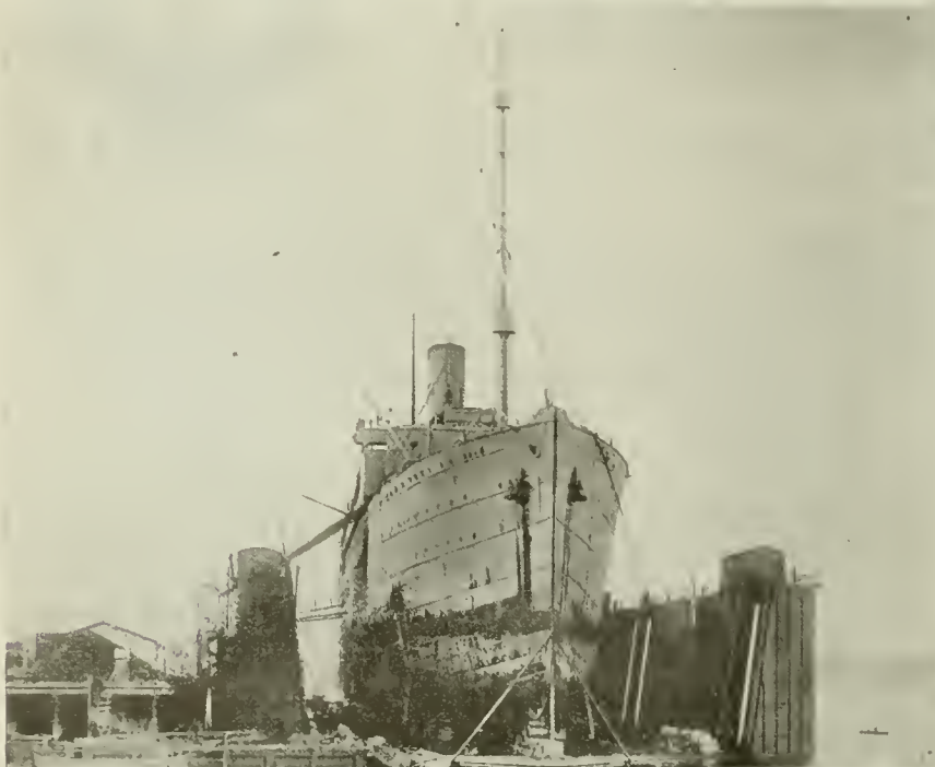
TYPICAL CANADIAN FLOATING DRY DOCK WITH VESSEL ABOARD.
