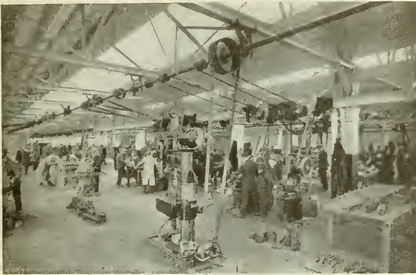
LATER VIEW IN TOOL ROOM WITH MACHINES FULLY INSTALLED.
