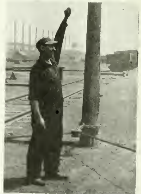
FIG. 35. CARELESS WORKMAN STANDING INSIDE OF A CABLE BENT AROUND SNATCH BLOCK.
