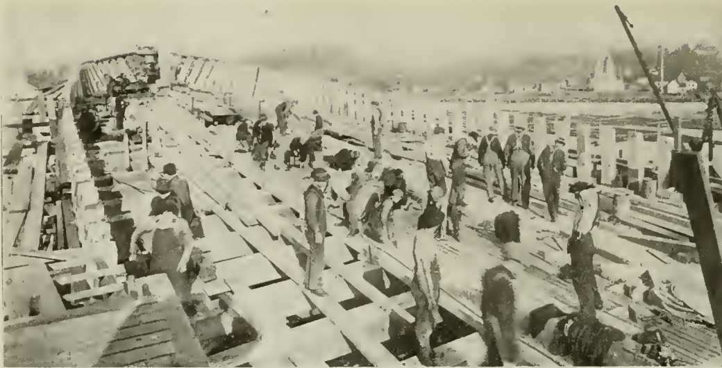
CAULKING THE MAIN DECK OF 260 FT. O.A. AUXILIARY POWERED WOOD SCHOONERS.
