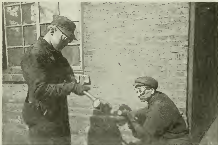
FIG. 22. SAFEST METHOD OF HOLDING A BAR.
