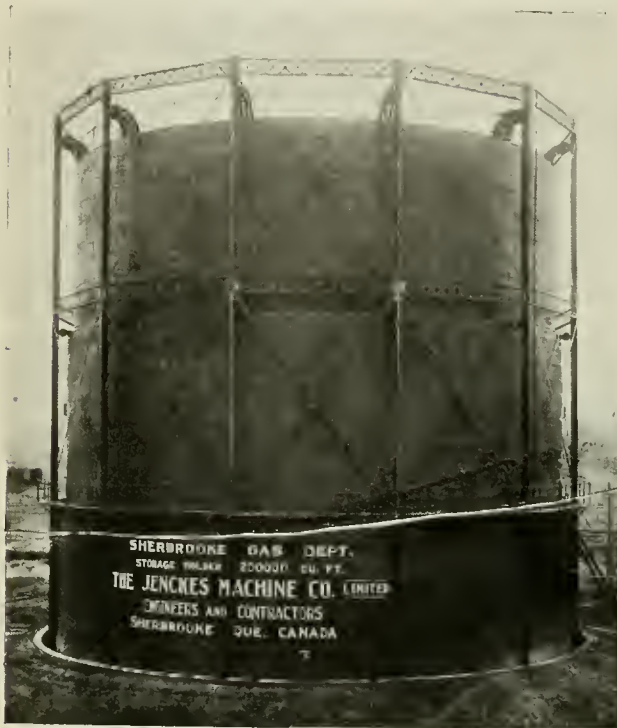
70 FT. DIA. GAS HOLDER OF 200,000 CU. FT. CAPACITY AT SHERBROOKE, QUE.
