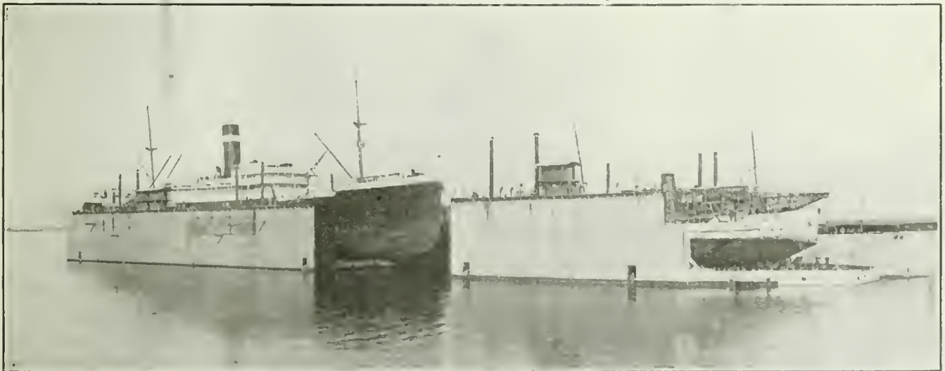
TYPICAL CANADIAN FLOATING DRYDOCK WITH TWO SECTIONS OPERATING INDEPENDENTLY.
