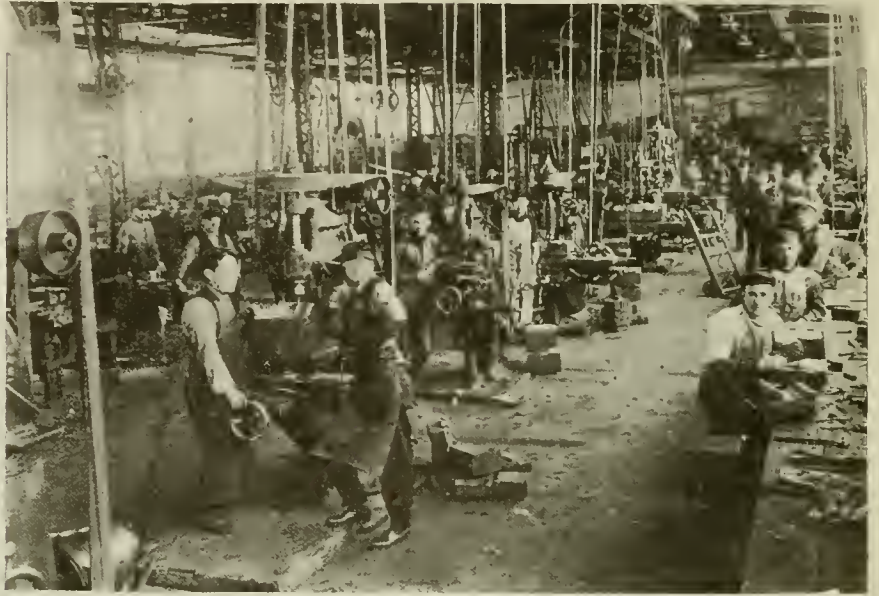
DIE-SINKING DEPARTMENT, SHOWING TYPES OF MACHINES EMPLOYED IN PRODUCING DIES FOR THE HAMMERS.
