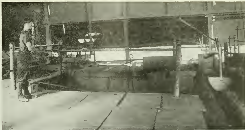
FIG. 16. MODERN RUNNER GATE OPERATED BY A CABLE AT A SAFE DISTANCE FROM THE RUNNER. ONLY A PART OF THE CABLE IS SHOWN.
