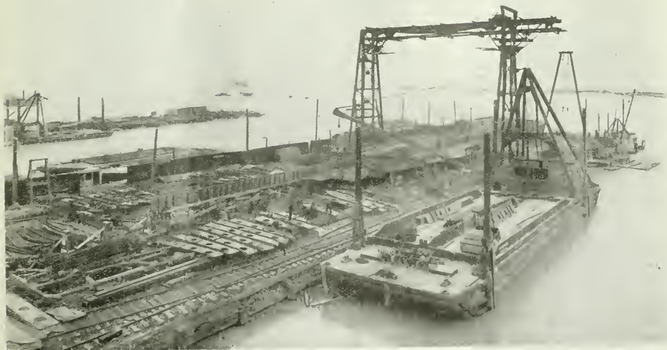
ELECTRICALLY OPERATED GANTRY AND SHIPBUILDING BERTH AT THOR IRON WORKS, TORONTO.
