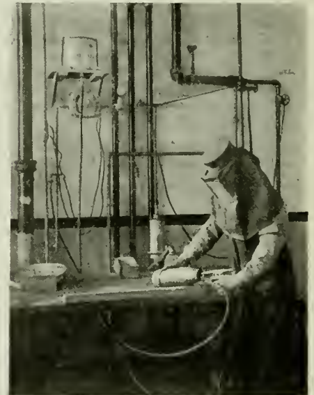
FIG. 13. PAASCHE AIR BRUSH EQUIPMENT FOR VARNISHING THE INTERIOR OF THE SHELLS.
