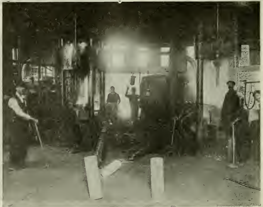
TWO 500-TON PRESSES FORGING 6 INS. SHELL. CONTINUOUS FURNACE IN REAR, AND GRAVITY CARRIERS ALONGSIDE EACH PRESS.
