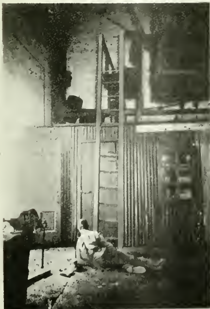
FIG. 9—MAN FALLS FROM LADDER
