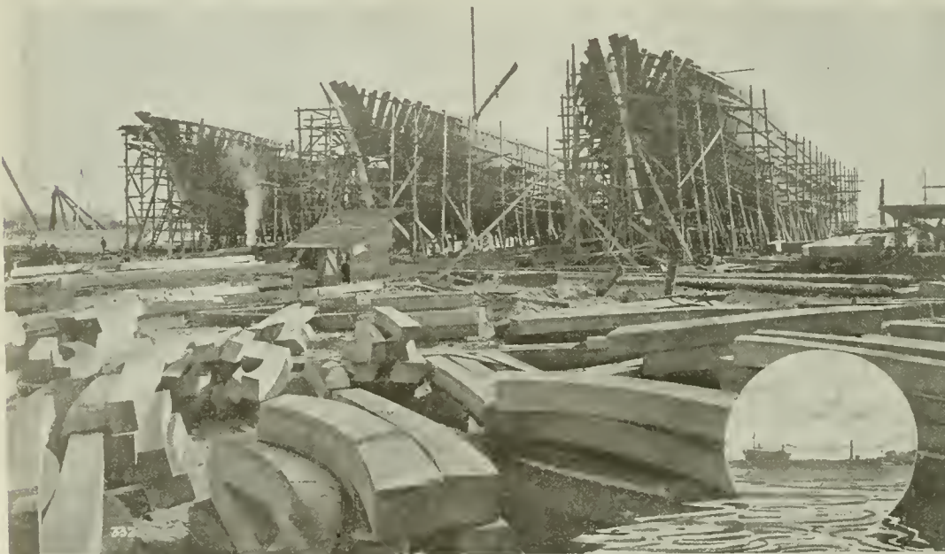
AUXILIARY POWERED SCHOONERS OF WOOD, 260 FT. OVER-ALL LENGTH, BUILDING AT NORTH VANCOUVER, B.C.
