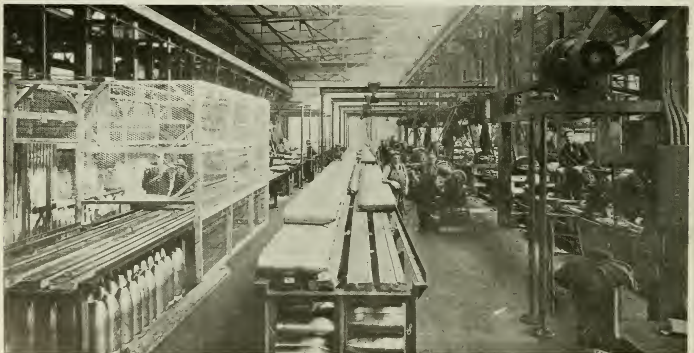
FIG. 12. VIEW OF BAY SHOWING TRACKS FOR WORK AND PRELIMINARY INSPECTION CRIB.
