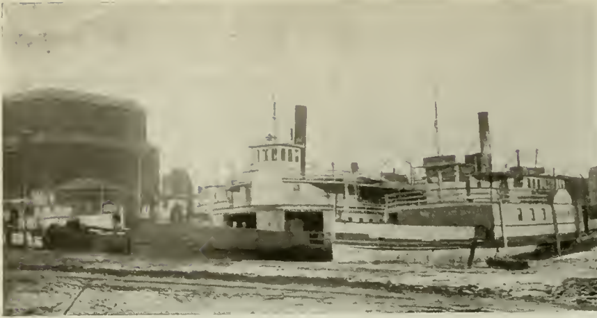
GENERAL VIEW OF PLANT OF THE MONTREAL DRYDOCK CO.
