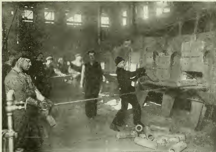
FURNACES USED FOR ANNEALING FORGINGS THAT REQUIRE HEAT TREATMENT.
