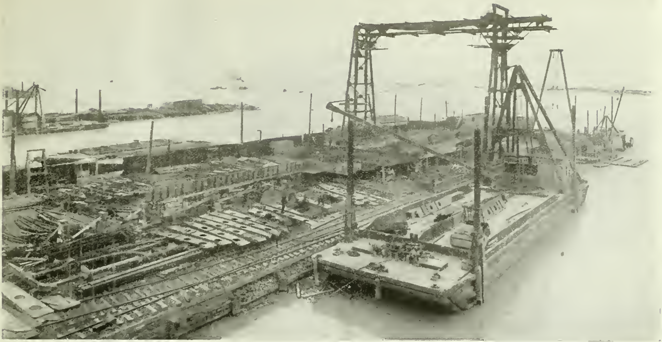
ELECTRICALLY OPERATED GANTRY AND SHIPBUILDING BERTH AT THIOR IRON WORKS, TORONTO.
