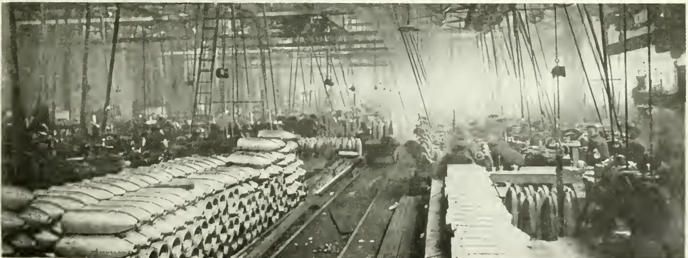
GENERAL VIEW OF SHOP LAYOUT FOR MACHINING THE 9.2 INCH HIGH EXPLOSIVE SHELL.
