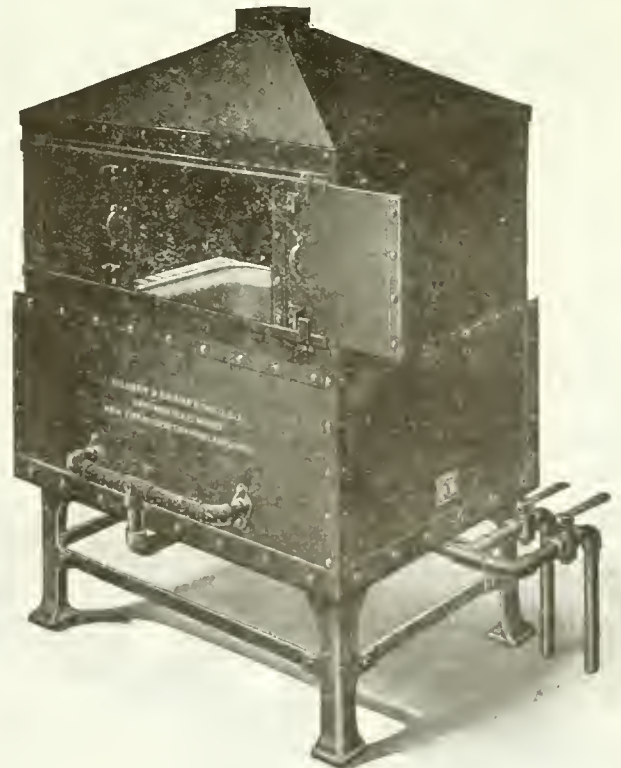
TYPE F-4 FURNACE WITH HOOD
