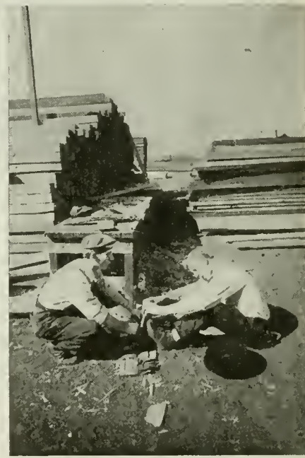
FIG. 39. RESULT OF LEAVING BOARD LYING ABOUT WITH NAILS IN IT.
