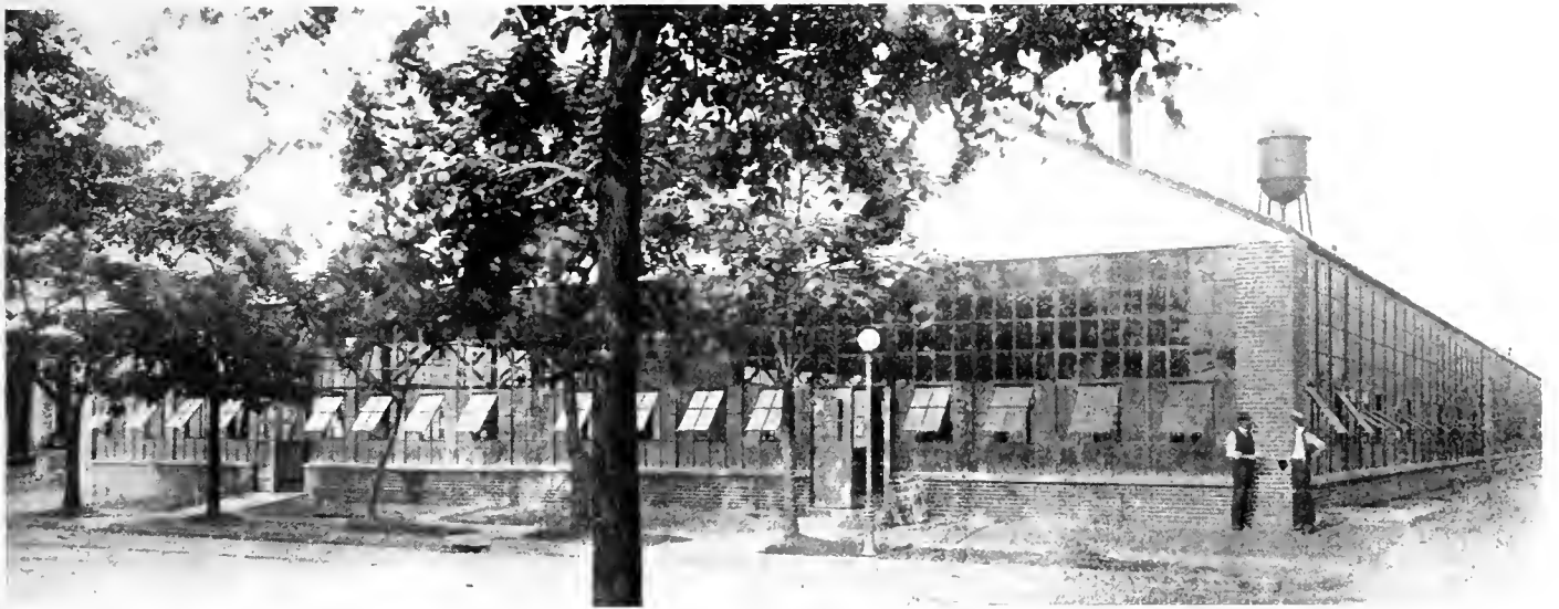
EXTERIOR OF BUILDING, SHOWING GLASS WALL CONSTRUCTION WHICH INSURES MAXIMUM LIGHT AND VENTILATION.
