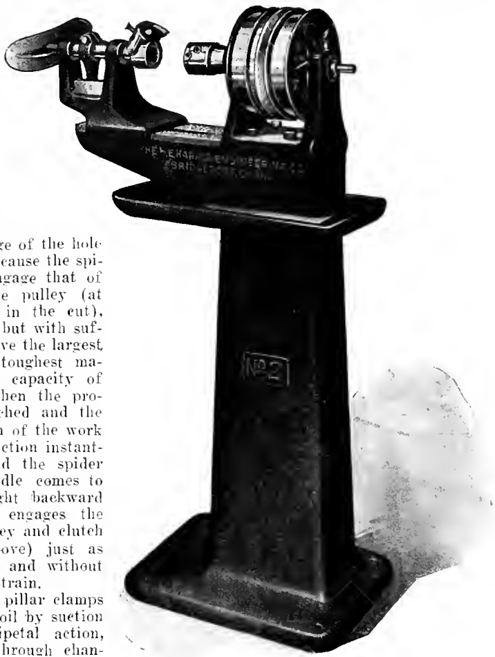
VIEW OF TAPPING MACHINE SHOWING BREAST OPERATED WORK HOLDER.
