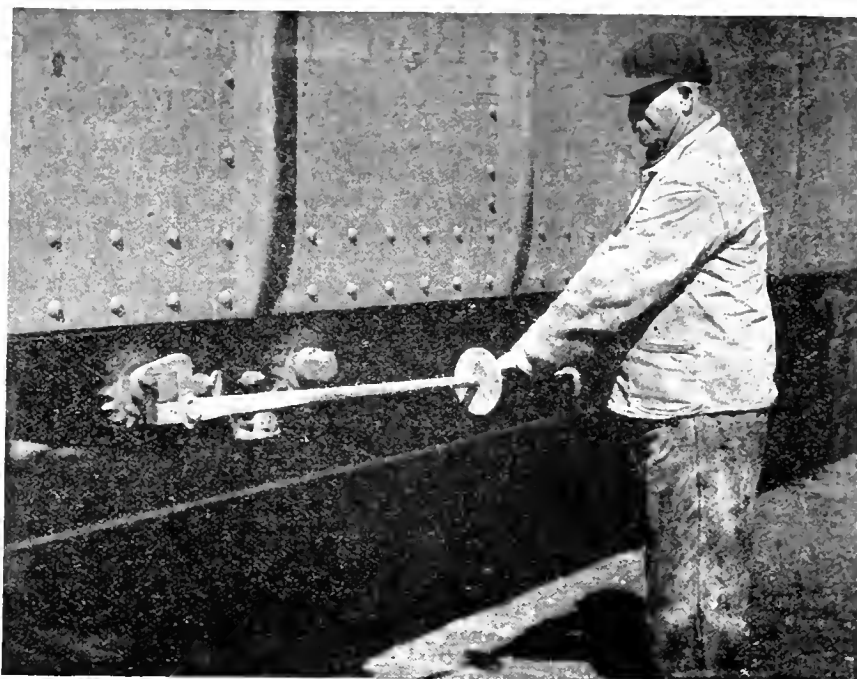
FIG. 22. TRESTLE LABORER USING SAFETY CAR WRENCH. WHEN THE SHAFT BEGINS TO REVOLVE, THE HINGED JAW RELEASES. DISC IS TO PREVENT MAN'S HAND STRIKING CAR, AND SHORT BEND ON END OF HANDLE PREVENTS USE OF PIPE EXTENSION.
