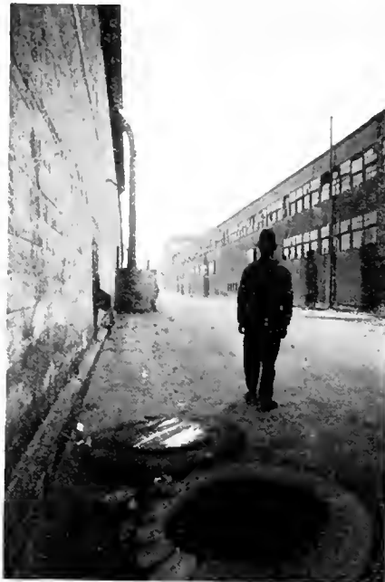
FIG. 28. WORKMAN LEAVING MANHOLE UNCOVERED
