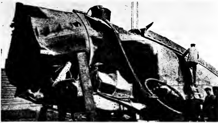
SHOWING EFFECT OF EXPLOSION ON MIDSHIPS SECTION OF HULL.
