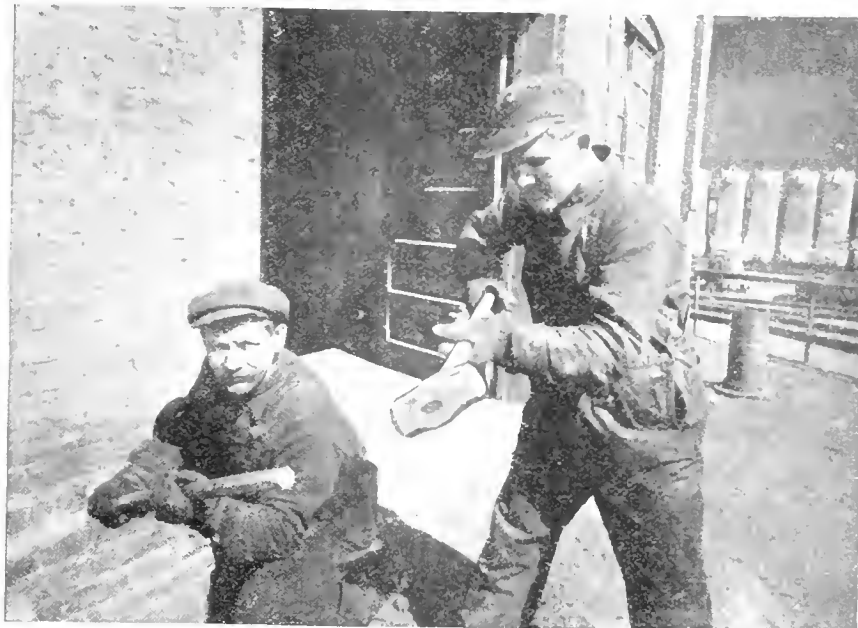
FIG. 31. UNSAFE WAY OF HOLDING BAR FOR A SLEDGE. MAN HOLDING BAR IS STANDING ON SAME SIDE AS STRIKER.
