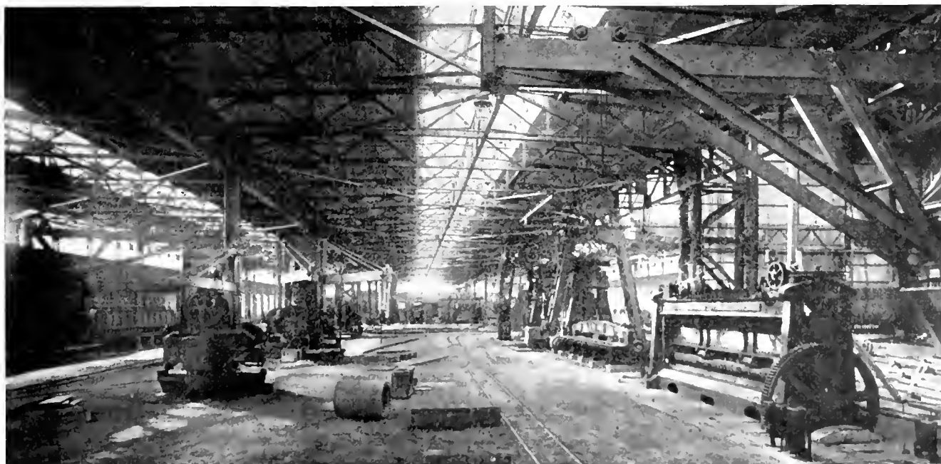
IRON WORKERS SHED, CANADIAN VICKERS, LTD., MONTREAL.
