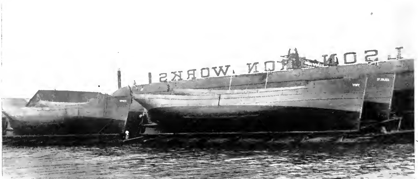
SHOWING THE FOUR VESSELS ON THE WAYS PREVIOUS TO LAUNCHING.
