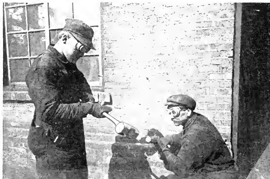
FIG. 22. SAFEST METHOD OF HOLDING A BAR.
