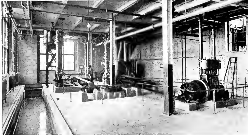
HYDRAULIC LABORATORY ESCHER, WYSS AND GWYNNE PUMPS DRIVEN BY BELLIS & MORCOM ENGINE.
