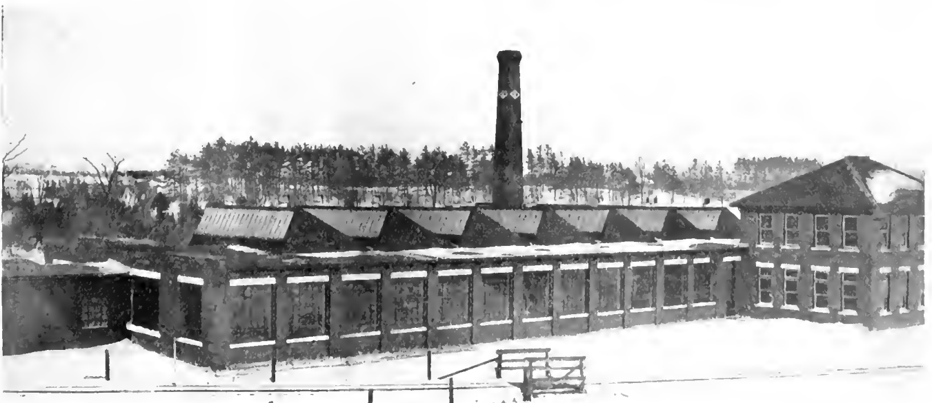
FIG. 1. EXTERIOR OF FACTORY SHOWING SAW-TOOTH ROOF, EXTENSIVE SIDELIGHT PROVISION, AND OFFICE BUILDING.
