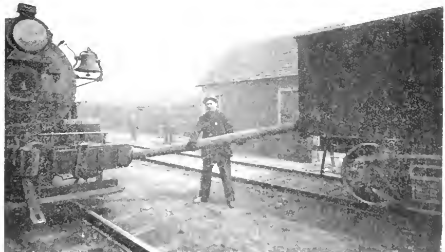
FIG. 21. SAFEST WAY OF USING POLE TO PLACE CARS
