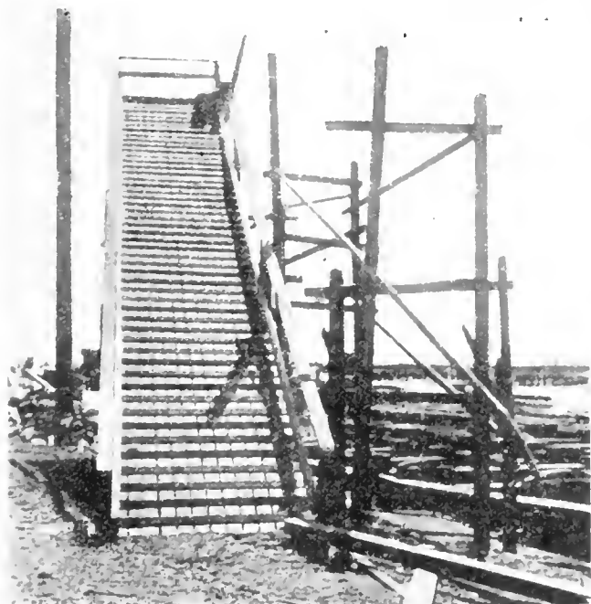
FIG. 6. WELL CONSTRUCTED MAIN APPROACH, WHICH IS A PERMANENT STRUCTURE, GIVING DIRECT ACCESS TO THE UPPER DECK OF A SHIP ON THE STOCKS.
