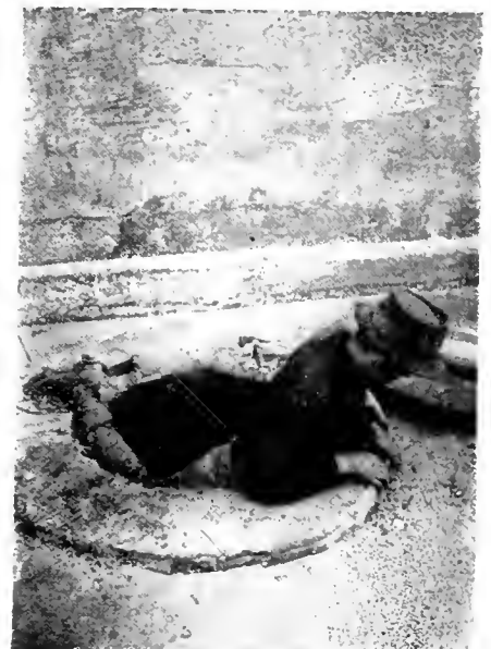
FIG. 29.—PASSER-BY FALLS IN MANHOLE LEFT OPEN BY OPERATOR
