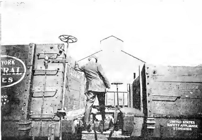
FIG. 3—A DANGEROUS PRACTICE, CLIMBING BETWEEN CARS
