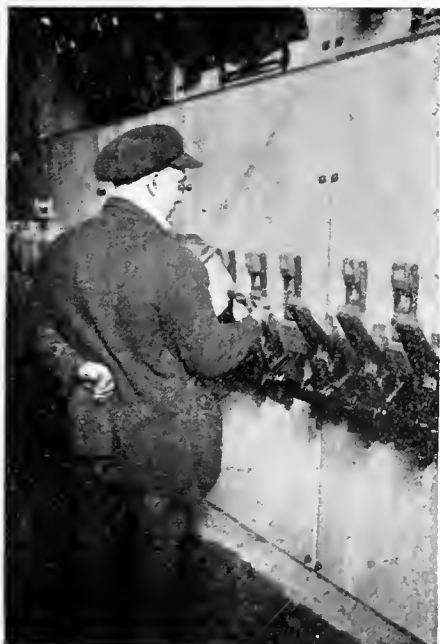
FIG. 40. SAFE WAY TO OPEN A SWITCH. USE ONE HAND AND KEEP OTHER BEHIND BACK.
