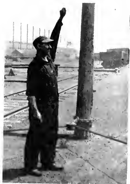
FIG. 35. CARELESS WORKMAN STANDING INSIDE OF A CABLE BENT AROUND SNATCH BLOCK.
