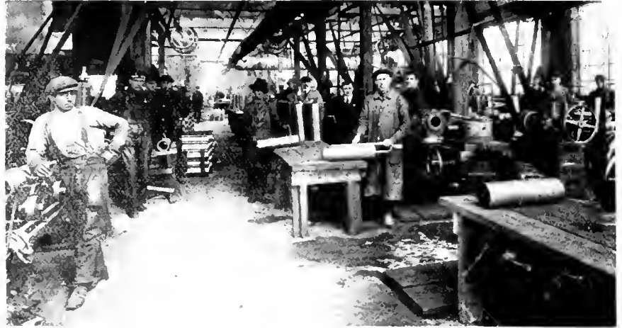
GENERAL VIEW OF SECTION OF SHELL SHOP.
