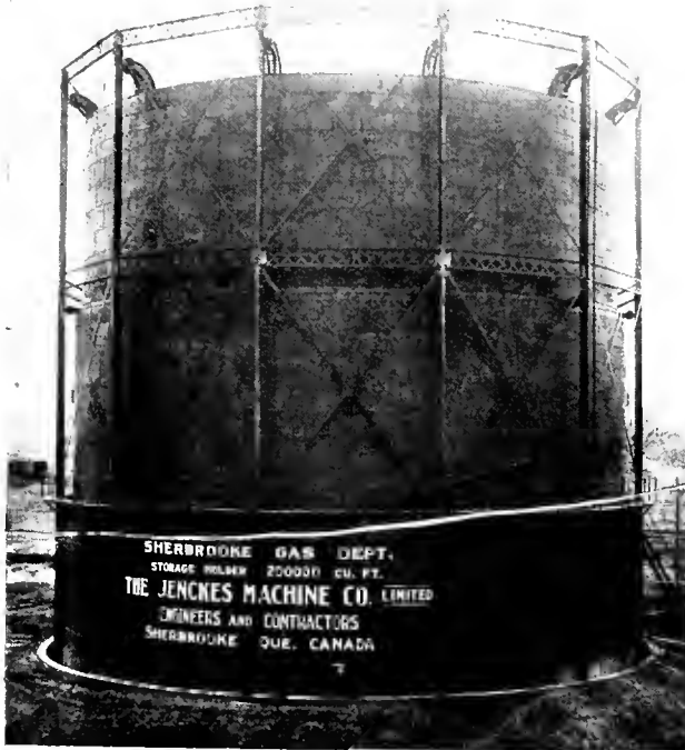
70 FT DIA GAS HOLDER OF 200,000 CU. FT. CAPACITY AT SHERBROOKE, QUE.
