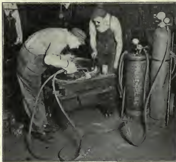
PREST-O-LITE EQUIPMENT BEING USED IN WELDING OPERATION.
