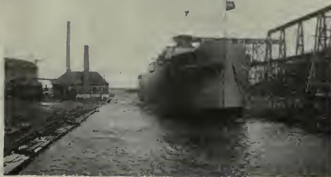
3,500-TON STEEL SHIP AFTER LAUNCHING
