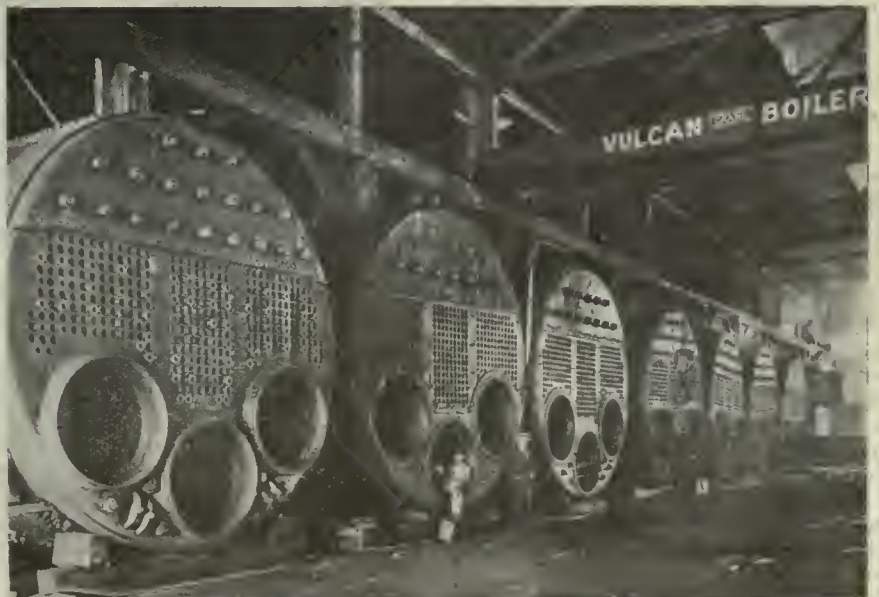
FIG. 4—VULCAN IRON WORKS BOILER SHOP
