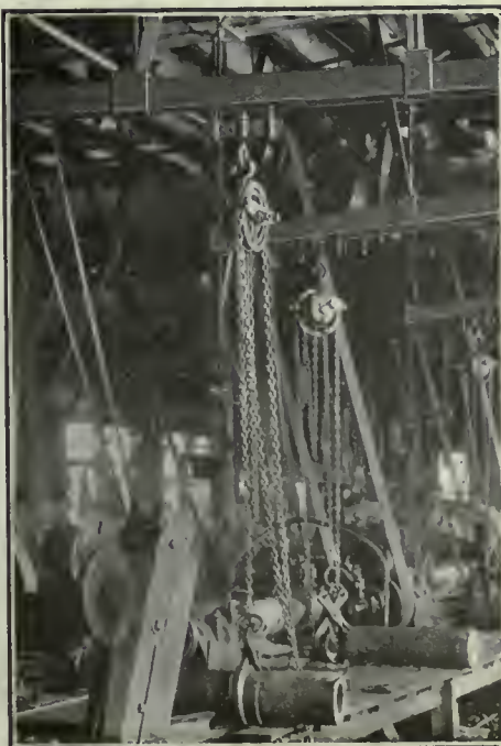
DETAIL VIEW OF CHAIN BLOCKS AND CARRIERS.
