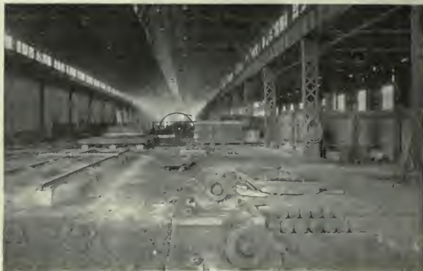
VIEW FROM ONE END OF THE MILL SHOWING ANNEALING FURNACES, ANNEALING BOXES ON THE RIGHT AND COOLING FLOOR ON THE LEFT. MILL TRAIN DRIVE IN BACKGROUND.
