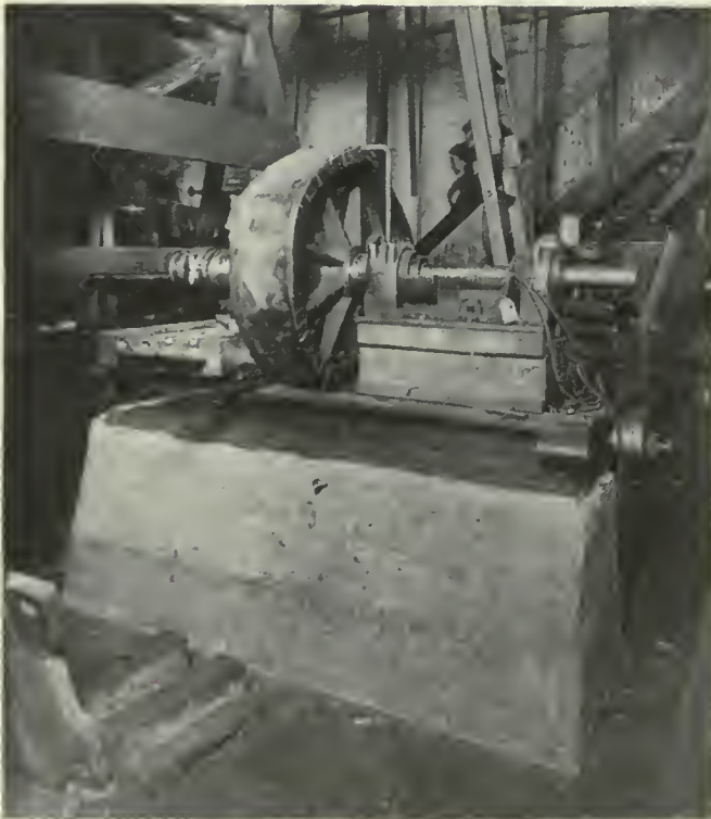
CONCRETE BASE CAST AROUND BASE OF GRINDING TOOL TO GET RIGIDITY
