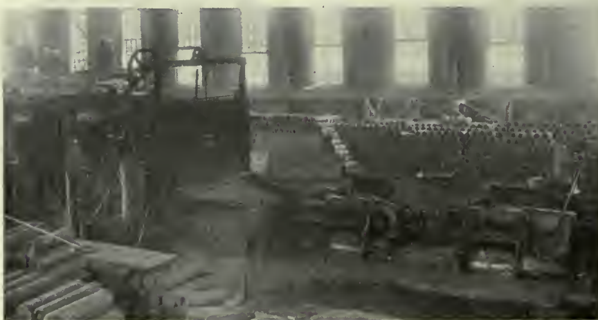
FURNACE USED FOR HEAT TREATMENT OF FORGINGS SHOWING AIR COOLING APPARATUS IN PLACE.
