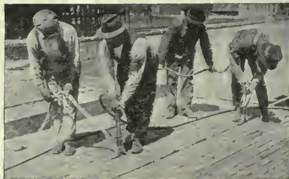
CAULKING DECK PLANKING
