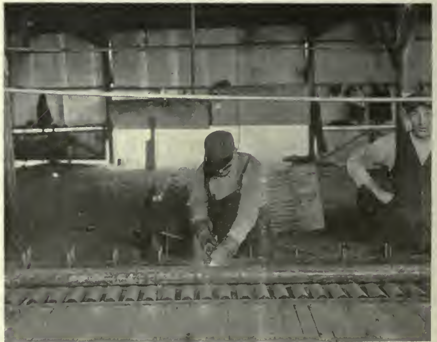
SPACING MACHINE DESIGNED BY MR. BECK.
