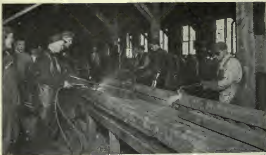
NICKING THE GOTHIC STEEL BY THE OXY-ACETYLENE TORCH.
