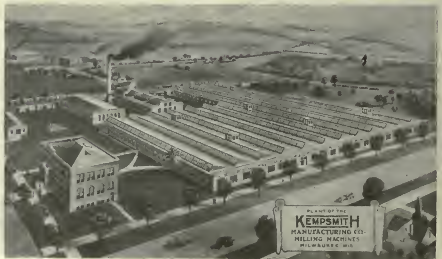
PLANT OF THE KEMPSMITH MANUFACTURING CO., MILWAUKEE.
