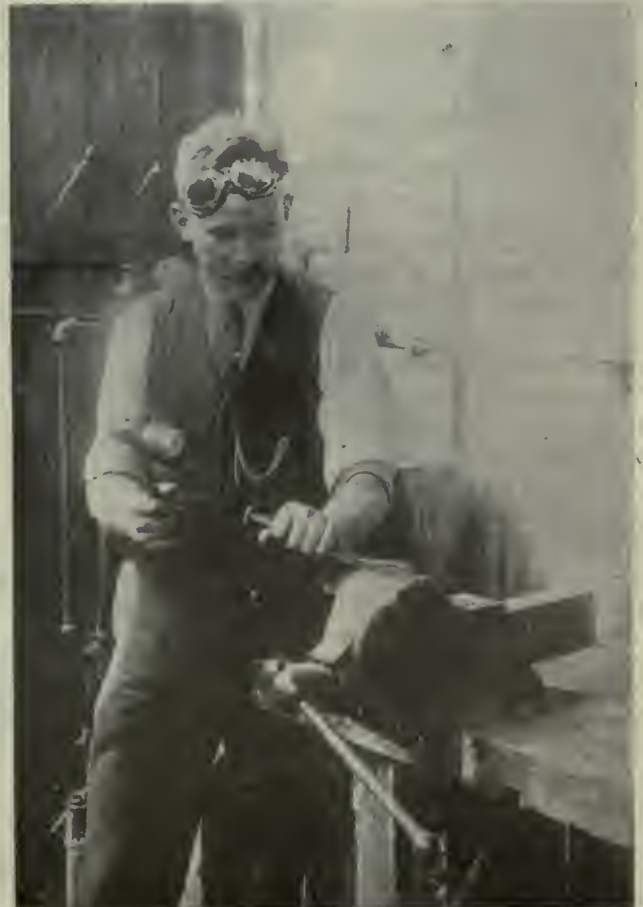
CHIPPING PLATE AFTER CUTTING FOR WELDING
