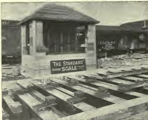
FIG. 1 WEIGH BEAM OF 150 TON TRACK SCALE
