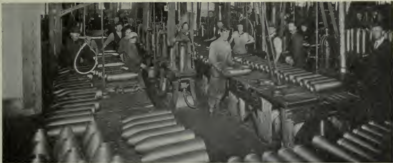
MACHINES FOR SANDBLASTING BASE OF 6-INCH SHELL
