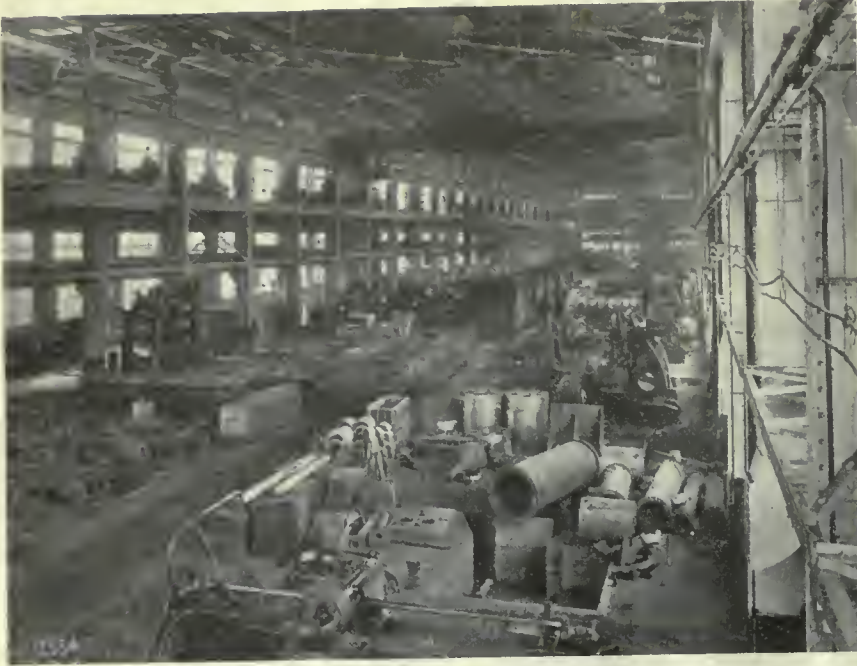
WESTINGHOUSE ERECTING SHOP.
