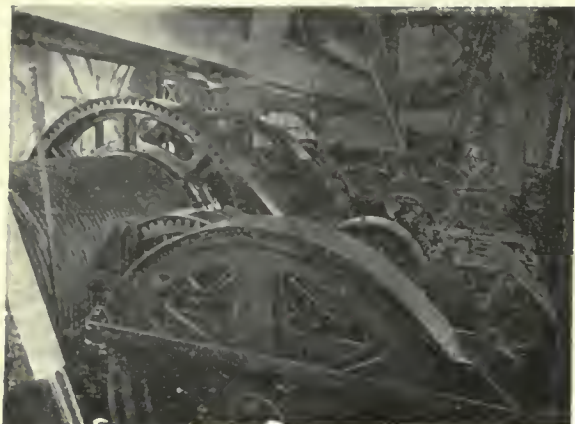
60 H.P. motors and hoist drums.
