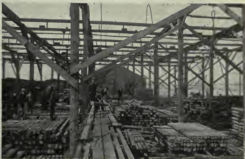
GOTHIC STEEL, METHOD OF HANDLING THE BARS PREPARATORY TO NICKING.
