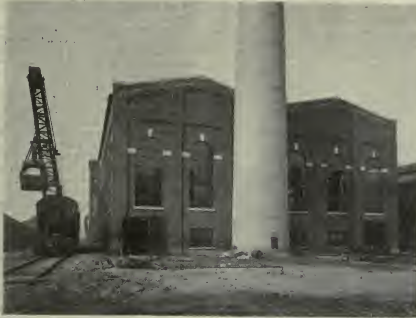
EXTERIOR OF POWER HOUSE
