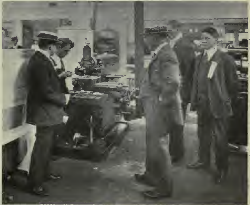
VARIOUS WELDING OPERATIONS BY THE OXY-ACETYLENE TORCH IN L'AIR LIQUIDE SOCIETY PORTION OF THE EXHIBIT OF THE DEPARTMENT OF THE SOLDIERS' CIVIL RE-ESTABLISHMENT.
