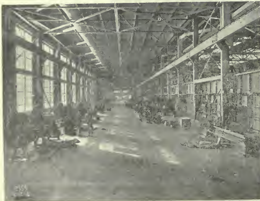
INTERIOR VIEW OF MACHINE SHOP.
