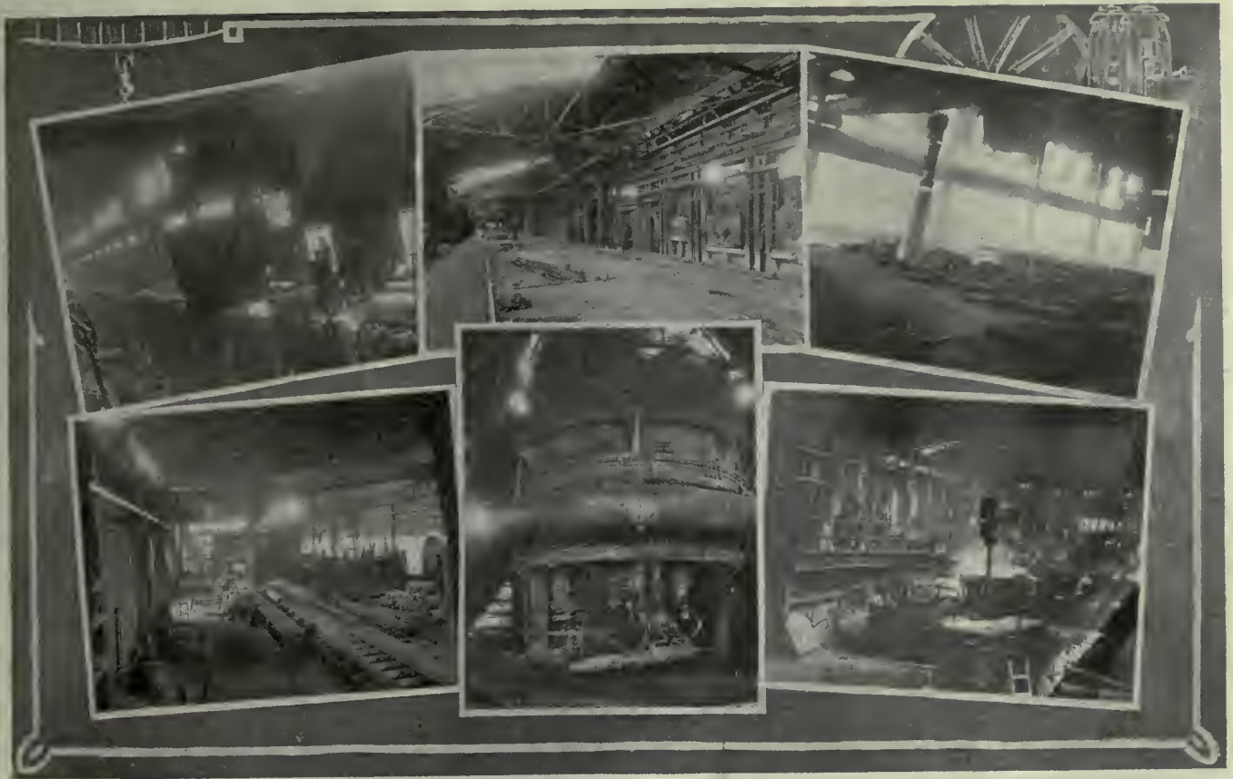
TOP LEFT TO RIGHT: CASTING STEEL INGOTS. CHARGING FLOOR OPEN HEARTH FURNACES. REMOVING HOT INGOT FROM SOAKING PIT. BOTTOM LEFT TO RIGHT: INTERIOR VIEW OF BLOOMING MILL. BOTTOM OF BLAST FURNACE. CASTING PIT OPEN HEARTH FURNACE PLANT.
