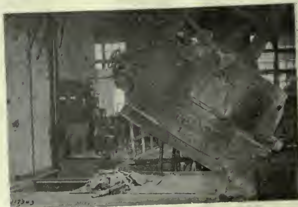
FURNACE IN TILTED POSITION
