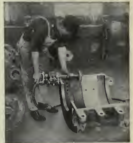
THE PNEUMATIC TOOL IN OPERATION.
