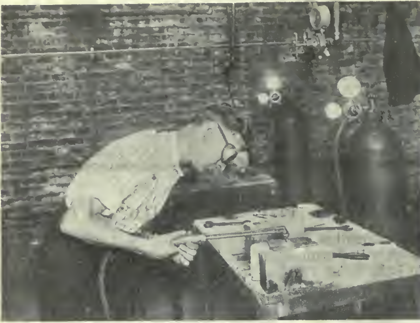
RECEIVING TRAINING IN THE USE OF OXY-ACETYLENE WELDING APPARATUS.
