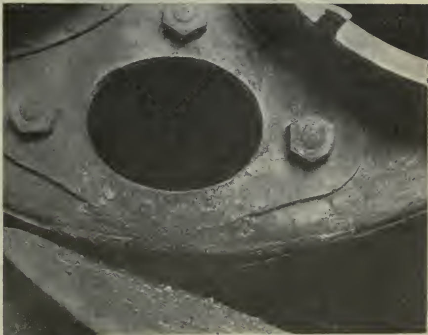
WELDING REPAIR TO MARINE BOILER
