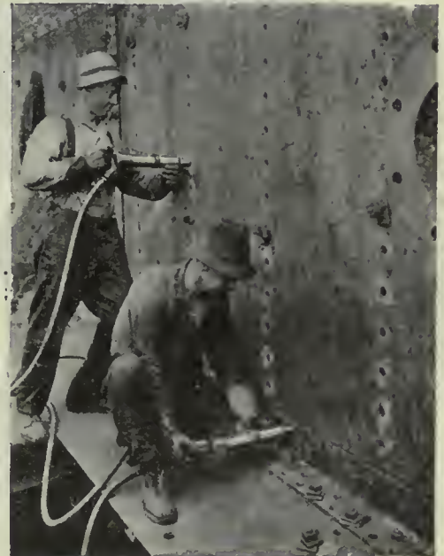
No. 60 One-Piece Long Stroke Hammer driving 3/8-inch flush rivets in Engine Room Bulkheads.
