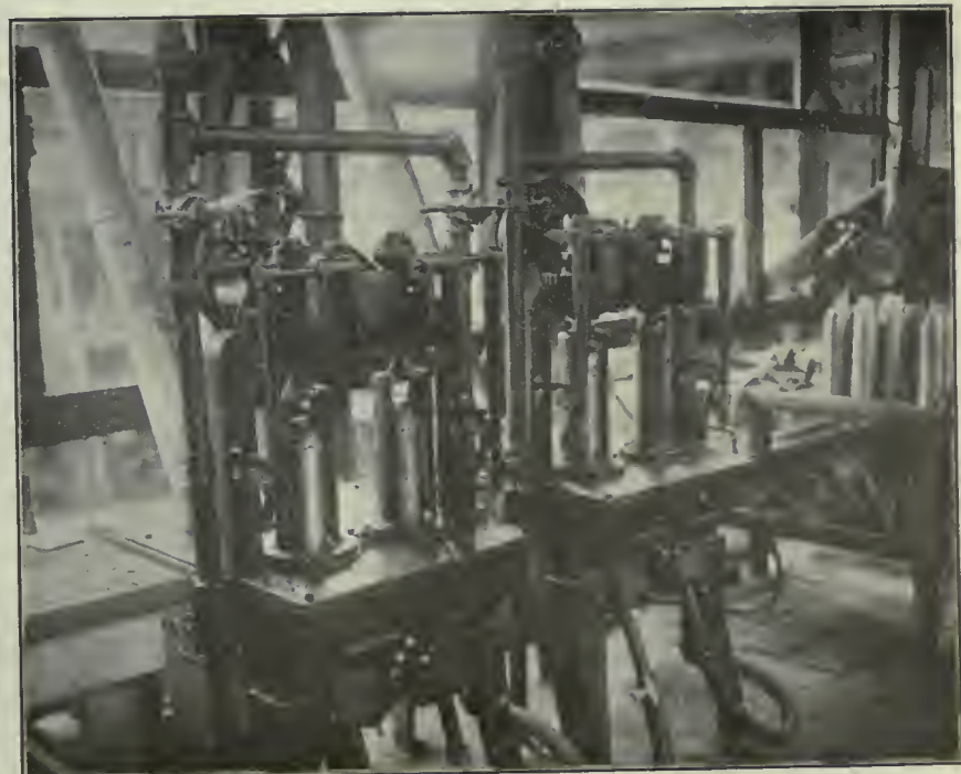
SAND BLASTING BORE OF SHELL.
