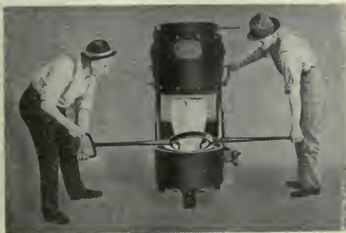
FURNACE OPEN FOR REMOVAL OF CRUCIBLE.
