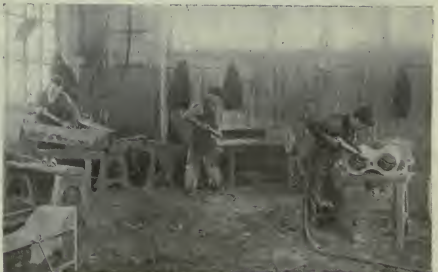
FIG. 1—PNEUMATIC HAMMERS AT WORK IN AN ENGLISH SHOP.
