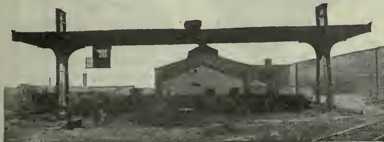
Electric Traveling Gantry Crane with Magnet
