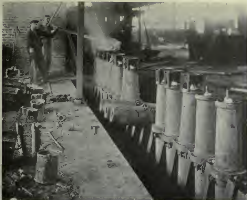
CASTING BRASS TUBES IN CAST-HOUSE OF DOMINION COPPER PRODUCTS CO.
