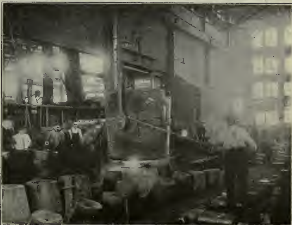
TEEMING TYRE INGOT FROM LADLE INTO INGOT MOULDS
