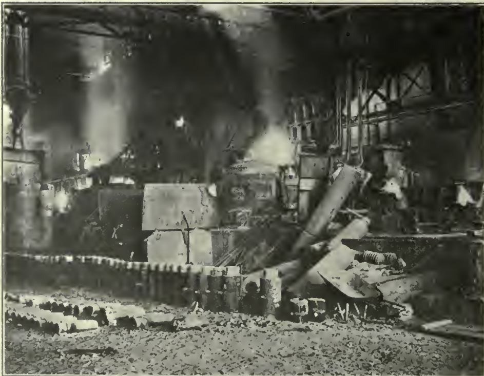
BATTERY OF SIX-TON HEROUULT FURNACES
