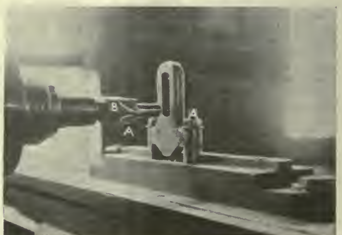
FIG. 4—MILLING THE SLOT
