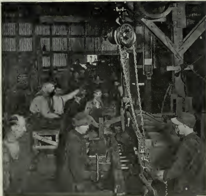
AFTER THE GOTHIC BARS ARE NICKED BY THE OXY-ACETYLENE TORCH THEY ARE CONVEYED TO THE BULLDOZER SHOWN AND BROKEN INTO BILLETS OF THE PROPER LENGTH.
