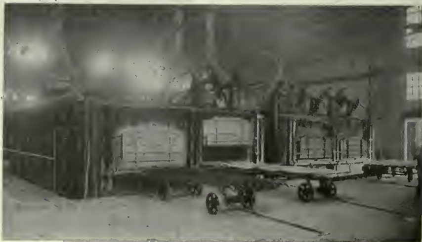
ANNEALING FURNACES IN PLANT OF DOMINION COPPER PRODUCTS CO.
