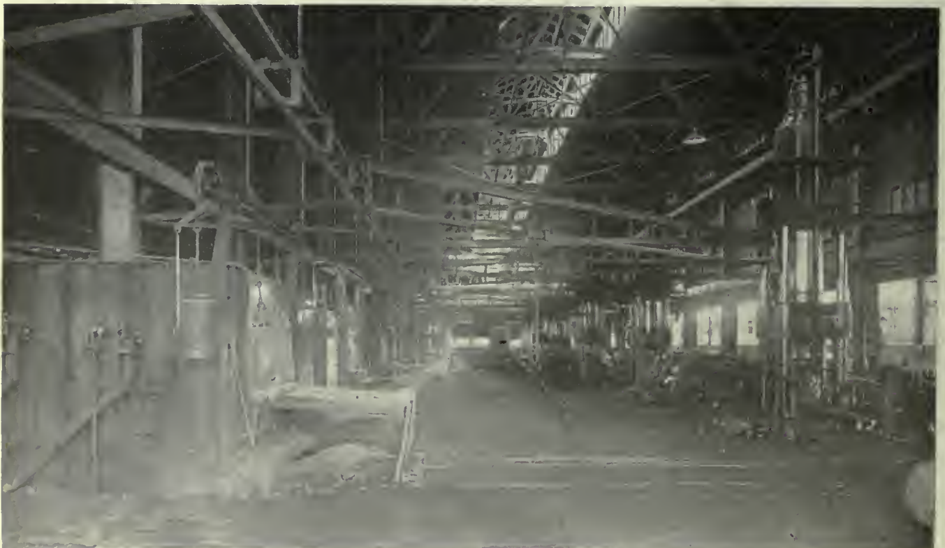
FORGE SHOP—FURNACES AND HYDRAULIC PRESSES.
