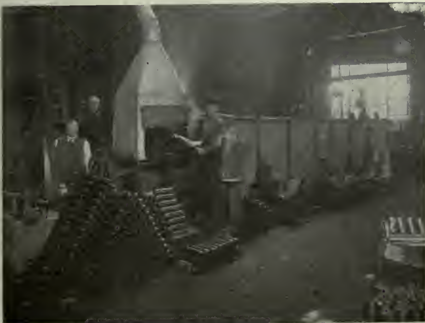
CONTINUOUS FURNACE FOR HEAT TREATING 75-MM. SHELLS.
