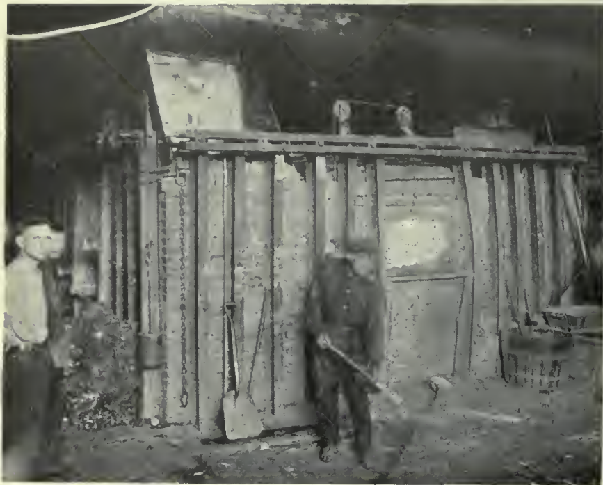
BACK VIEW OF THE 15-TON FURNACE SHOWING CHARGING FLOOR.
