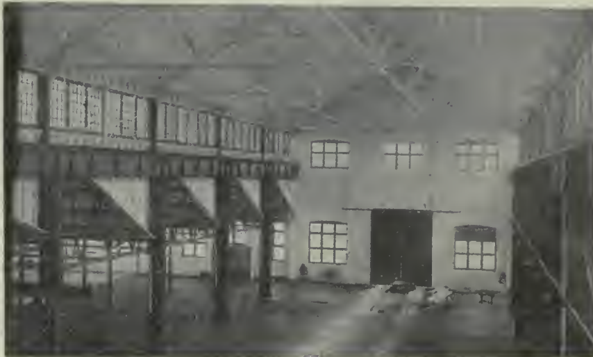
INTERIOR VIEW OF NEW SHOP AT THE CANADA MACHINERY CORPORATION.
