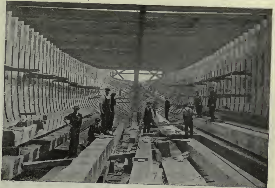
FIG. 7—HULL OF THE MARGARET HANEY, AUXILIARY POWER SCHOONER, UNDER CONSTRUCTION
