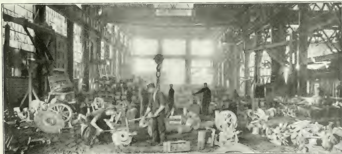
FIG. 1. GENERAL VIEW OF FETTLING SHOP FLOOR
