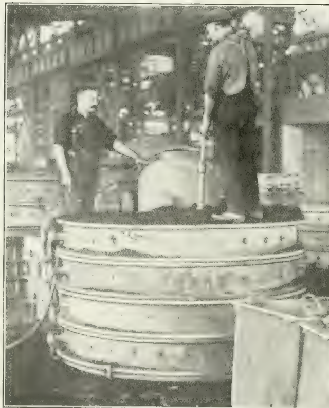
FIG. 11. PREPARING MOLD FOR LARGE STEEL HYDRAULIC CYLINDER.
