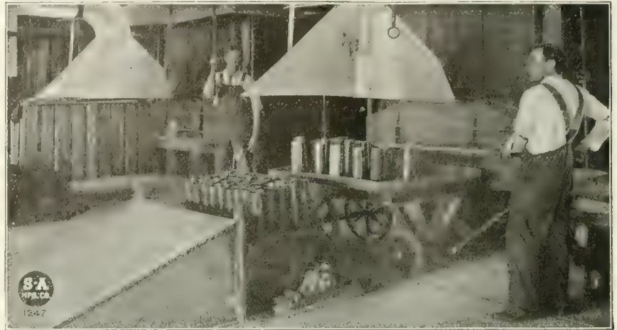
FIG. 1. CARTRIDGE CASES BEING PICKED OFF PAN FROM ANNEALING FURNACE AND LOADED INTO WIRE BASKET ON CONVEYOR.
