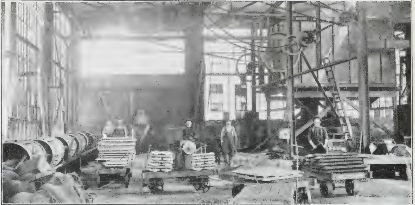
FIG. 5. GENERAL VIEW OF FETTLING SHOP.
