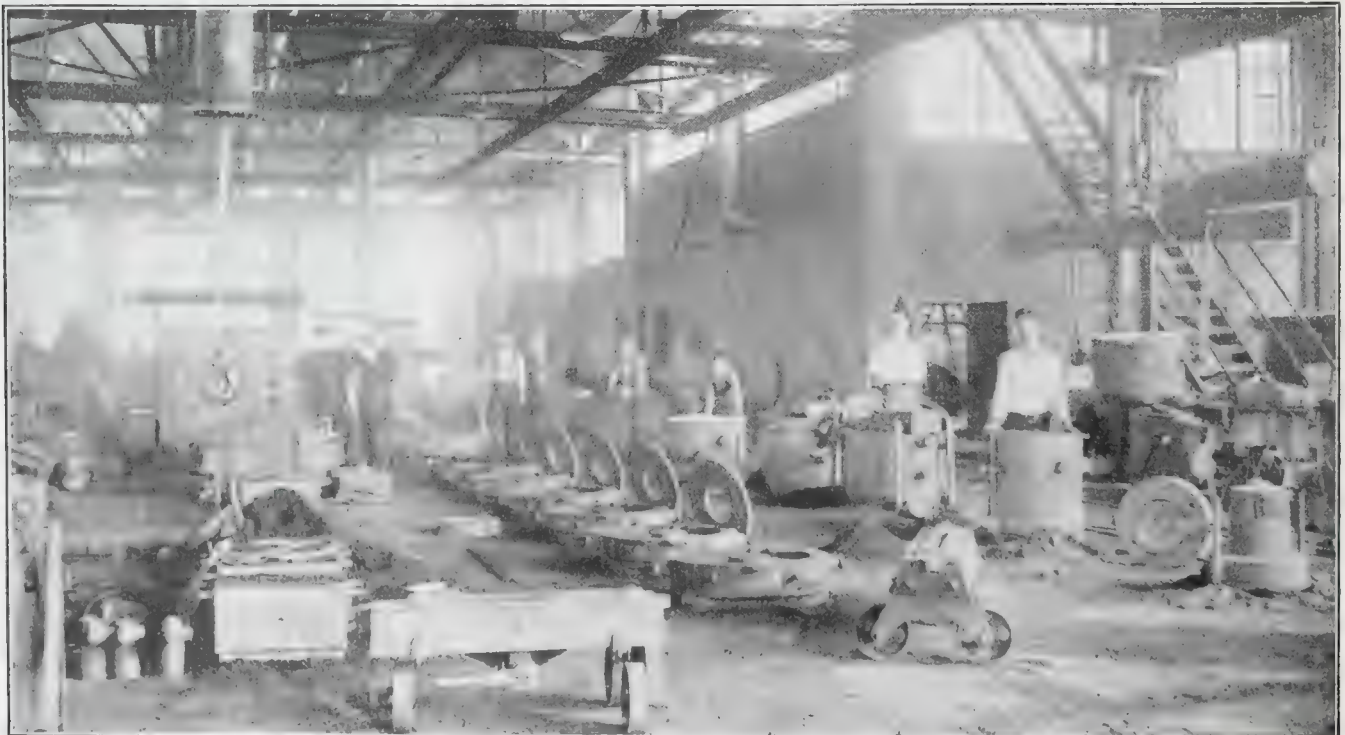
FIG. 4. HEATING BOILER MOLDING SHOP.
