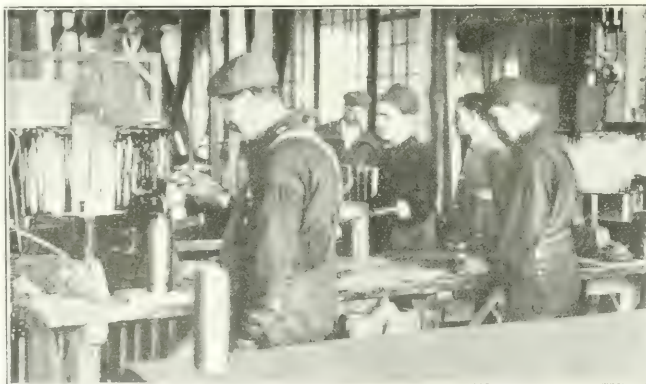
FIG. 11 FILLING SHELLS WITH RESIN. TANKS HEATED BY ELECTRICITY
