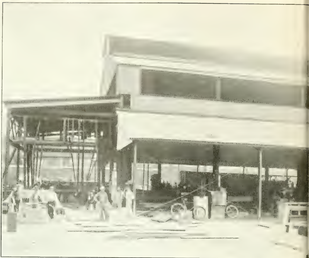
FORGING SHOP ERECTED FOR PRODUCING
