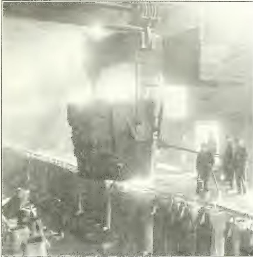
"TEEMING" THE MOLTEN STEEL INTO INGOT MOLDS.
