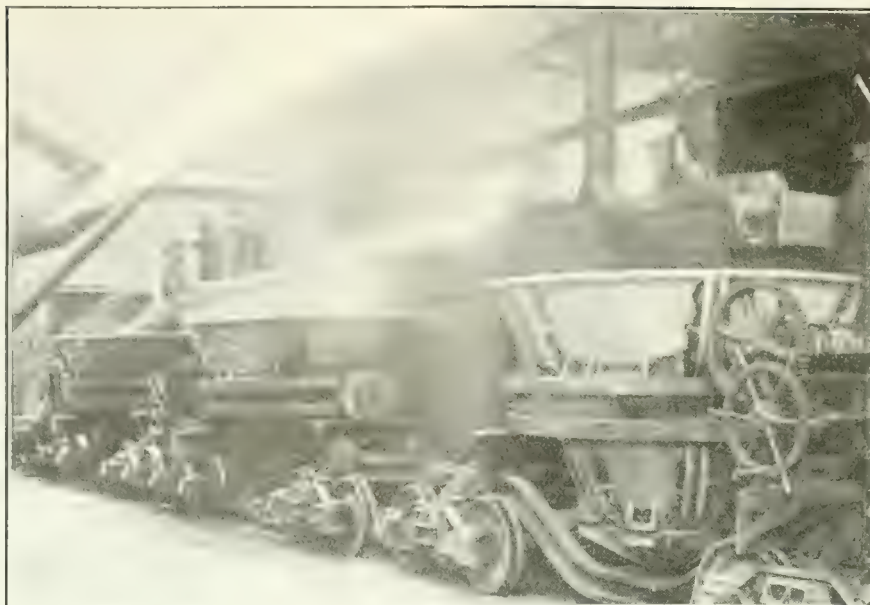
RUNNING SLAG FROM THE BLAST FURNACE INTO LADLE-CARS.
