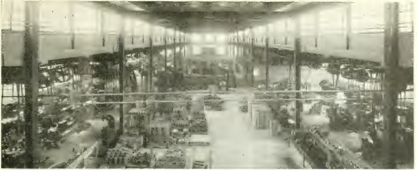
FIG. 1. VIEW OF MAIN BAY SHOWING ASSEMBLY BENCHES AND WORK IN PROGRESS. MACHINE DEPARTMENTS ARE LOCATED IN EACH SIDE BAY.
