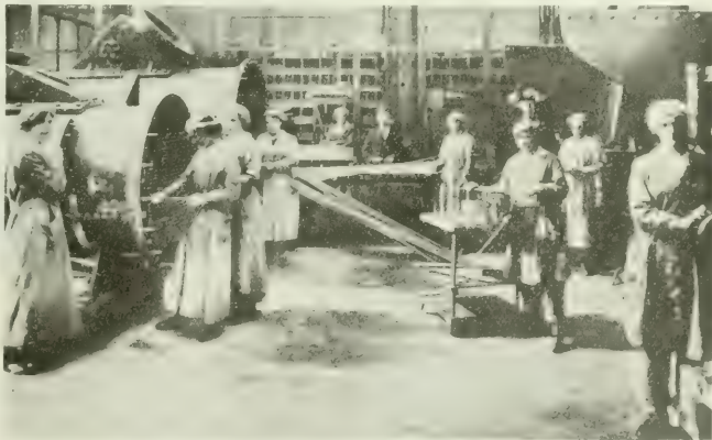
TUBING A MARINE ENGINE CONDENSER.
